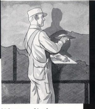
Flax-li-num has long been recognized as the highest type of insulation available . . Diamond mesh metal lath painted with asphaltum after forming, is universally accepted as the ideal plaster base.
