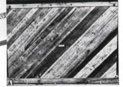
Ordinary stud and plate walls sheathed diago-nally are 4 to 7 times as stiff and 7 to 8 times as strong as if borizontally sheathed.
