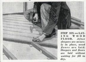
THE Bull Dog Method of anchoring wood floors over concrete eliminates dry rot. This doubles floor life, for, because of dead air space, sleepers do not deteriorate. If desired,
