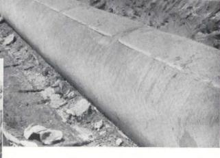
Hydrated lime used as an admixture in 8-mile concrete aqueduct, 5 ft. diameter and 115 ft. head. St. Paul, Minn. Lloyd Thompson, Construction Engineer.
