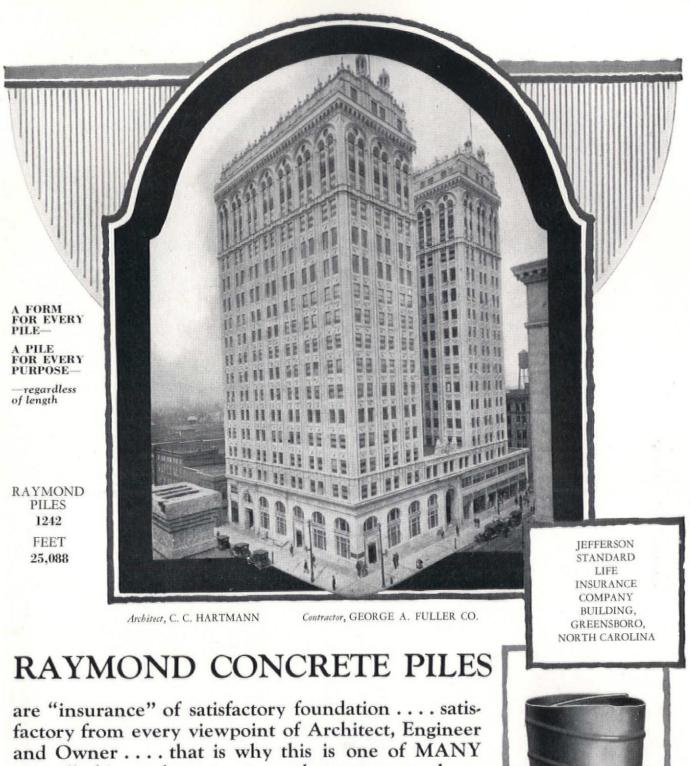
typically big modern structures that rest upon them. Every pile poured into a spirally reinforced steel shell and every shell left in the ground.
