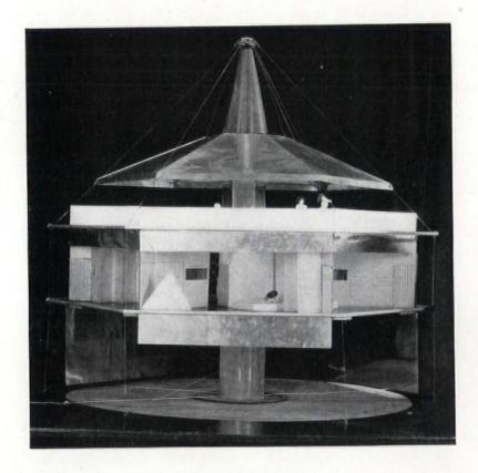
Finished structure showing duralumin awning, central mast with elevator and vertical grouping of conduits for heat, light, air, disposal and water; translucent non-breakable panes inclosing vacuums for outer walls; translucent ceilings; a bedroom indirectly floodlighted with one triangular metallic window shutter partially drawn; parking space under the house; the whole structure suspended from the mast.
