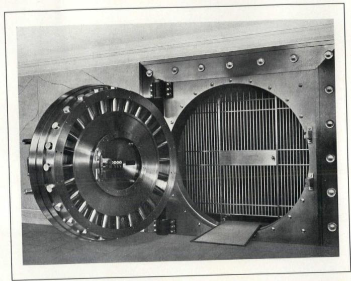
MASTERS at fitting and finishing put the final touch to Diebold Vault Doors . . . and with hand tools. That is why each one has about it a feeling of individualism that can't be produced from the mould of mass production • The Diebold Vault Door shown here weighs fifty tons. Yet it moves on its giant crane-hinge mounting to the touch of the hand. Closed and fully checked it withstands the most determined attack of expert cracksmen.
