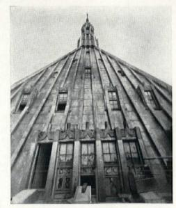
An unusual perspective of the tower showing effect gained by the straight lines. The entire top is encased in Anaconda Copper.
