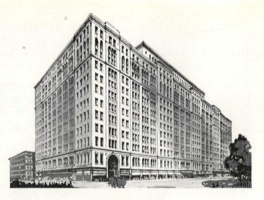
T. Eaton Company, Ltd., Montreal, Quebec. Ross & MacDonald, Architects. Sproatt & Rolph, Consultants. Foundations waterproofed with 12,000 pounds Truscon Waterproofing Paste. Truscon Stone Backing used to dampproof cut stone. Truscon Agatex Crystals used for hardening subbasement floor of new building.
