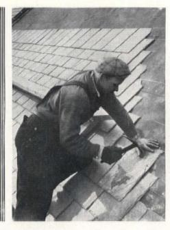
Ebenezer Community Building, Chicago, showing how slate is nailed directly to the roof-deck of Federal Nailing Concrete Slabs. Archt., Andrew E. Norman.
