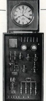
LLUSTRATION shows Type AEG Emergency Lighting System Control Panel, mounted in steel cabinet with Electric Self Winding Clock for supervision and control of charge of storage battery, which is one of the many Landis features
