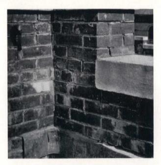
Cracks in Parapet Caused by Improper Mortar and Insecure Bonding of Brick and Mortar
