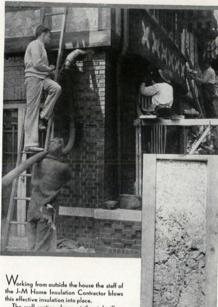
The wall section shown at the right illustrates how closely J-M Home Insulation packs into the walls, filling all the spaces between the studs.
