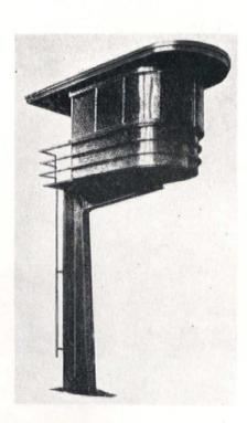
Traffic Tower, Berlin, Mies van der Rohe, Architect. The cantilevered support insures a minimum of obstruction to the street traffic
