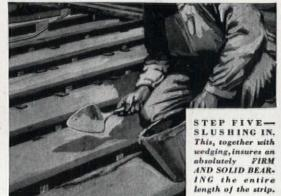
THE Bull Dog Method and process of anchoring wood floors over concrete prevents buckling, squeaking and doming. Once properly wedged and slushed, the sleepers hold the floors rigidly, permanently.
