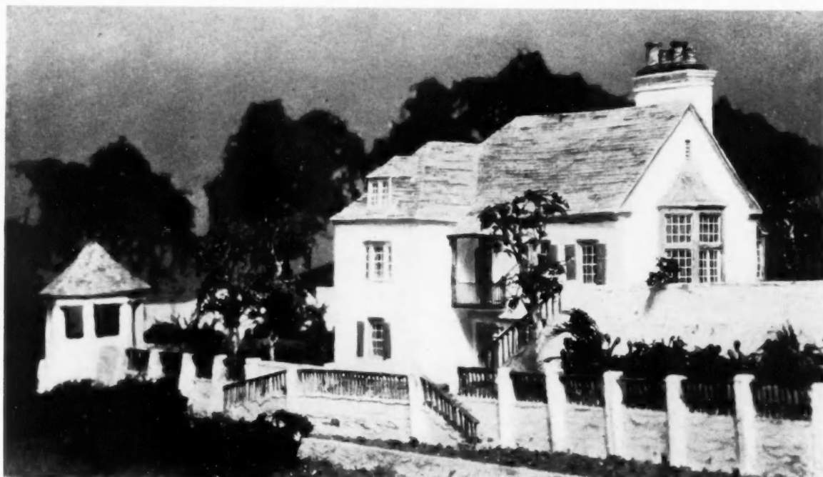
PHOTOGRAPH OF MODEL ESTATE OF C. H. WHITE, BENNINGTON, VERMONT BOGNER AND BILLINGS, ARCHITECTS
