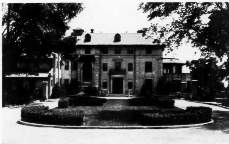
Seventeen telephone outlets provide for complete telephone convenience in the residence and garage of Mr. Edward Schmidt, 16960 East Jefferson Avenue, Detroit. The telephone wiring is carried in conduit built into the walls and floors. RAYMOND CAREY, Architect, Detroit, Michigan.
