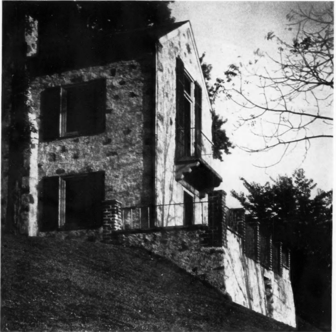
HOUSE FOR MRS. SAMUEL A. KING, BRYN MAWR, PENNSYLVANIA MELLOR AND MEIGS, ARCHITECTS
