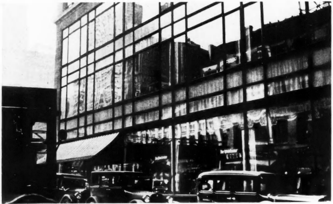
CURTAIN WALL OF GLASS BUCKLEY-NEWHALL BUILDING, 1071 SIXTH AVENUE, NEW YORK CITY JOHN B. SNOOK SONS, ARCHITECTS
