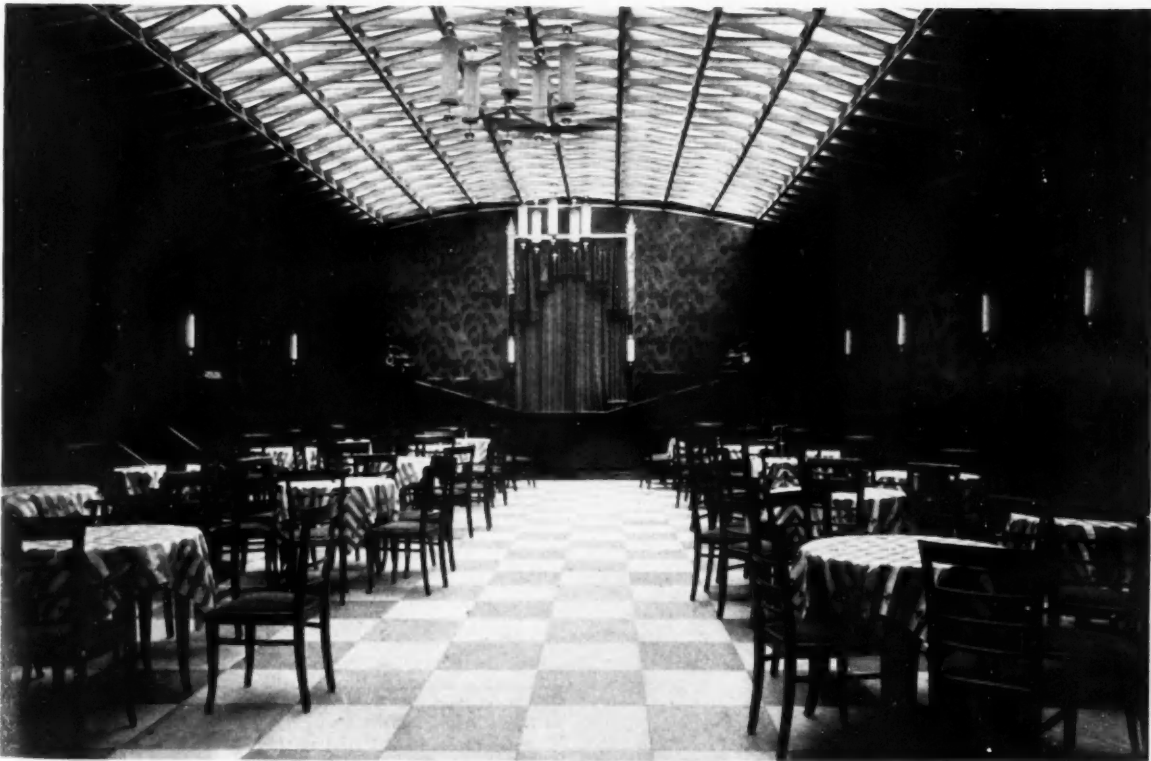
INTERIOR SHOWING STEEL VAULT CONSTRUCTION RESTAURANT, DESSAU, GERMANY PAULSEN, ARCHITECT
