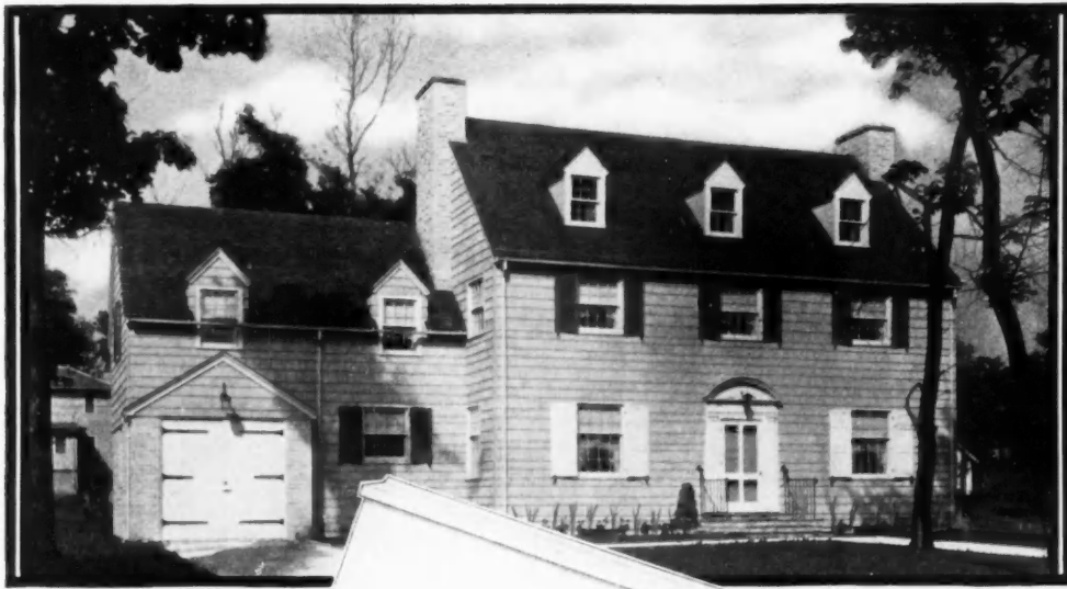
Home of F. W. Luchring, Minneapolis Architect, Roy Childs Jones— Tyrie & Chapman, Associates
