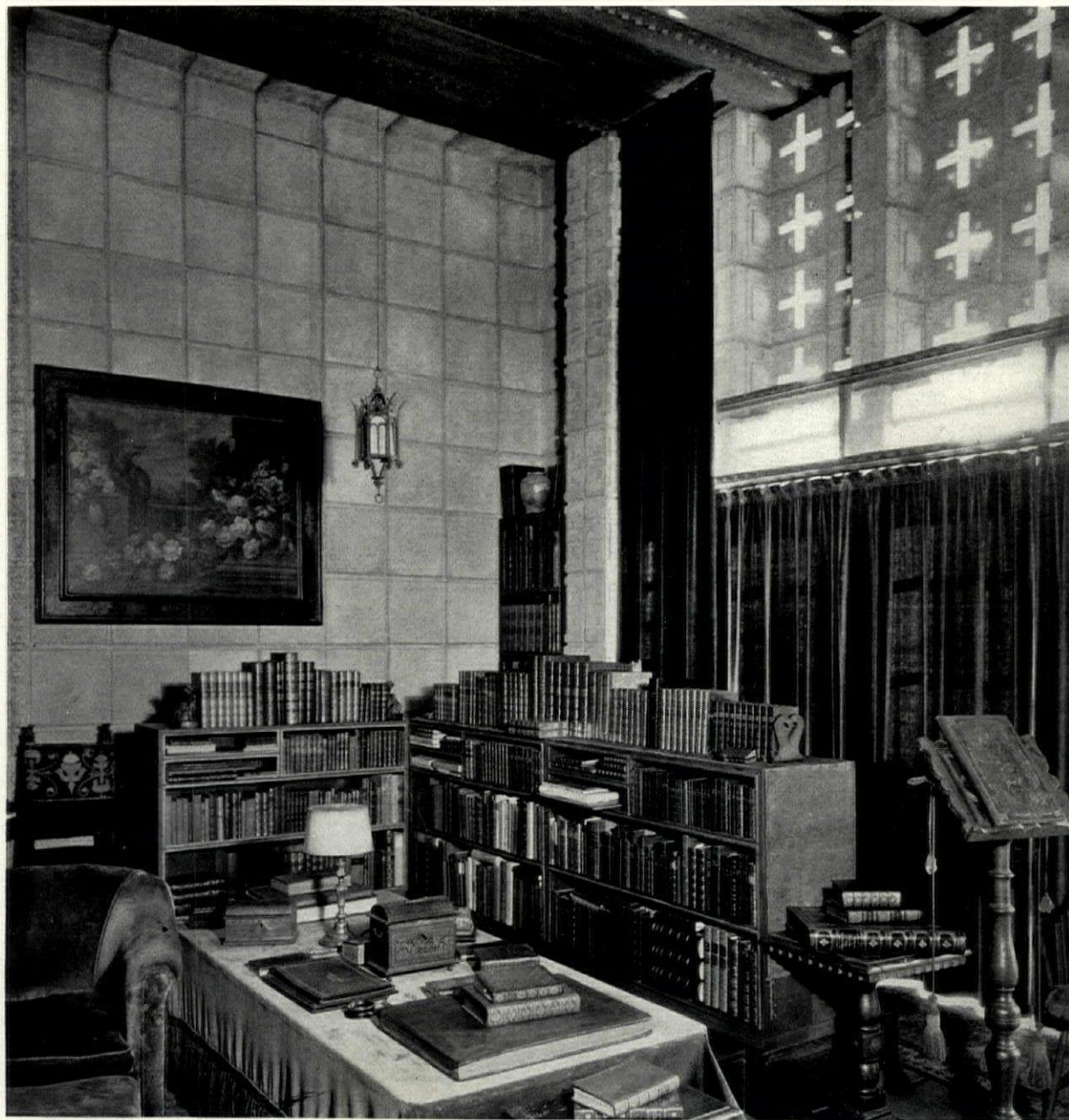
USE OF PLAIN AND PATTERNED BLOCKS FOR INTERIOR WALLS LA MINIATURA, PASADENA, CALIFORNIA FRANK LLOYD WRIGHT, ARCHITECT
