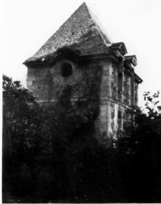
CORNER PAVILION OF THE CITY WALLS, RICHELIEU
