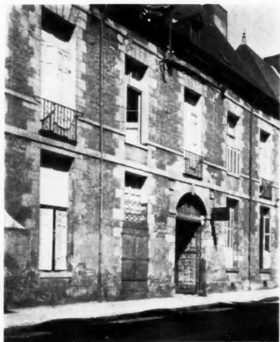
TYPICAL HOTEL ON THE GRANDE RUE
