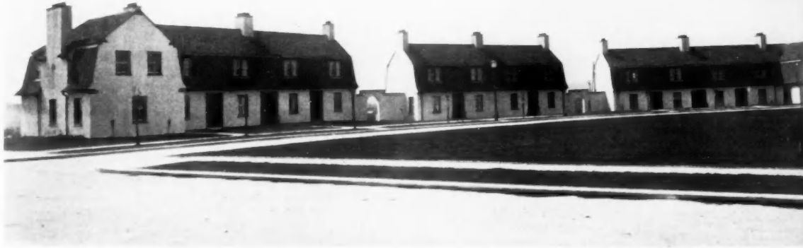
A GROUP OF GRADE II HOUSES (MANSARD TYPE), KEMSLEY VILLAGE
