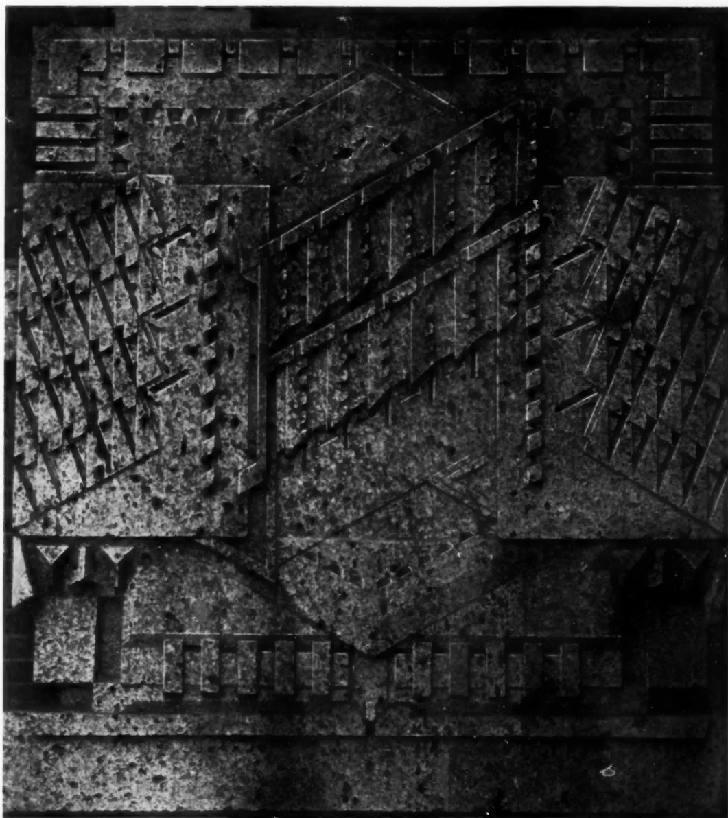
LAVA-CUTTING TEN FEET SQUARE, SHOWING TEXTURE OF MATERIAL MODIFYING THE SEVERE CARVING THE IMPERIAL HOTEL, TOKIO FRANK LLOYD WRIGHT, ARCHITECT
