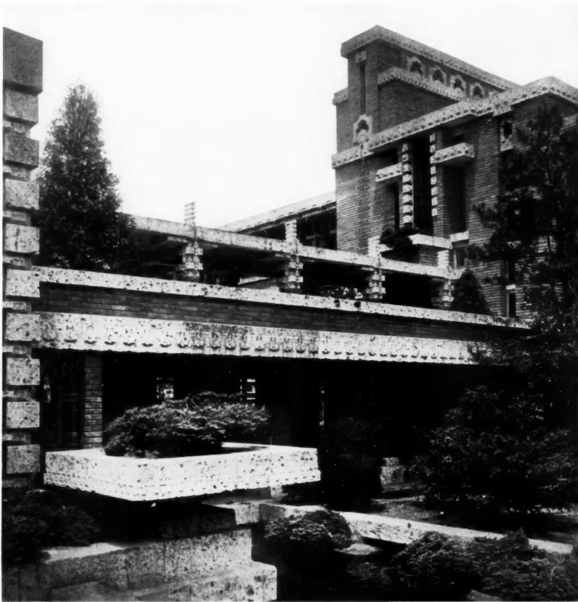
CANTILEVER SLAB WITH CUT-LAVA EDGES OVER PASSAGE BETWEEN LOBBY AND GUEST WINGS
