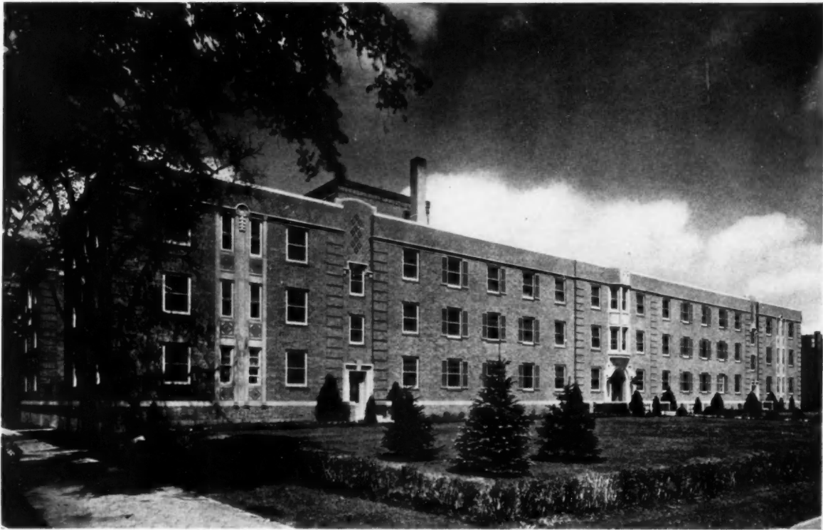
GENERAL VIEW OF EXTERIOR
