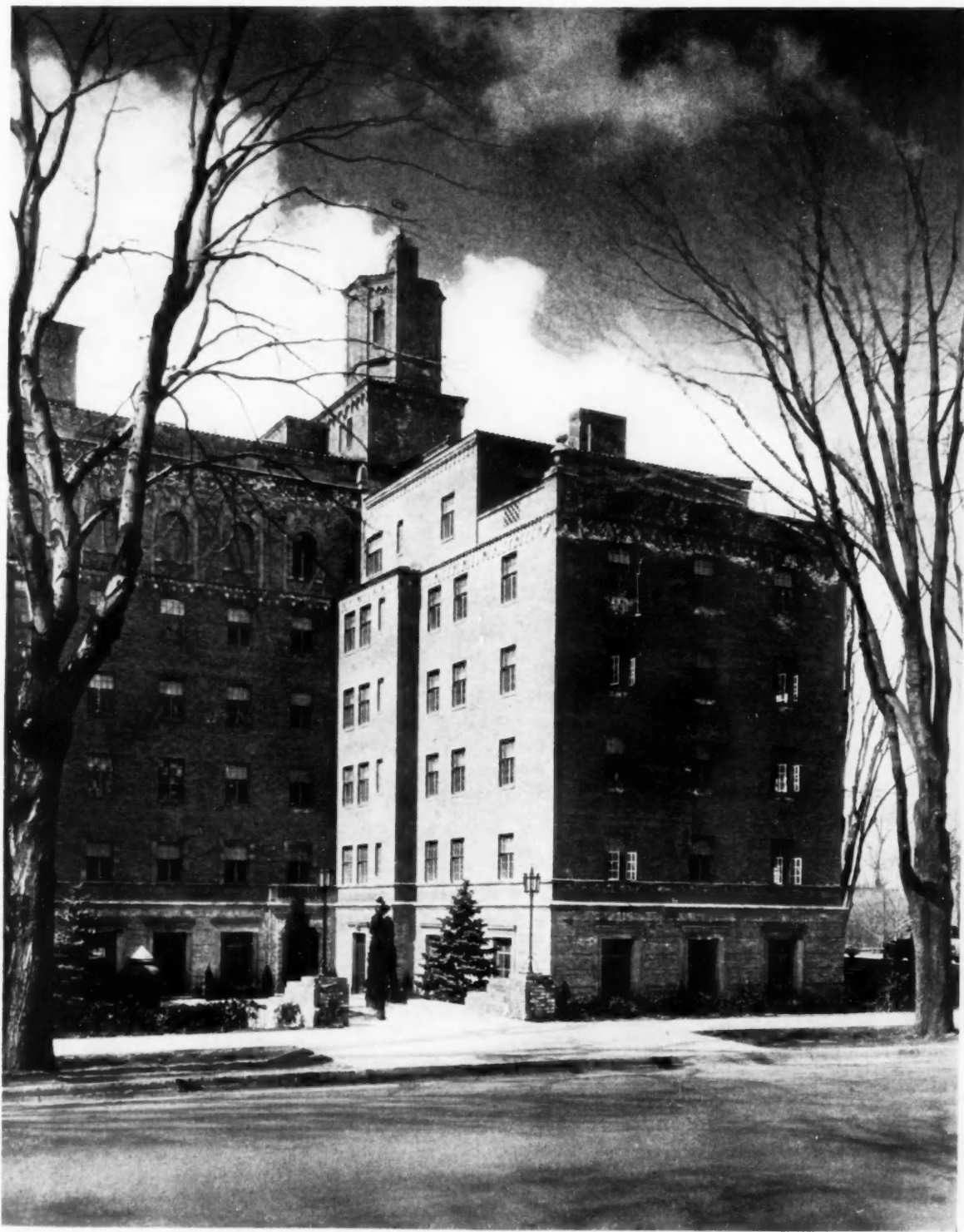
KENWOOD APARTMENTS, GREAT NECK, L. I. LE ROY P. WARD, ARCHITECT; HARRY J. KERRIGAN, ASSOCIATE
