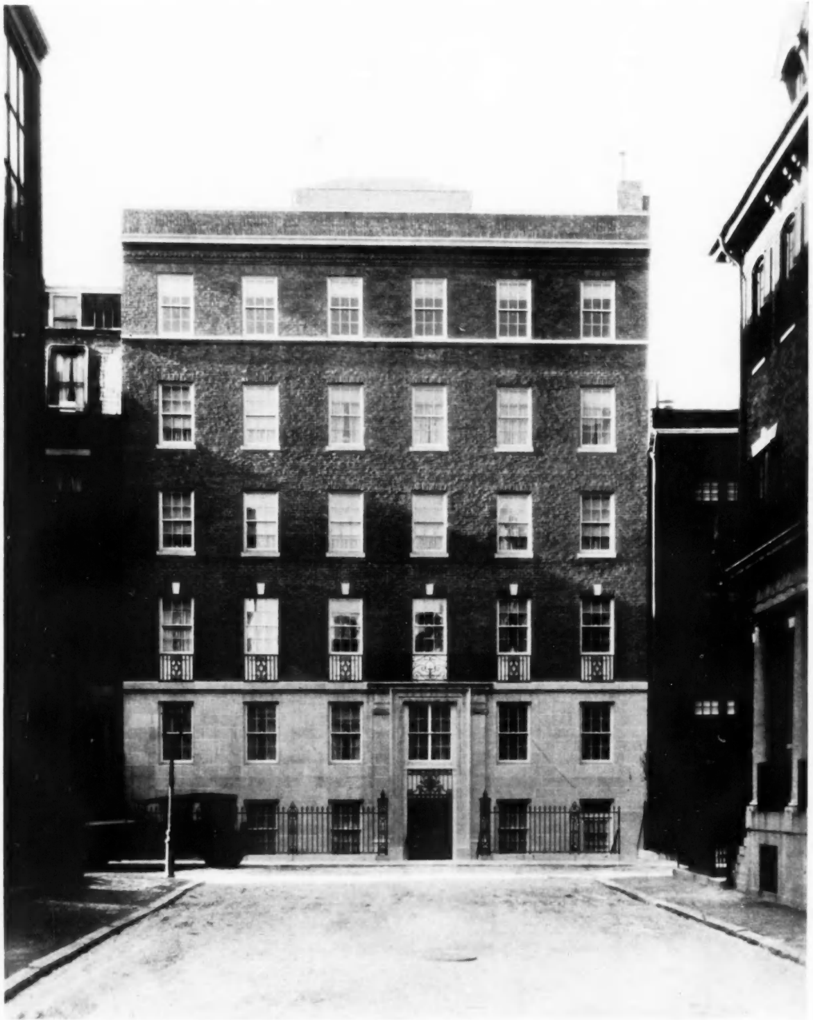
APARTMENT HOUSE AT 10 OTIS PLACE, BOSTON, MASS. BIGELOW & WADSWORTH, ARCHITECTS
