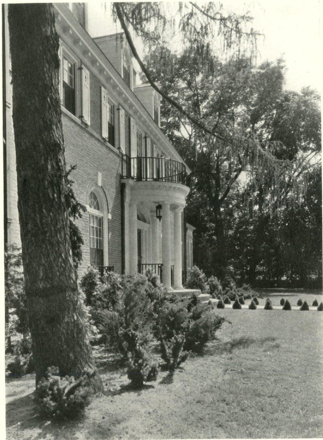
RESIDENCE OF J. P. MANNING, ESQ., BOSTON, MASS. McLaughlin & Burr, Architects
