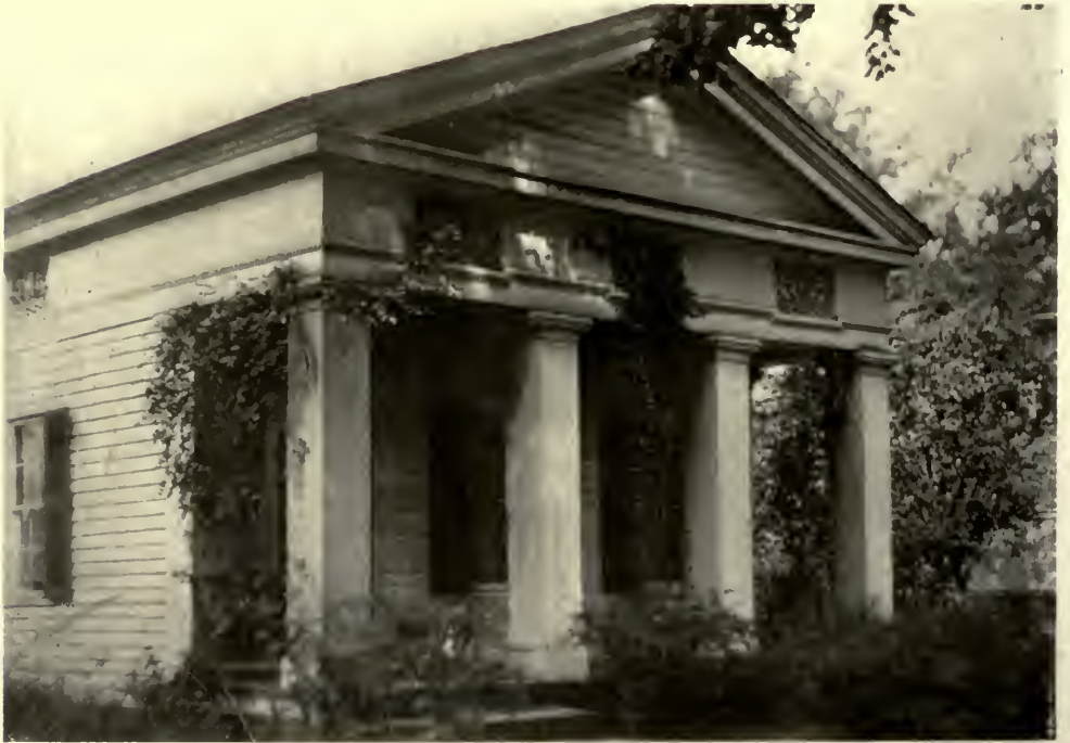
THE BENNETT (KEMPF) HOUSE, ANN ARBOR. THE TEMPLE IN VERNACULAR. THE ANTA CAPITALS ARE PROFILED ENTIRELY WITH PLAIN CHAMFERS AND FILLETS.
