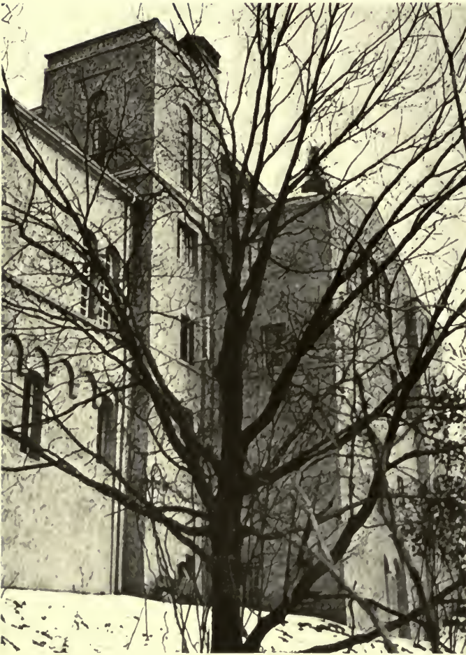
DETAIL OF SMALL TOWER.
