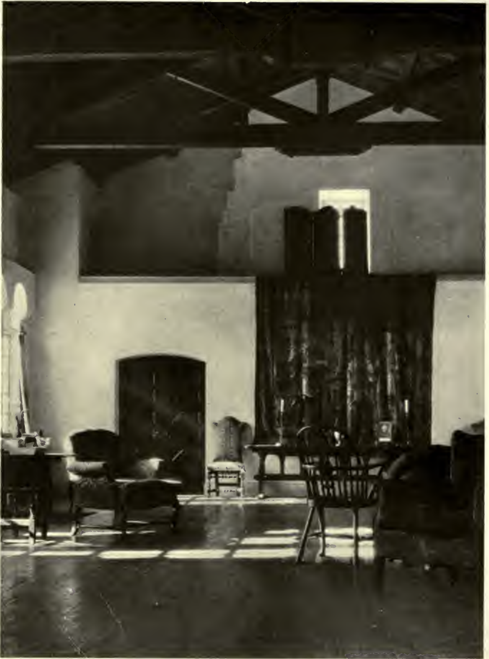
LIVING ROOM, SHOWING GALLERY AND DOOR LEADING INTO GLASSERY— PHI DELTA THETA FRATERNITY HOUSE, CORNELL UNIVERSITY, ITHACA, N. Y. WILLIAM McLEISH DUNBAR, ARCHITECT.
