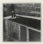
Spraying roof deck of box car with Carbosota Creosote Oil (no paint used).
