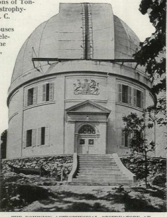
THE DOMINION ASTROPHYSICAL OBSERVATORY AT VICTORIA, B. C., IS CIRCULAR, 66 FEET IN DIAMETER, AND SURMOUNTED BY A REVOLVING DOME WHICH IS COVERED WITH TONCAN METALA
