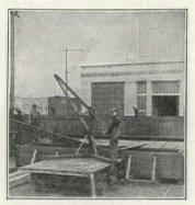
The Open-Tank Process: Simple wooden tank (lined with sheet iron), equipped with steam colls and small derrick.
