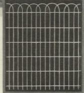
The above illustration shows Style No. 6, 42" high, wires No. 9 strand, No. 8 wicket. The mesh is 2x6, too small to allow children to climb upon the fence. This is the strongest and most durable of all Excelsior Fences, and we recommend it for use wherever highest quality and long service are desired.
