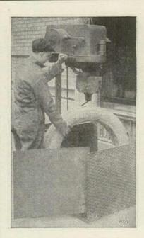
Model E-Electric. That part of Hoist and G & G Spring Guard Gates shown telescope below grade, and the G & G Sidewalk Doors lie flush with grade when Hoist is not in operation.
