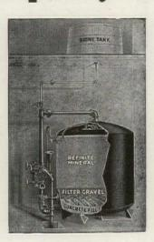
Sectional View of Refinite Water Softener
