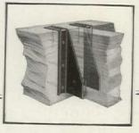
VAN DORN Patented Steel Joist Hanger.
