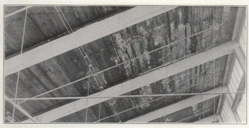
Roof planks of weave shed of textile mile destroyed by decay in nine years. (Courtesy F. J. Hoxie, Engr., Associated Factory Mutual Fire Ins. Cos., Boston)
