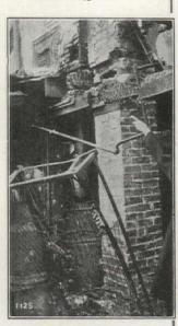
Chimney without Flue Lining. See where the brick dropped out and the fire started.
