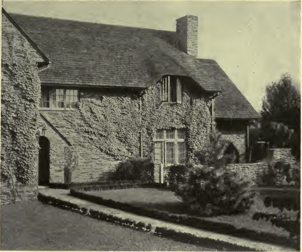
FORECOURT—HOUSE OF LEONARD T. BEALE, ESQ., ST. DAVIDS, PA. Mellor & Meigs, Architects.
