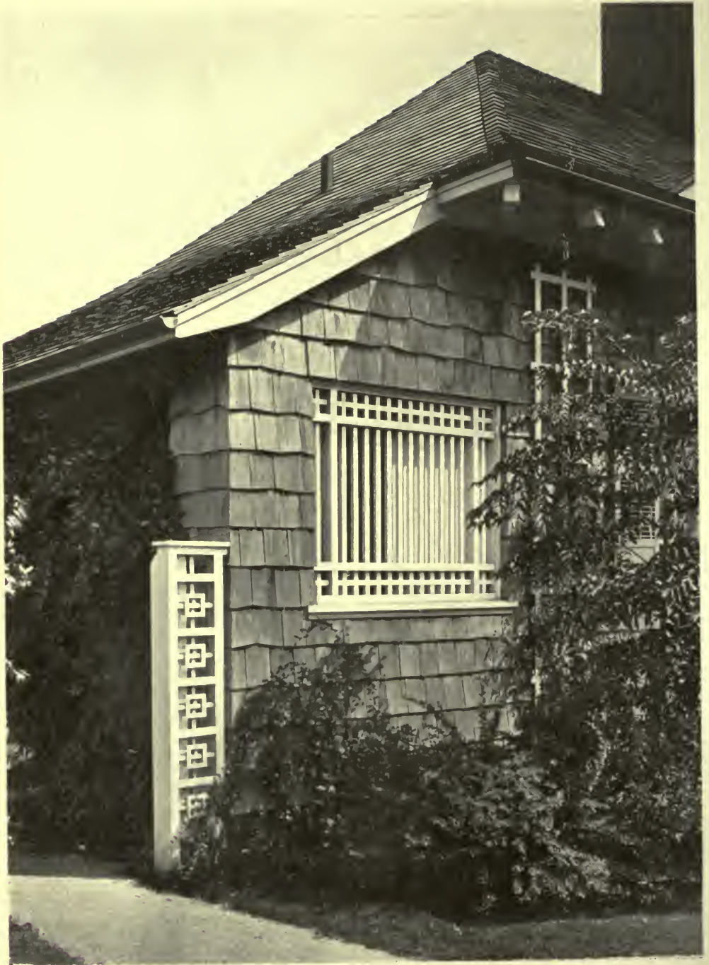
DETAIL OF SERVICE WING—COUNTRY HOUSE AT SOUTHAMPTON, L. I. GOODHUE LIVINGSTON, ESQ., OWNER AND ARCHITECT.
