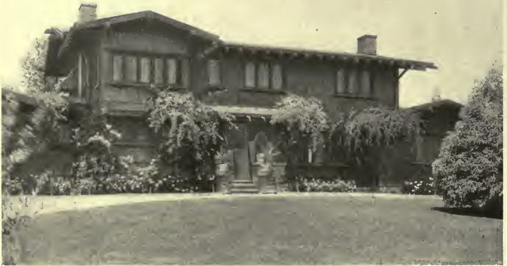
RESIDENCE OF WILLIAM A. CHILDS, ESQ., RIVERSIDE, CAL. George A. Clark, Architect.
