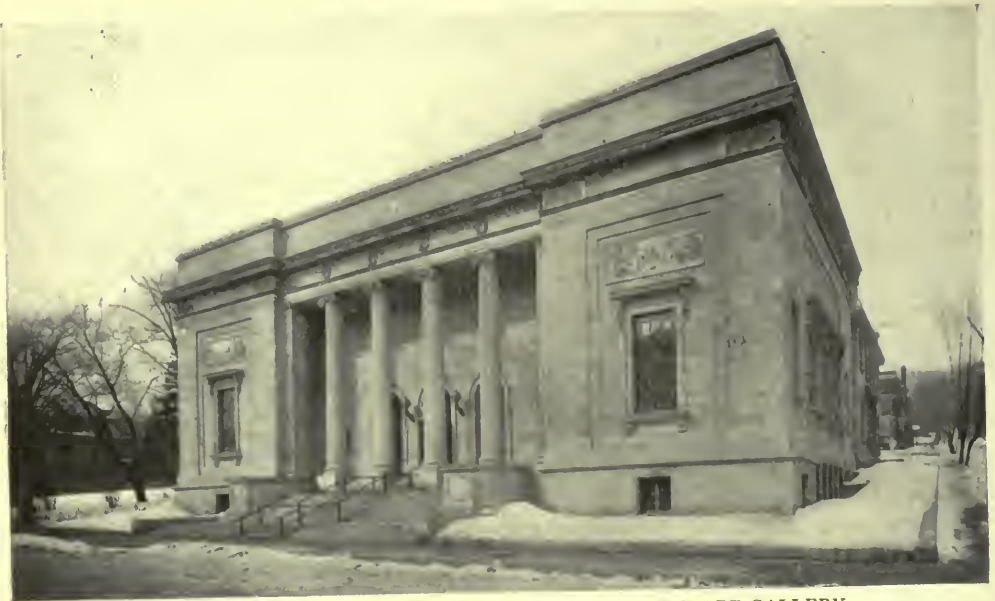
MAIN FACADE ON SHERBROOKE STREET—MONTREAL ART GALLERY. E. and W. S. Maxwell, Architects.
