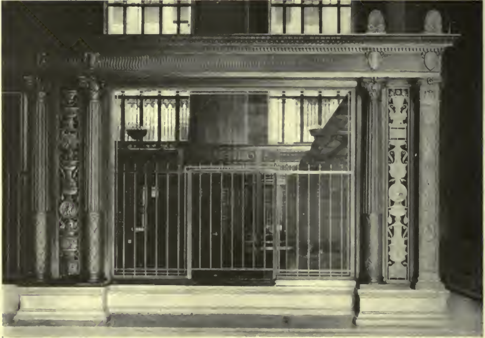
DETAIL OF BRONZE SCREEN—BANKING ROOM, GUARANTY TRUST CO., NEW YORK CITY. York & Sawyer, Architects.
