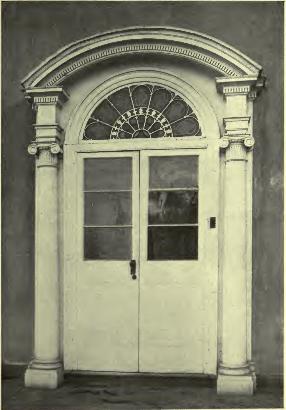
NORTH DOOR—THE WOODLANDS, PHILADELPHIA. BUILT ABOUT 1770. AN EXAMPLE OF THE "THIRD TYPE" OF GEORGIAN.
