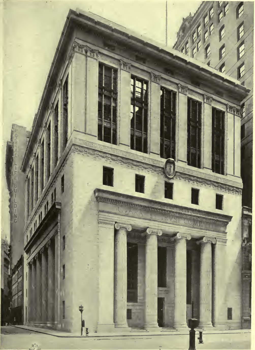
BANKING HOUSE OF THE GUARANTY TRUST COMPANY, NEW YORK CITY. YORK & SAWYER, ARCHITECTS.
