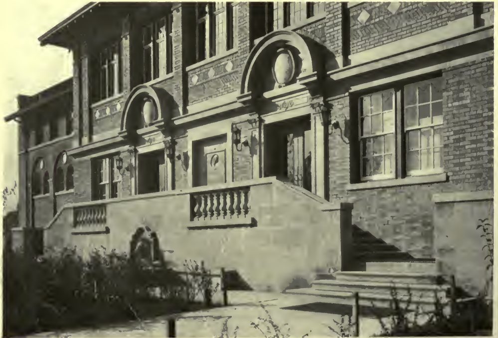
ALLEN STREET ENTRANCE—JOHN C. PROCTOR RECREATION CENTER, PEORIA, ILL. Hewitt & Emerson, Architects.
