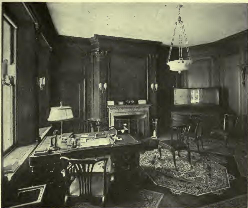
MR. MORGAN'S PRIVATE OFFICE—BANKING HOUSE OF J. P. MORGAN & CO. Trowbridge & Livingston, Architects.
