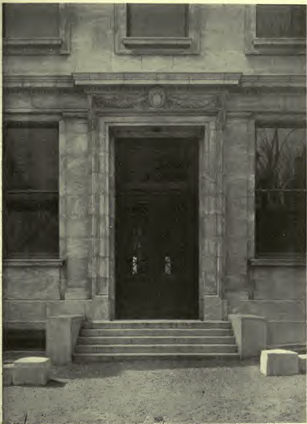
DETAIL OF ENTRANCE ON ONTARIO AVENUE—MONTREAL ART GALLERY. E. AND W. S. MAXWELL, ARCHITECTS.
