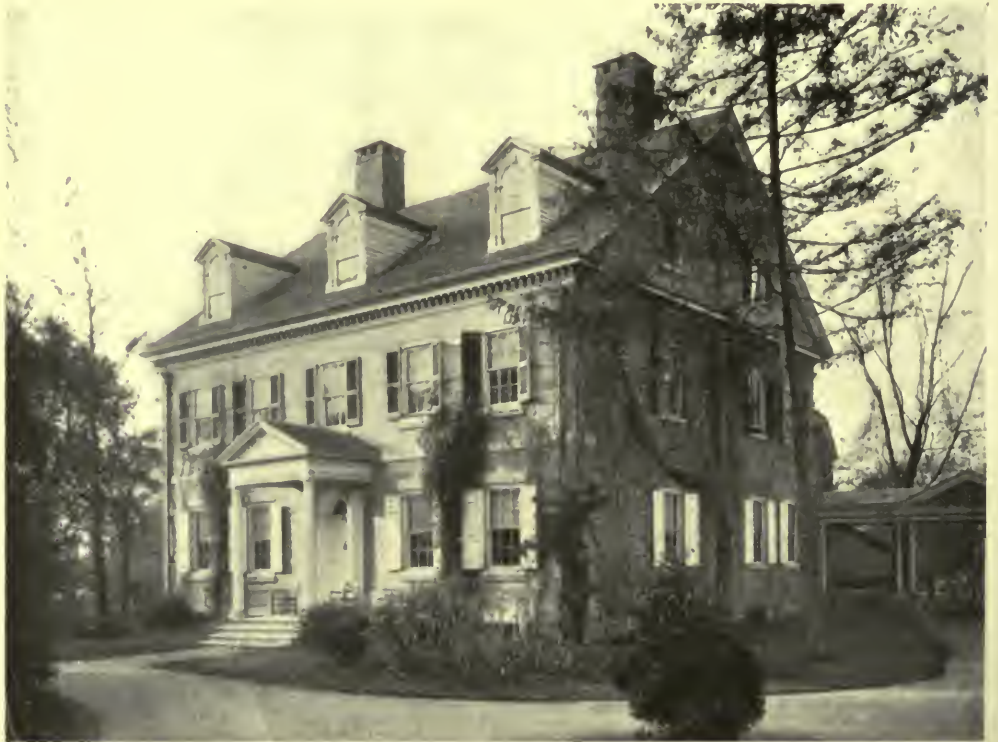
EAST FRONT—UPSALA, GERMANTOWN, PHILADELPHIA. An Example of the "Third Type" of Georgian.
