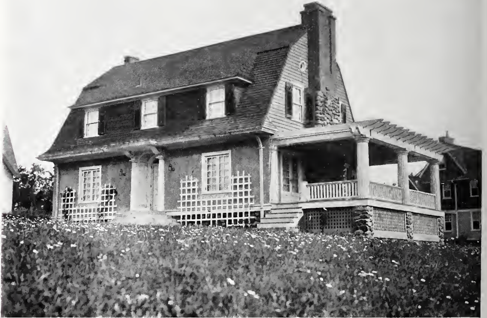
RESIDENCE OF JOHN P. ALLEN, ESQ., SCARSDALE, N. Y. John C. Moore, Architect.
