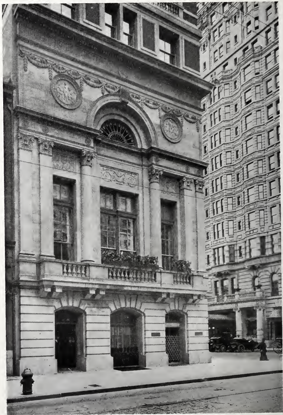
DETAIL ON WALNUT STREET, THE RITZ-CARLTON HOTEL, PHILADELPHIA, PA. HORACE TRUMBAUER AND WARREN & WETMORE, ASSOCIATED ARCHITECTS.
