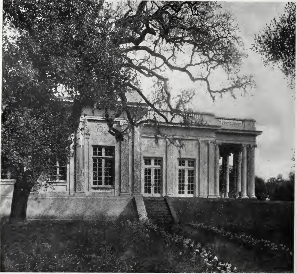
THE McNEAR RESIDENCE, MENLO PARK, CAL. Bliss and Faville, Architects.
