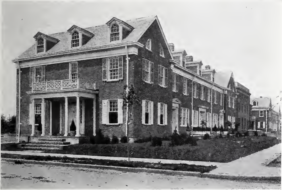
HOUSES AT JAMAICA, L. I.—ONE GROUP OF FIVE HOUSES. Electus D. Litchfield, Architect.
