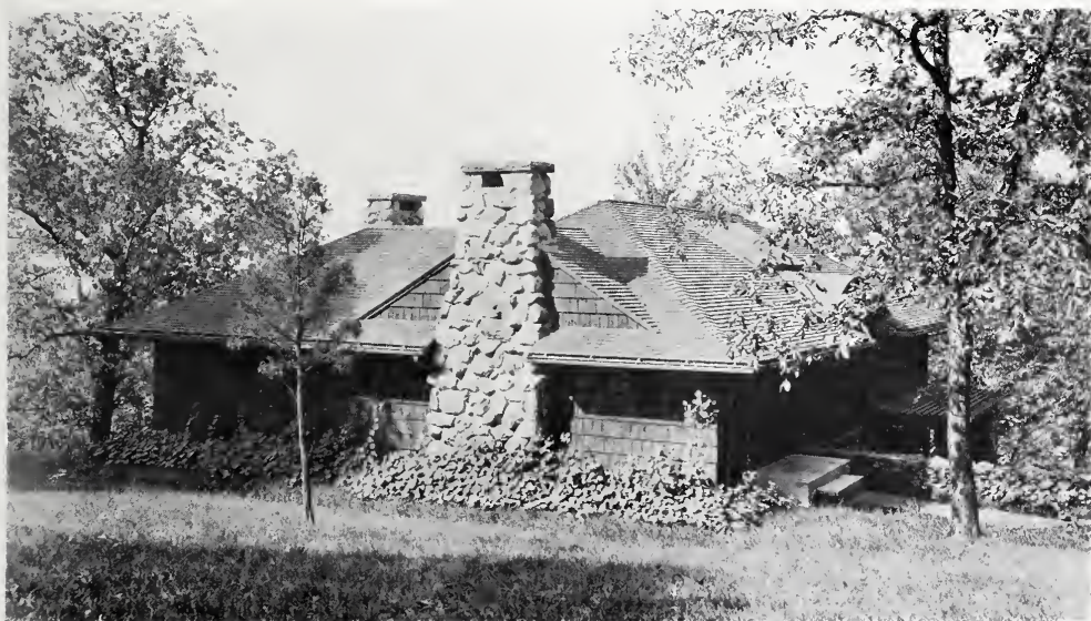
FROM THE UP-HILL SIDE—STUDIO IN WESTCHESTER COUNTY, N. Y. Arthur T. Remick, Architect.
