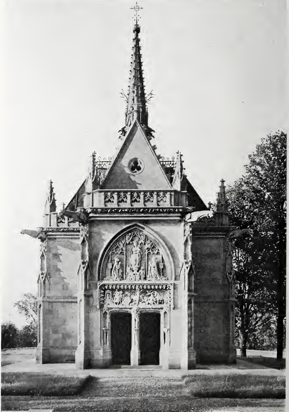
FRONT ELEVATION—MAUSOLEUM OF O. H. P. BELMONT, ESQ., WOODLAWN, N. Y. HUNT & HUNT, ARCHITECTS.
