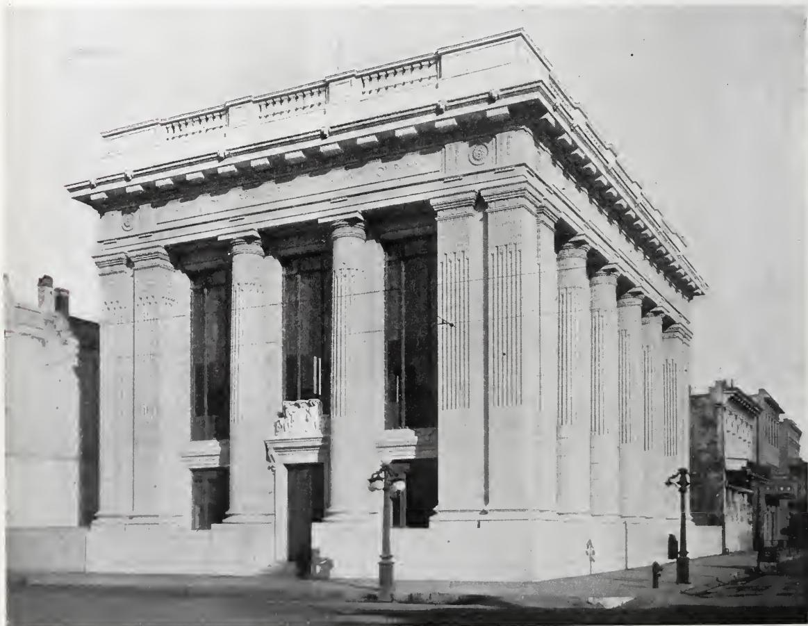
THE NATIONAL BANK OF D. O. MILLS & CO., SACRAMENTO, CAL. Willis Polk & Co., Architects.
