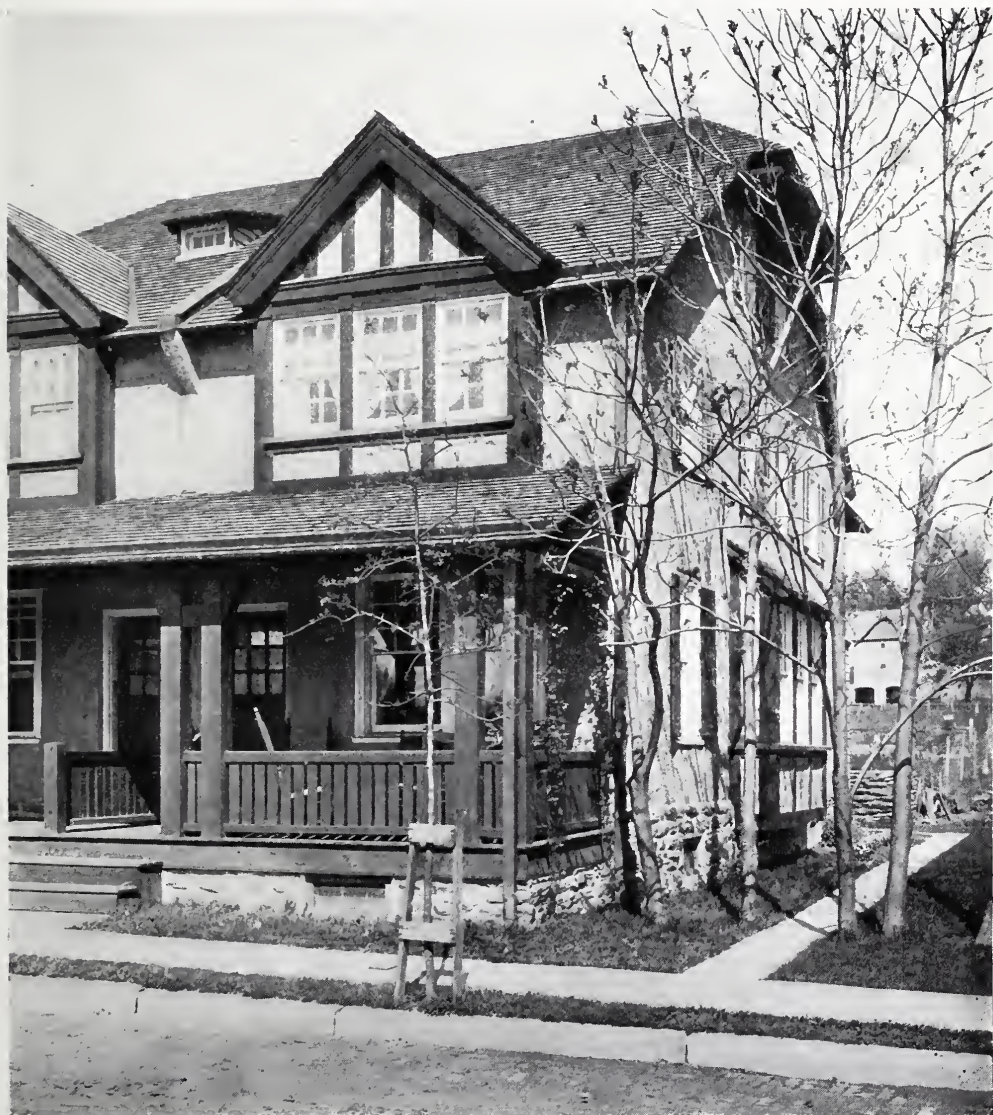
PORCH DETAIL—DOUBLE HOUSE ON BENEZET ST., CHESTNUT HILL, PA. Duhring, Okie & Ziegler, Architects.
