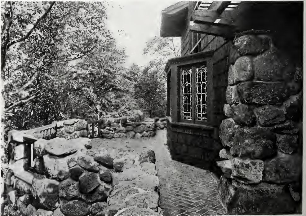
DETAIL OF THE TERRACE—STUDIO IN WESTCHESTER COUNTY, N. Y. Arthur T. Remick, Architect.
