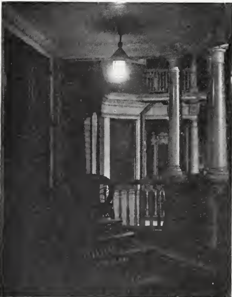
Fig. 9. Typical veranda lighting with 40-watt lamp within opal cylinder.
