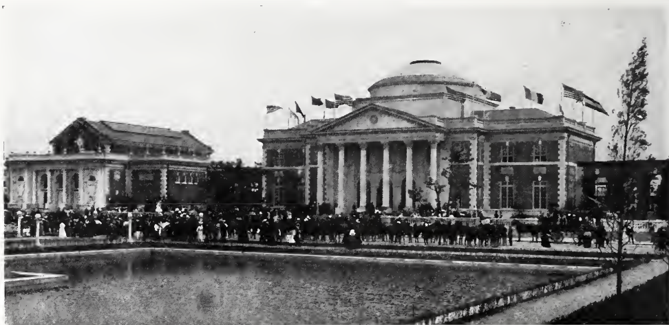
EXPOSITION BUILDINGS, JAMESTOWN, VA., 1907. Parker, Thomas & Rice, Architects.
