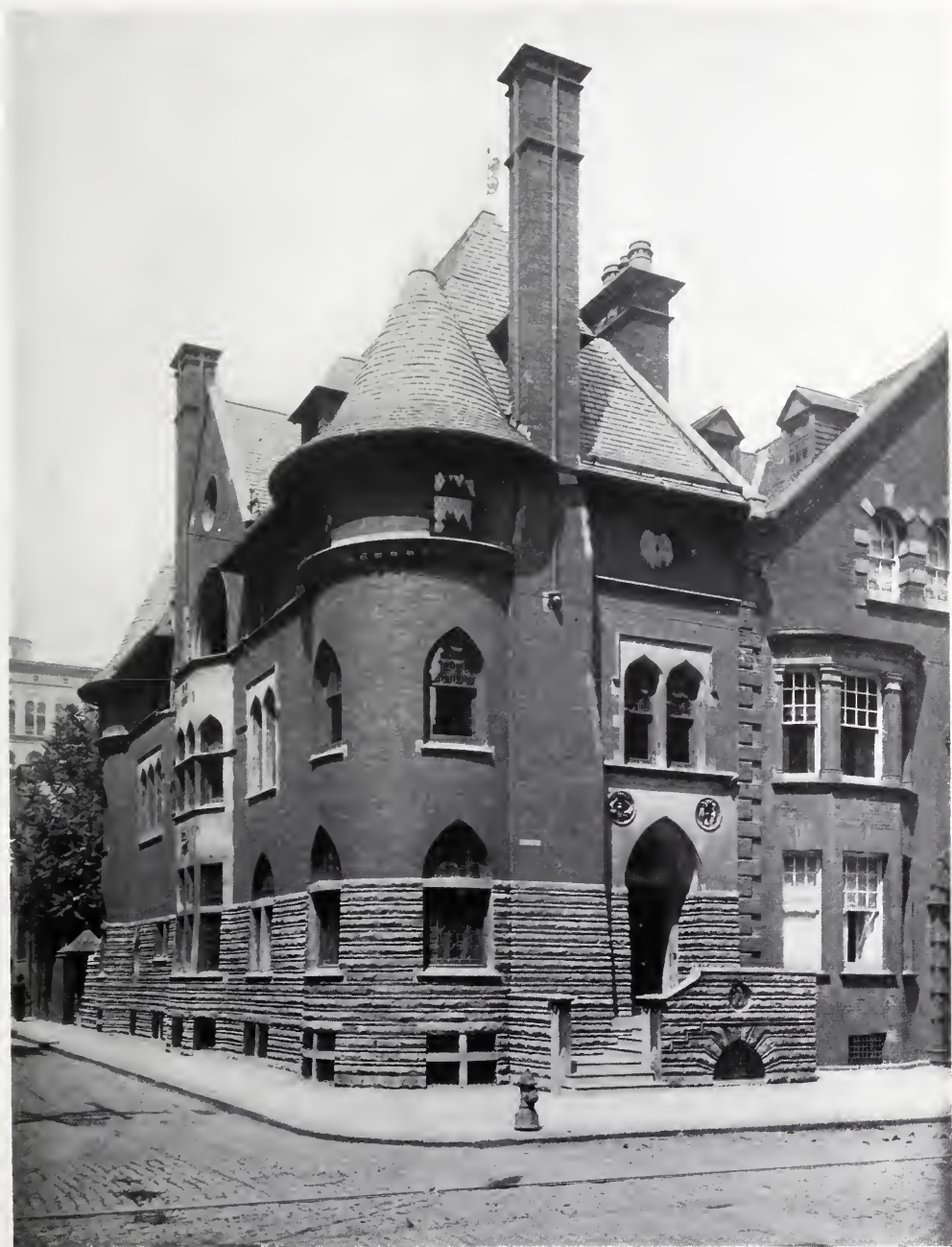
A RESIDENCE AT THE CORNER OF LOCUST AND JUNIPER STREETS, PHILADELPHIA, PA. WILSON EYRE, ARCHITECT.
