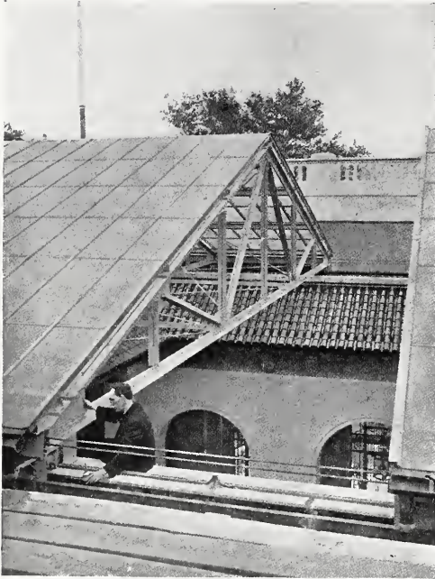
THE SLIDING ROOF OVER THE PATIO.
