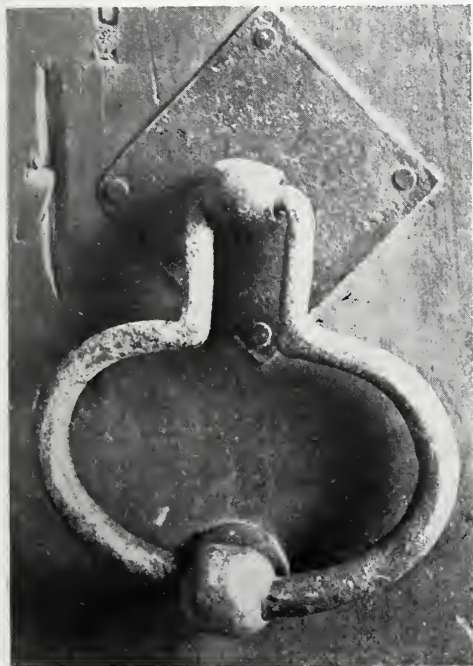
TWO EXAMPLES OF EARLY DUTCH DOOR KNOCKERS OF HAND WROUGHT IRON.
