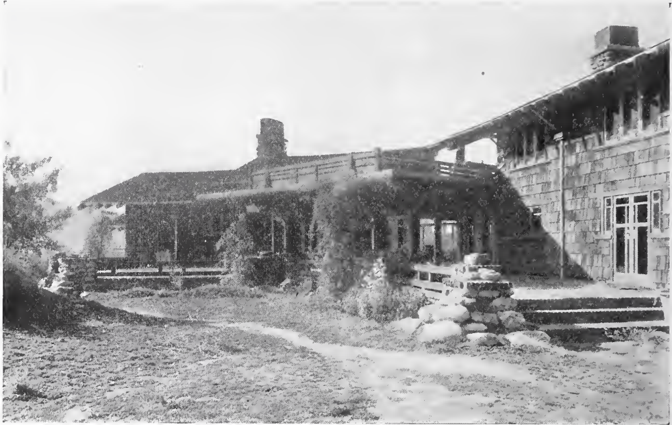
THE PRATT RESIDENCE, NORDHOFF, CAL. Greene and Greene, Architects.
