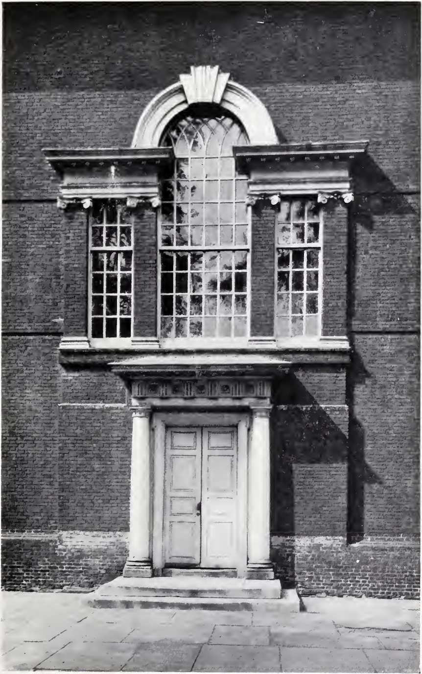
THE PALLADIAN WINDOW OVER THE SOUTH ENTRANCE OF THE STATE HOUSE ("INDEPENDENCE HALL").
