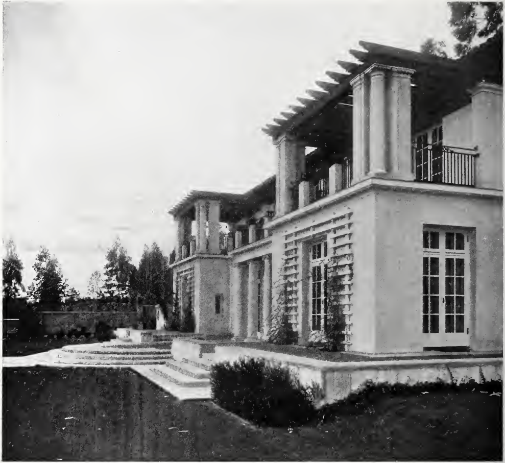
DETAIL. RESIDENCE IN SIERRA MADRE, CAL. Robert David Farquahar, Architect.
