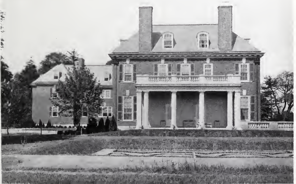
END ELEVATION, RESIDENCE OF MRS. L. Z. LEITER, BEVERLY FARMS, MASS. Parker, Thomas & Rice, Architects.
