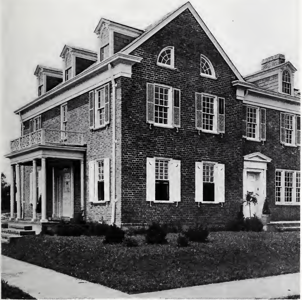
DETAIL OF END HOUSE—HOUSES AT JAMAICA, L. I. Electus D. Litchfield, Architect.
