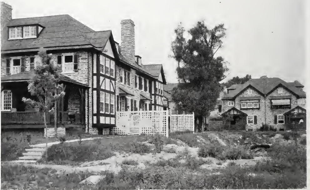
A DETAIL AND PERSPECTIVE VIEW OF THE QUADRUPLE HOUSES. Duhring, Okie and Ziegler, Architects.
