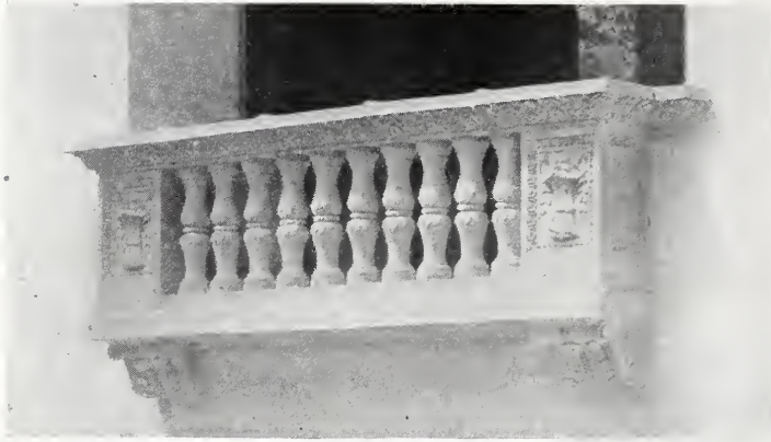
DETAIL OF BALCONY IN THE PATIO—THE PAN-AMERICAN BUILDING, WASHINGTON, D. C.
