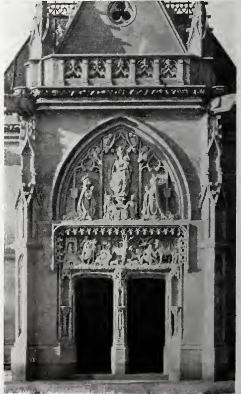
ENTRANCE DETAIL—MAUSOLEUM OF O. H. P. BELMONT, ESQ., WOODLAWN, N. Y. Hunt & Hunt, Architects.
