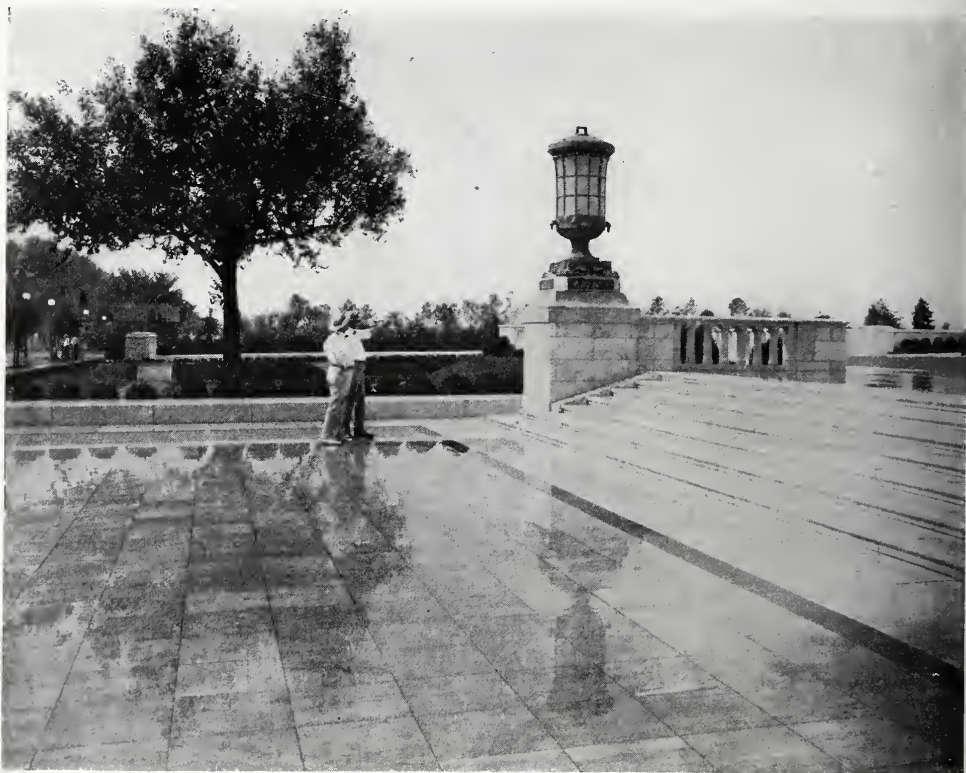
ENTRANCE STEPS. TERRACE AND ONE OF THE GREAT BRONZE LANTERNS, THE PAN-AMERICAN BUILDING, WASHINGTON, D. C. Albert Kelsey and Paul P. Cret, Associate Architects.
