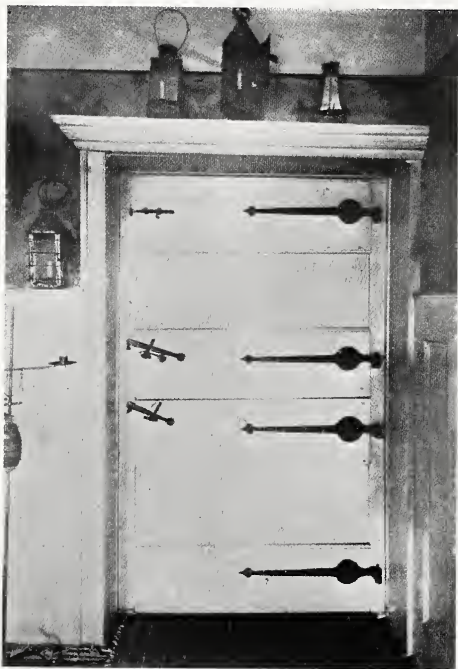
AN OLD DUTCH DOOR, SHOWING HINGES, LATCHES AND BOLT.
