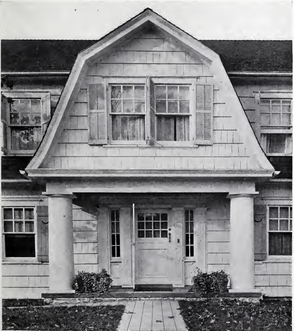
ENTRANCE DETAIL, RESIDENCE OF A. D. HUNTINGTON, ESQ. SUTTON MANOR, N. Y. CHESTER A. PATTERSON, ARCHITECT.
