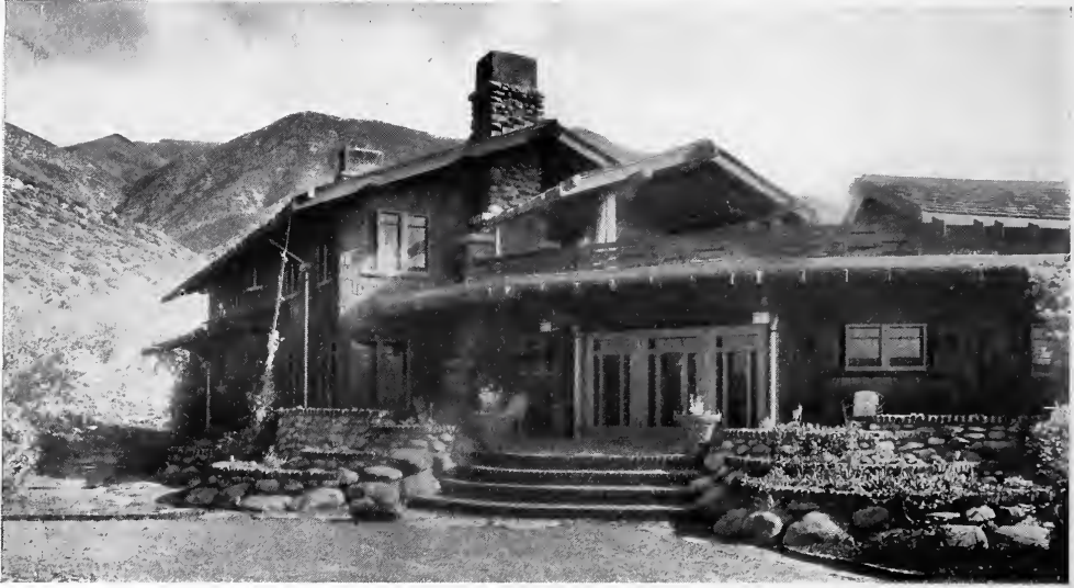
THE PRATT RESIDENCE, NORDHOFF, CAL. Greene and Greene, Architects.
