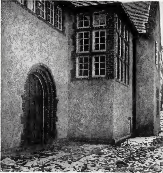
ENTRANCE DETAIL, HOUSE AT CHESTNUT HILL, PA. Edmund B. Gilchrist, Architect.
