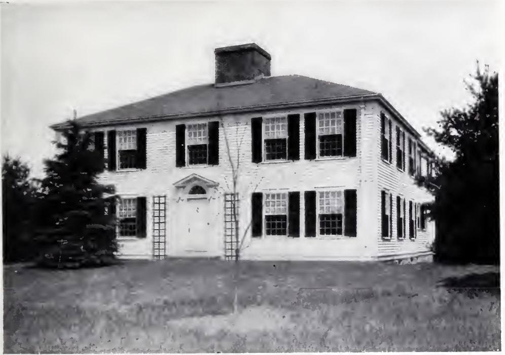
COTTAGE ON THE ESTATE OF WALTER C. BAYLIES, ESQ., TAUNTON, MASS. Parker, Thomas & Rice, Architects.
