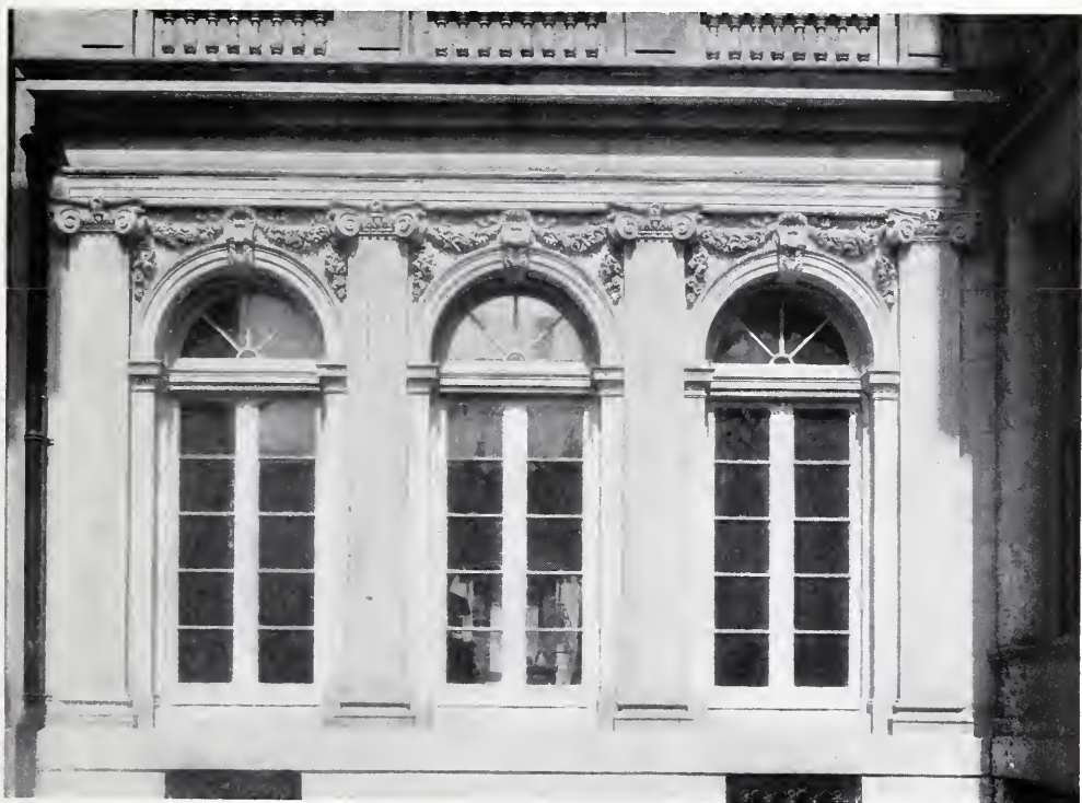
DETAIL, RESIDENCE OF WALTER C. BAYLIES, ESQ., BOSTON, MASS. Parker, Thomas & Rice, Architects.
