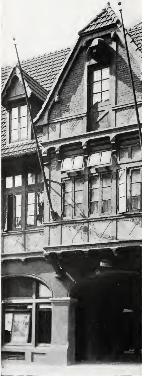
DETAIL OF THE NORTH GERMAN LLOYD STEAMSHIP OFFICES, BALTIMORE, MD. Parker, Thomas & Rice, Architects.
