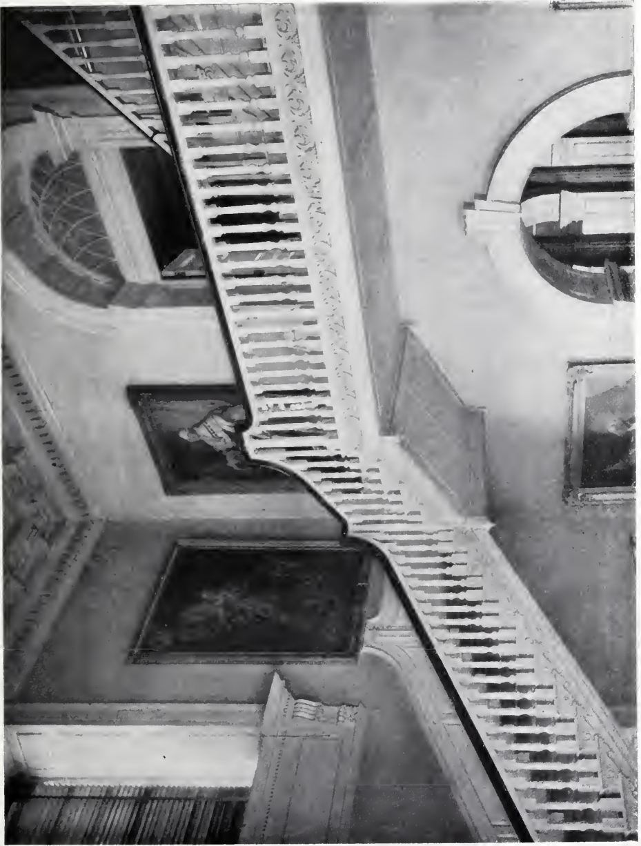
UPPER STAIRWAY IN TOWER OF INDEPENDENCE HALL, PHILADELPHIA, PA.
