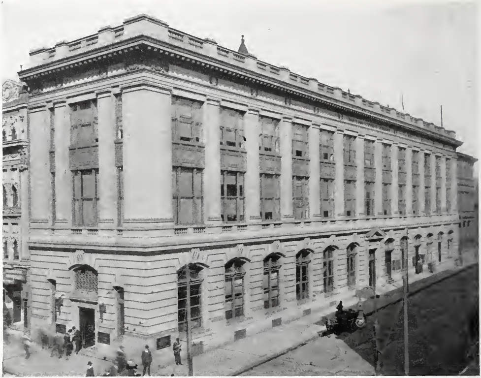
THE MARYLAND CASUALTY COMPANY BUILDING, BALTIMORE, MD. Parker, Thomas & Rice, Architects.
