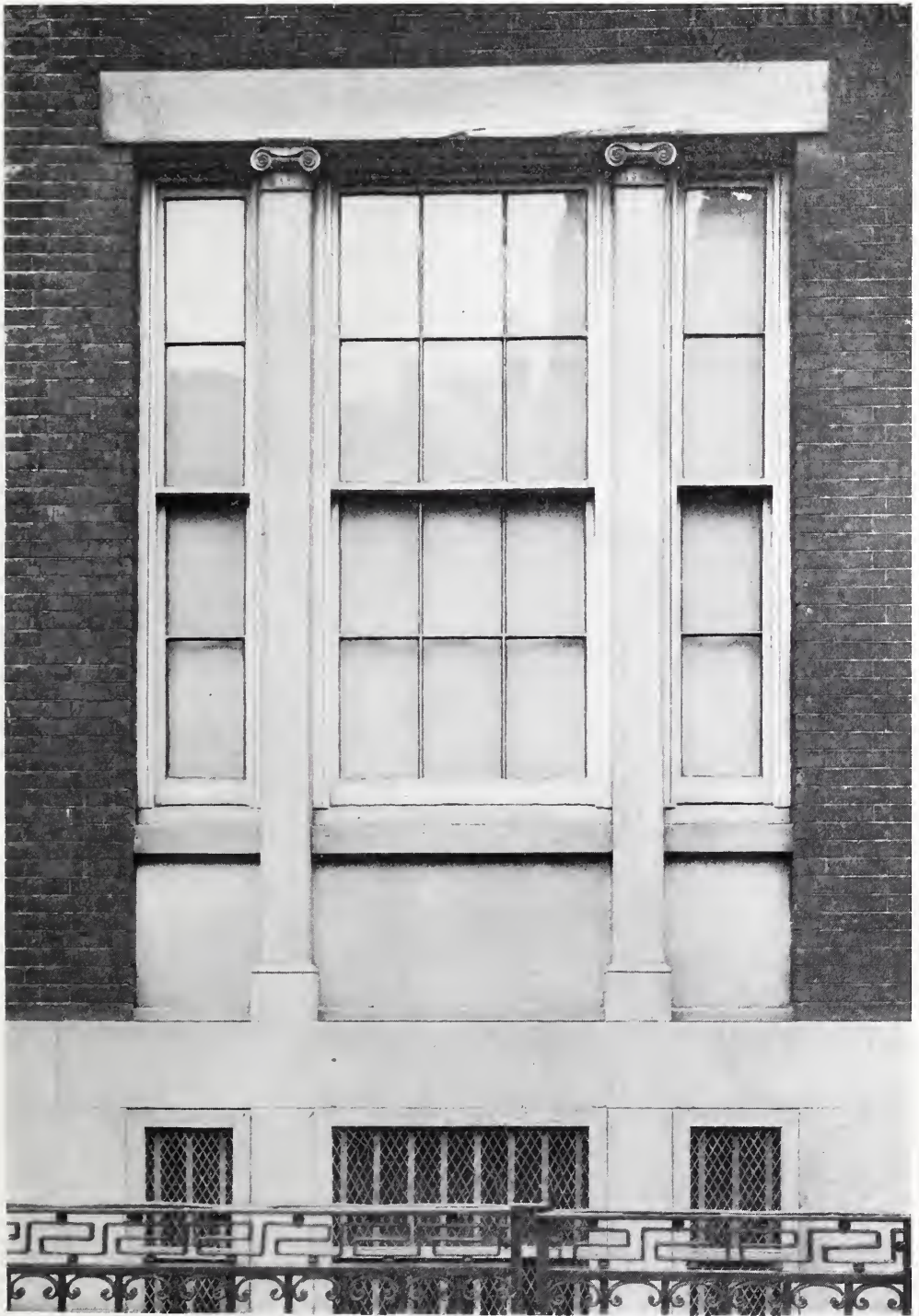
DETAIL OF A WINDOW FROM AN OLD HOUSE ON WALNUT STREET, PHILADELPHIA, PA. Note the Greek fret in the iron rail.
