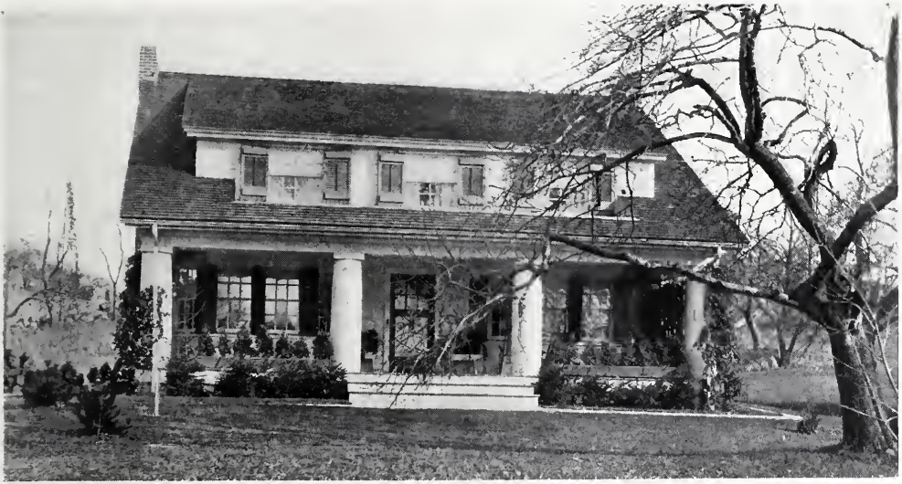
RESIDENCE OF ARTHUR W. WOOD, ESQ., ARDSLEY, N. Y. Arthur T. Remick, Architect.
