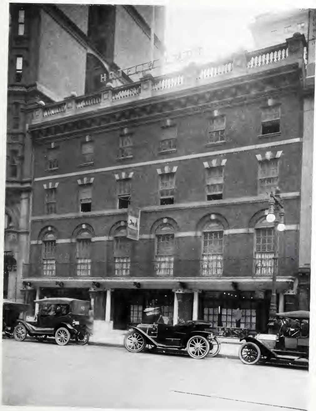
"THE LITTLE HOTEL WILMOT," SOUTH PENN SQUARE, PHILADELPHIA, PA. WILLIAM S. MCAULEY, ARCHITECT. An example of a well-advised return to local Georgian prototypes.
