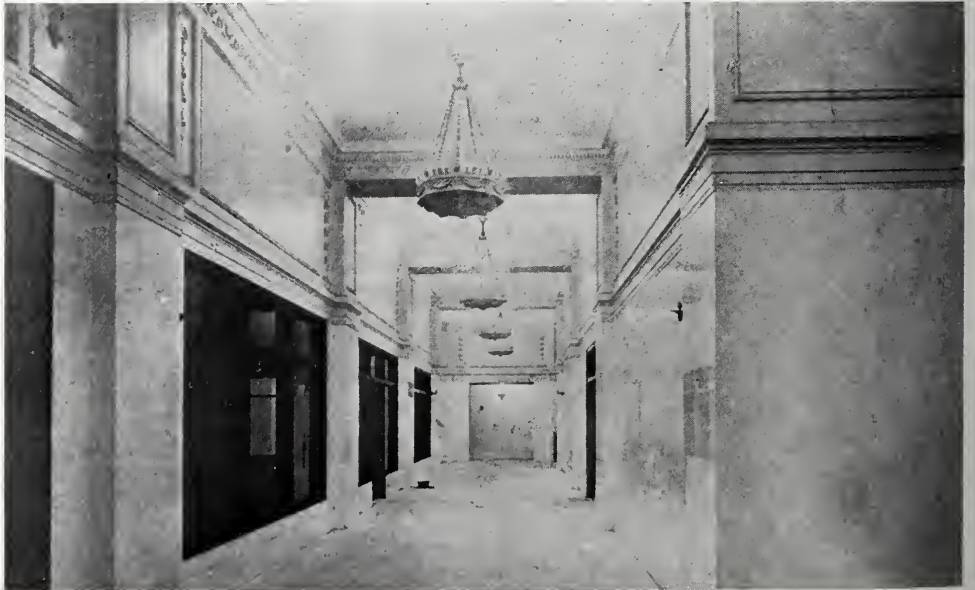
FIG. 9. THE SAME CORRIDOR WITH INDIRECT LIGHTINGS IN FIXTURES MORE HARMONIOUS WITH THEIR SETTING.
