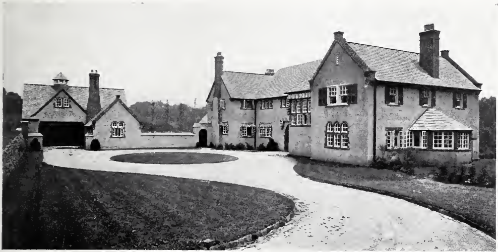
HOUSE AND GARAGE AT CHESTNUT HILL, PA. Edmund B. Gilchrist, Architect.
