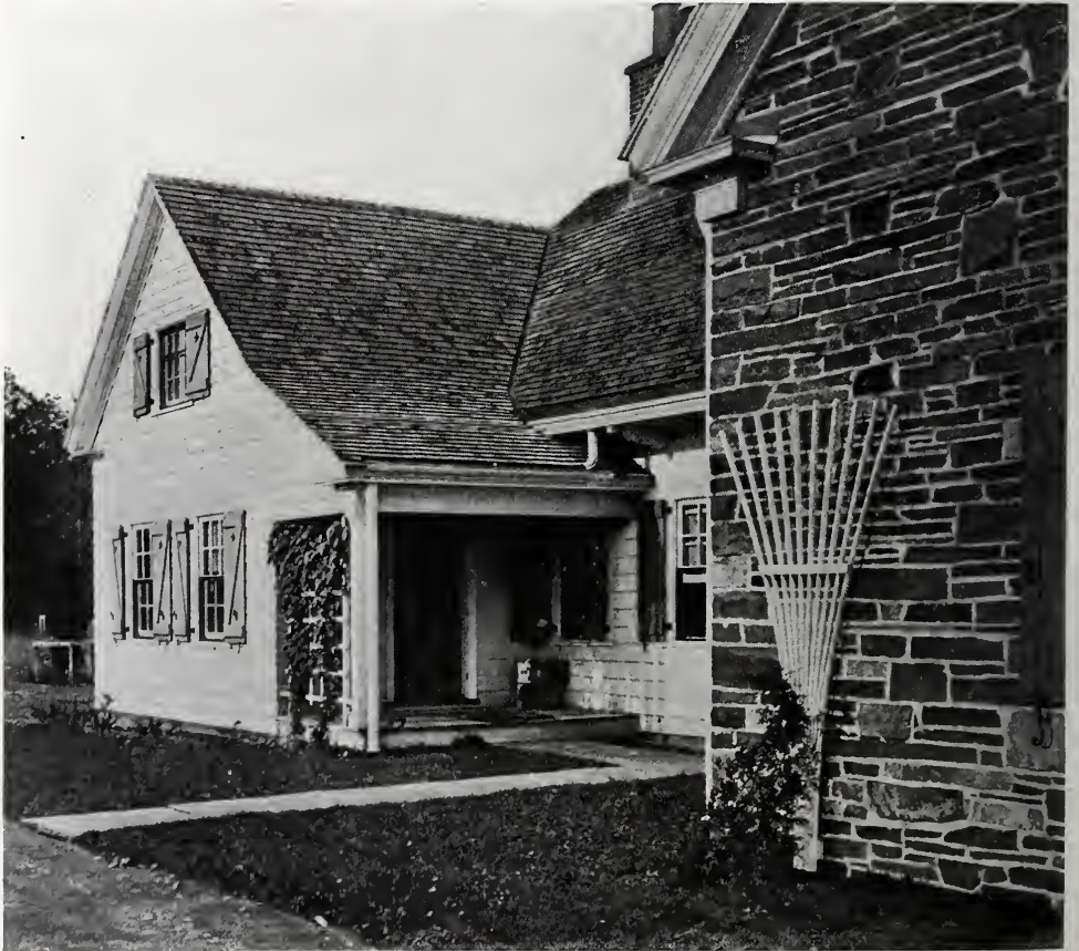
DETAIL OF WING, RESIDENCE OF JULES BREUCHAUD, ESQ., ULSTER CO., N. Y. Myron S. Teller, Architect.
