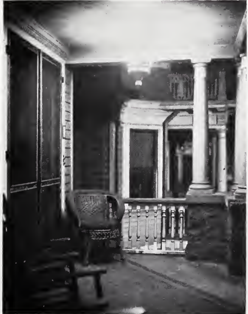
Fig. 10. Indirect lighting with 40-watt lamp and reflector equipment.
