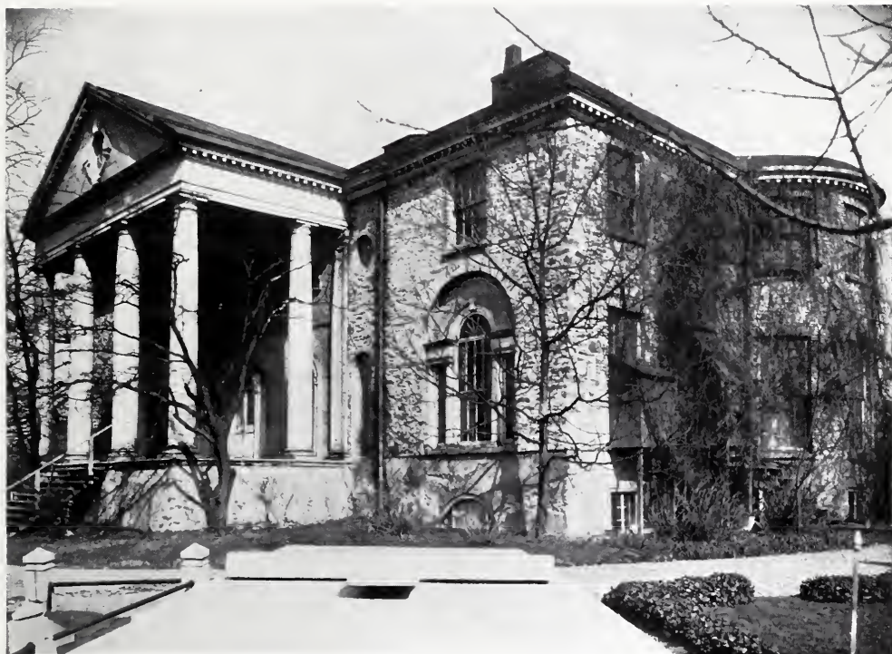
THE WOODLANDS, PHILADELPHIA, PA., SOUTH FRONT, BUILT CIRCA 1770. An example of the "Third Type" of Georgian.
