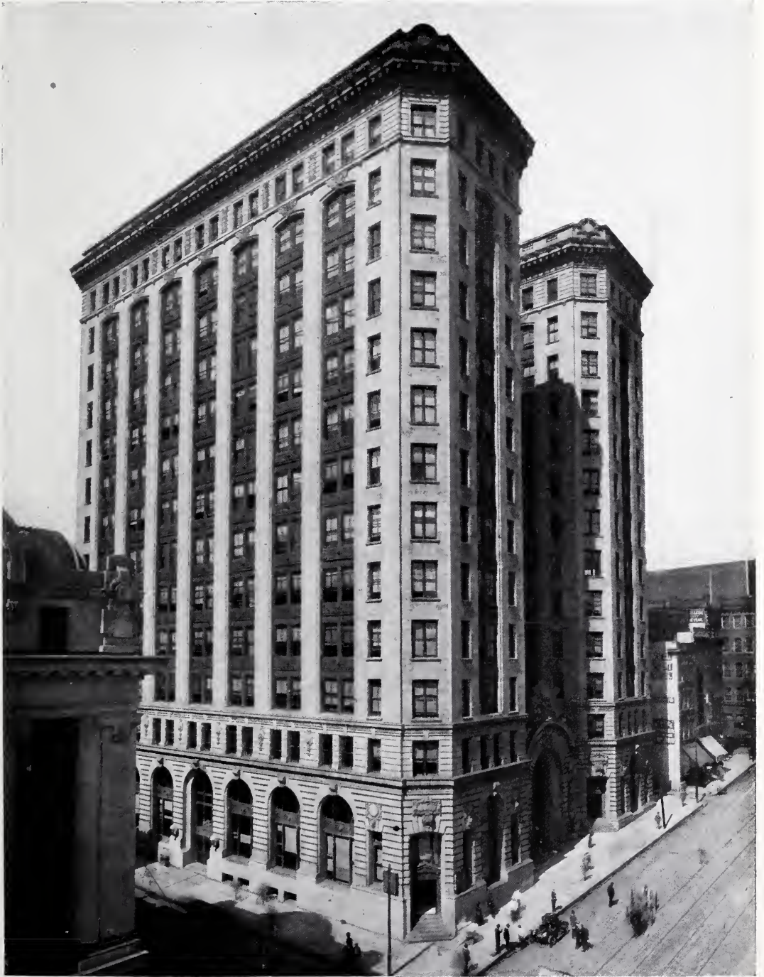
THE BALTIMORE AND OHIO OFFICE BUILDING, BALTIMORE, MD. PARKER, THOMAS & RICE, ARCHITECTS.
