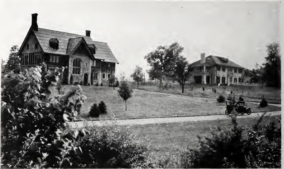
RESIDENCE OF LESLIE DANA, ESQ. (LOT 1 TO THE LEFT.) RESIDENCE OF J. S. BEMIS, ESQ., BRENTMOOR PARK, ST. LOUIS, MO. (LOT 2 TO THE RIGHT.)
