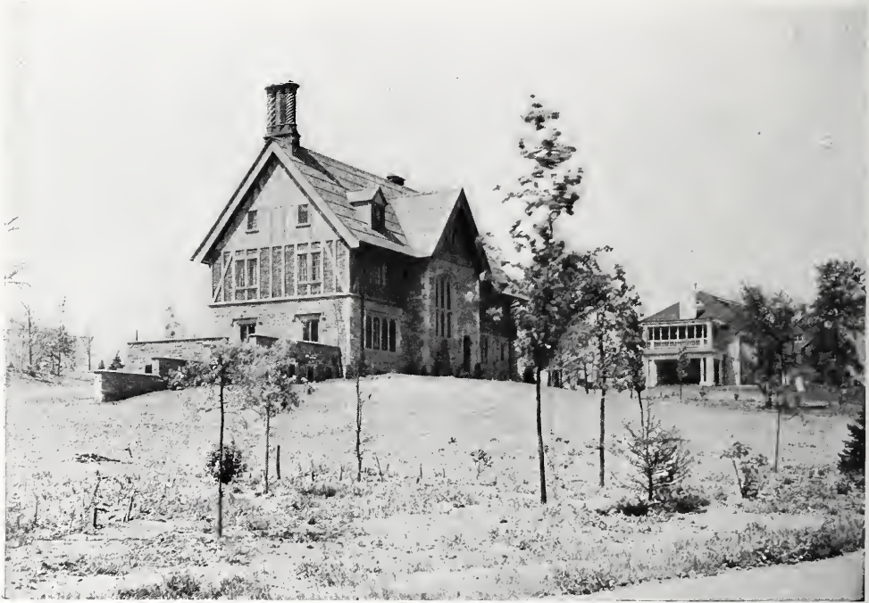
RESIDENCE OF LESLIE DANA, ESQ., BRENTMOOR PARK, ST. LOUIS, MO. (LOT 1.) Klipstein & Rathmann, Architects.
