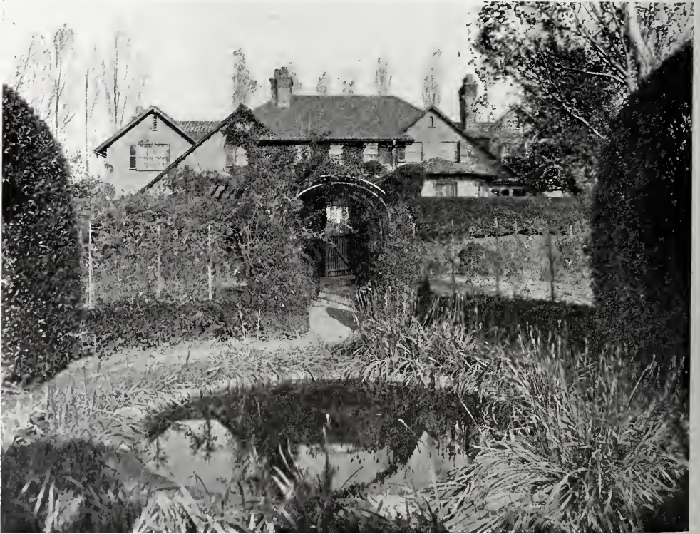
THE GARDEN FRONT, COUNTRY HOUSE AT GREAT NECK, L. I. Wilson Eyre & McIlvaine, Architects.
