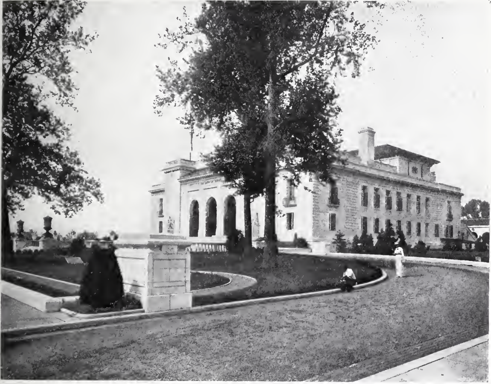
THE APPROACH—THE PAN-AMERICAN BUILDING, WASHINGTON, D. C.
