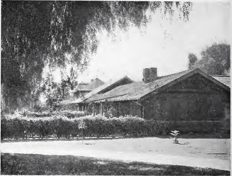
THE HOLLISTER RESIDENCE, HOLLYWOOD, CAL. Greene and Greene, Architects.
