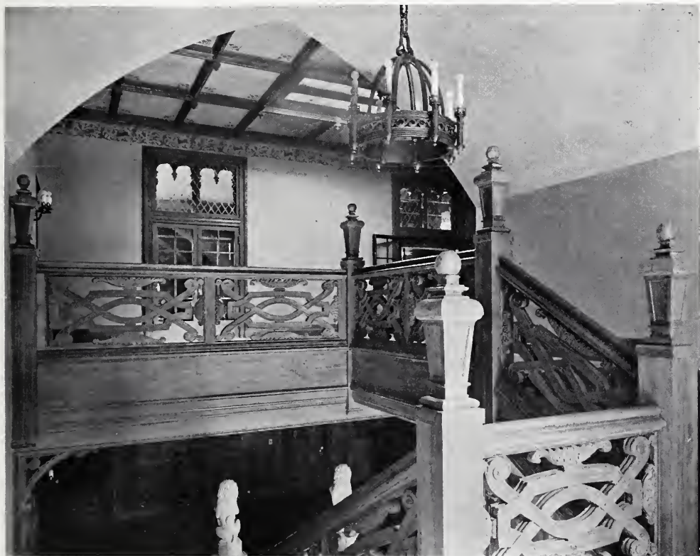
STAIR DETAIL—RESIDENCE OF F. F. BREWSTER, ESQ., NEW HAVEN, CONN. Stephenson & Wheeler, Architects.
