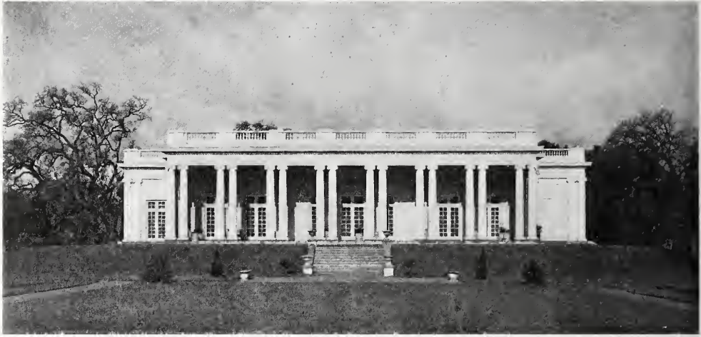
THE McNEAR RESIDENCE, MENLO PARK, CAL. Bliss and Faville, Architects.
