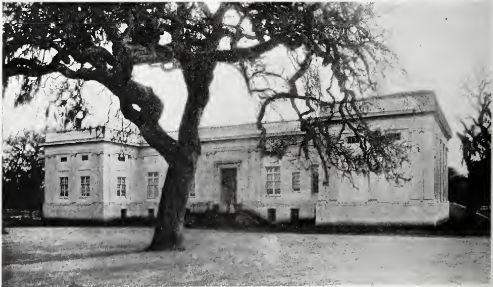
THE McNEAR RESIDENCE, MENLO PARK, CAL. Bliss and Faville, Architects.
