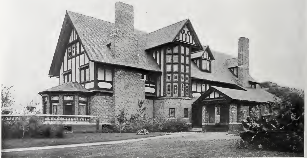
Showing how effectively an octagonally planned bay window may be gabled. For the sake of roof harmony all the roof-included dormers are gabled, and were carefully studied in perspective. The one-story bay is the only jarring note.
