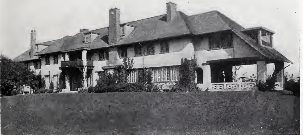
RESIDENCE OF HUGH J. MCBIRNEY, ESQ., LAKE FOREST, ILL. Howard Shaw, Architect.
