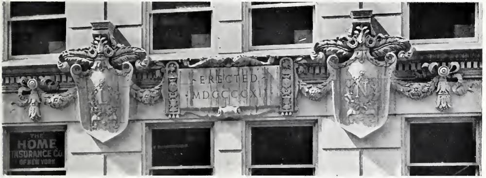
DETAIL AND INCISED LETTERING, THE LEADER-NEWS BUILDING, CLEVELAND, O. Charles A. Platt, Architect.
