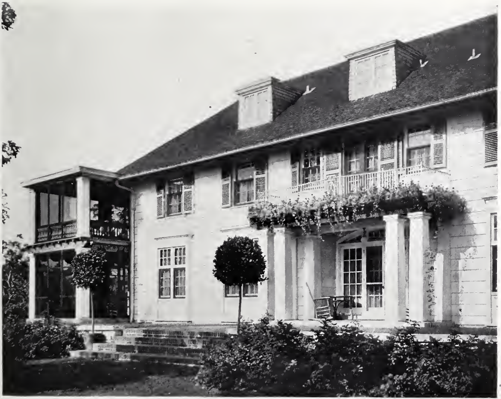
RESIDENCE OF R. C. SCHAFFNER, ESQ., HIGHLAND PARK, ILL. Howard Shaw, Architect.
