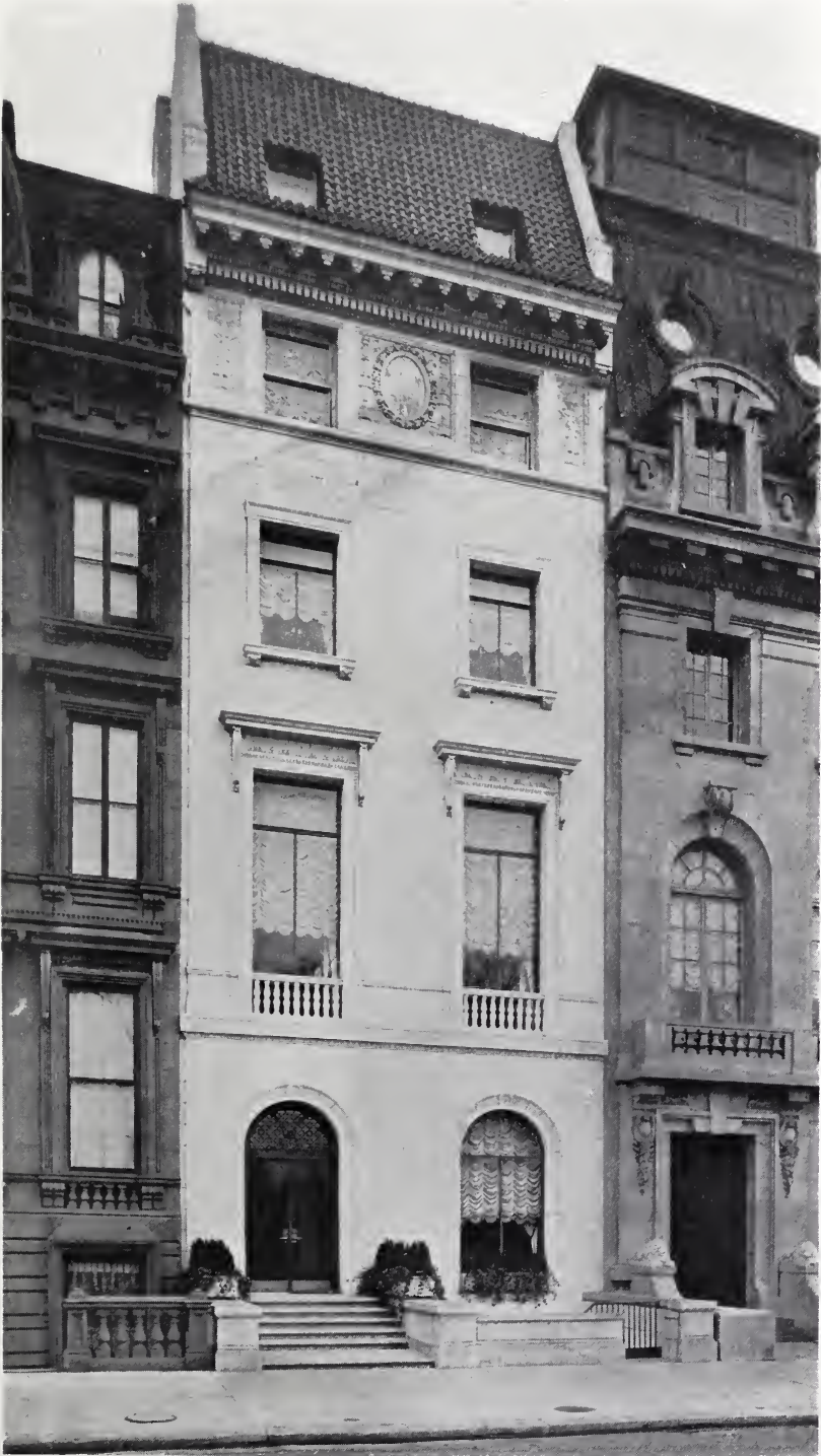
RESIDENCE OF J. W. HERBERT, ESQ. HARRY ALLAN JACOBS, ARCHITECT.
