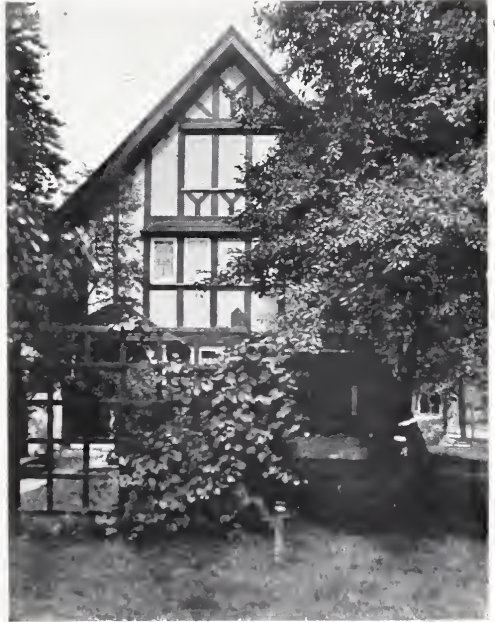
The gable of good pitch is particularly domestic in quality, and is always "indicated" where much finished attic space is wanted.
