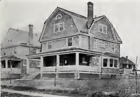
The use of a gambrel roof above two full stories gives a heavy and barn-like effect, even if the house (unlike the illustration) is well designed in itself.
