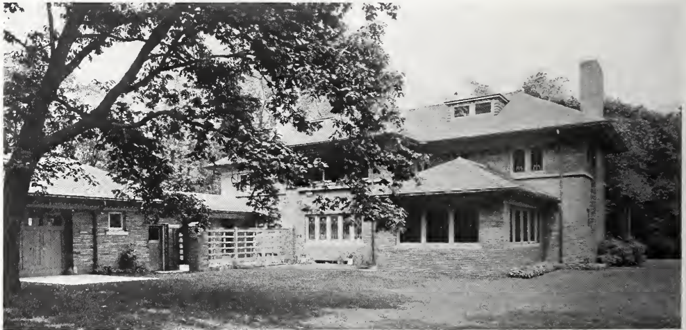
A house by Spencer and Powers at Oak Park, Ill., showing a reasonable maximum for the overhang of eaves. Roofed with light red shingle tiles and moulded hips. The main roof has a pitch of 5 in 8, and a maximum overhang of about four feet.
