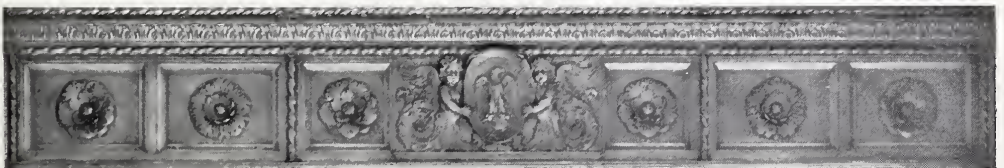
A DETAIL OF BRONZE, THE LEADER-NEWS BUILDING, CLEVELAND, O. Charles A. Platt, Architect.
