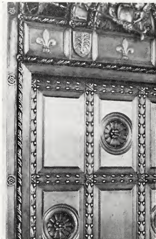
DETAIL OF ELEVATOR DOORS IN BRONZE, THE LEADER-NEWS BUILDING, CLEVELAND, O.
