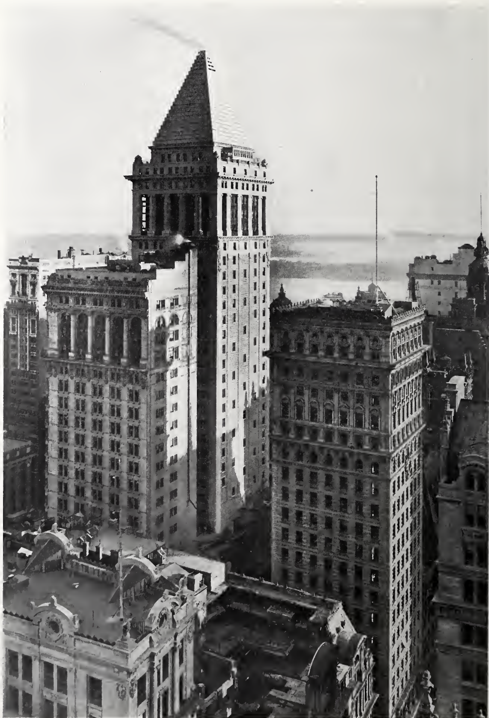
Photograph by Johnston & Hewitt. The smoke-stack of the building is carried out at the apex of the pyramidal roof.
