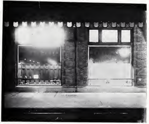
Fig. 2. Change effected by substituting reflectors of ordinary blotting paper for shades, which allowed too much light to pass above and below them.
