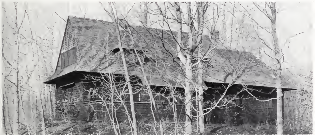
A shingle roof with close-trimmed gable end, and eaves carried across it to accentuate the low horizontal lines of the cottage. The hip-roofed dormers are inconspicuous against the rather steep roof.
