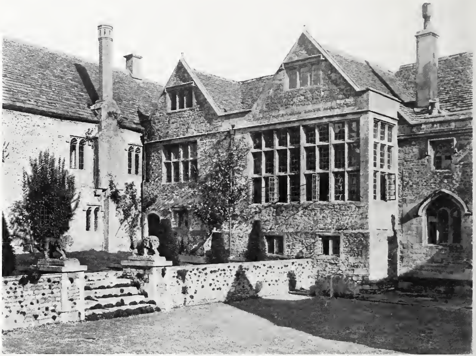
CASEMENT WINDOWS IN SOUTH WRAXHALL MANOR HOUSE, WILTSHIRE, ENGLAND.
