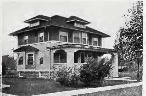
A clumsy and over-eaved dormer effect common in many American suburbs. It is a type of "real estate" house, built to sell.
