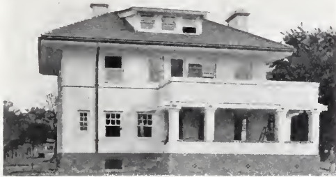
Eaves rather too wide and heavy, and the roof marred by the large central dormer.
