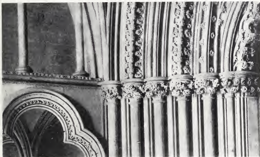
DETAIL OF THE WEST PORCH, ELY CATHEDRAL, ENGLAND.
