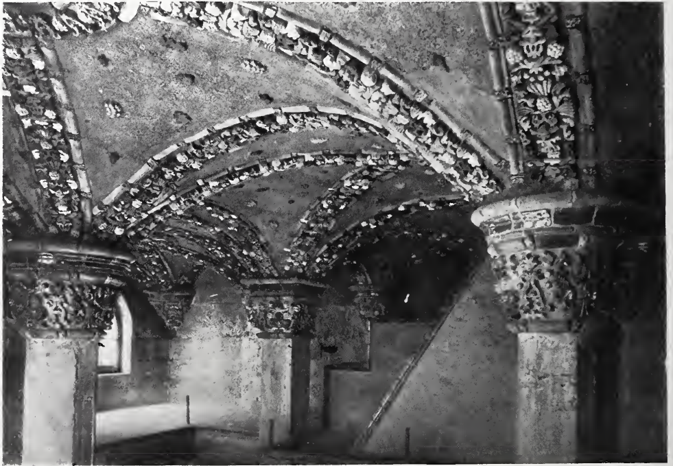
A PORTION OF THE LIBRARY CEILING.
