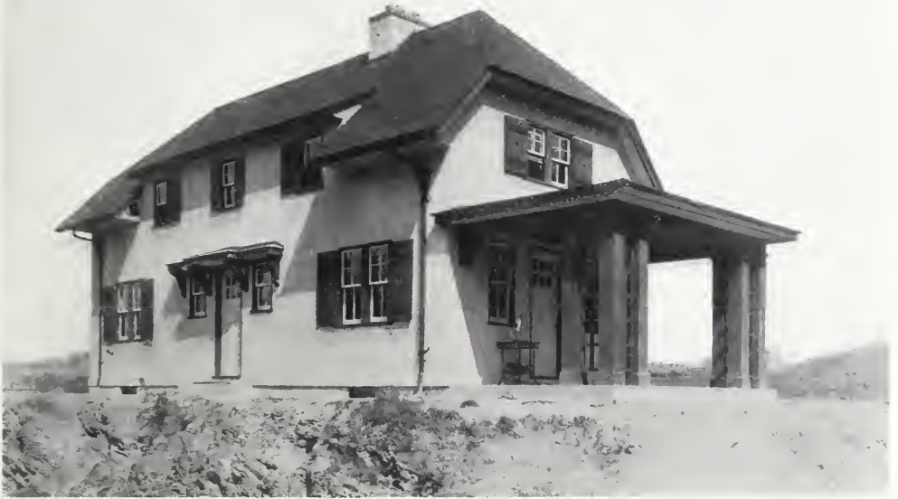
The construction of this house is stucco on wire lath, the whole being built for $3,500.
