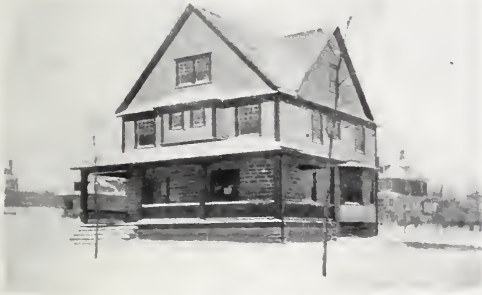
An awkward gable roof lacking preparation in the second floor plan for the cross-gable on the side, which is too large in proportion. The sketch shows a better treatment.
