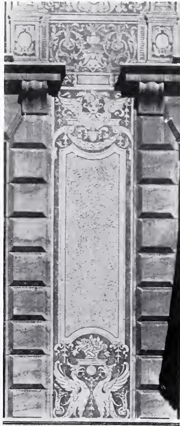
DETAIL OF A SGRAFFITO PANEL, FACADE AT 548 FIFTH AVENUE., NEW YORK CITY Carrère and Hastings, Architects Menconi, Decorator
