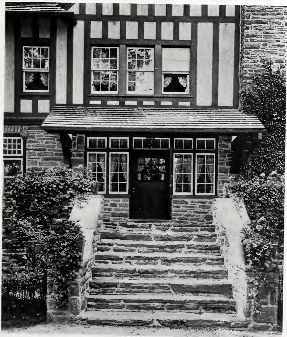
DETAIL—RESIDENCE OF VICTOR C. MATHER, ESQ., HAVERFORD, PA. Duhring, Okie and Ziegler, Architects.
