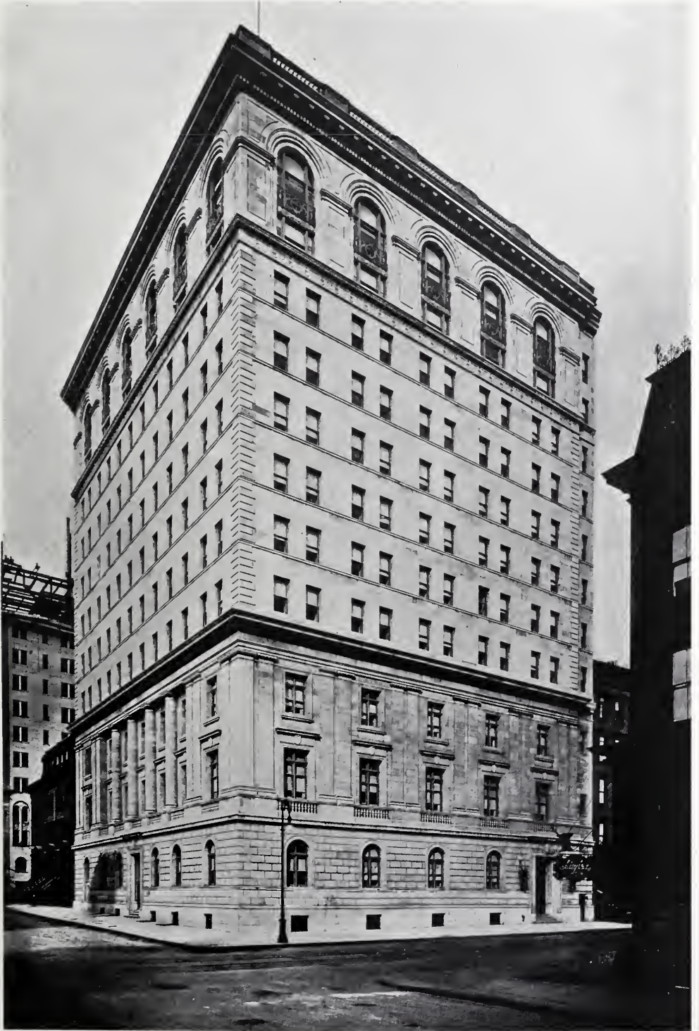
HEADQUARTERS BUILDING FOR THE YOUNG WOMEN'S CHRISTIAN ASSOC., NEW YORK CITY. DONN BARBER, ARCHITECT.
