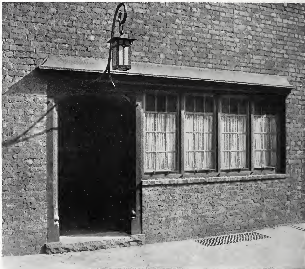
CASEMENTS GROUPED WITH A DOOR—ENTRANCE TO THE OFFICES OF MELLOR AND MEIGS, PHILADELPHIA, PA.
