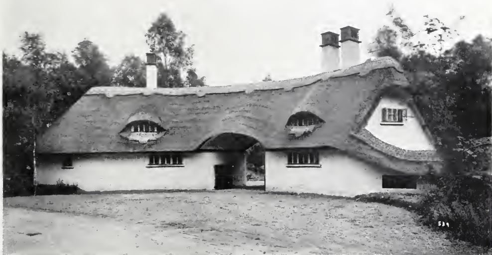
THATCHED STABLE WITH CASEMENT WINDOWS, POLLARD'S WOOD GRANGE, ENGLAND. Forbes and Tate, Architects.
