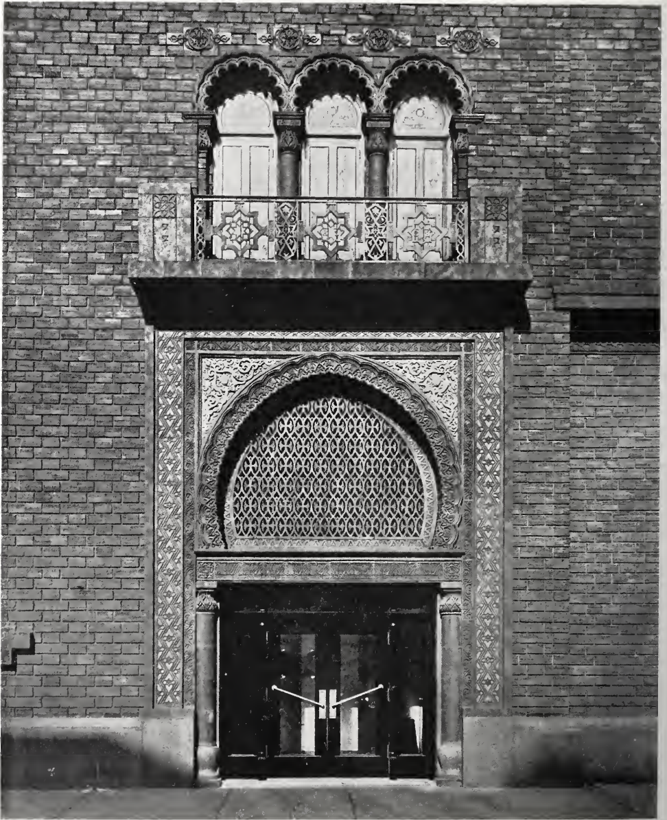
DETAIL OF ENTRANCE ON OHIO STREET, MEDINAH TEMPLE, CHICAGO, ILL. Huehl and Schmid, Architects.
