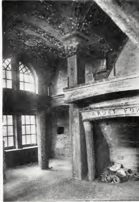
A CORNER IN THE LIBRARY. Concrete and tile are virtually the sole materials used in the house.
