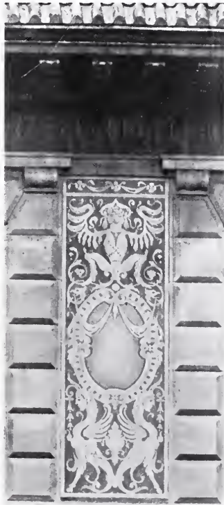
DETAIL OF A SGRAFFITO PANEL. FACADE AT 548 FIFTH AVE., NEW YORK CITY. Carrère and Hastings, Architects. Menconi, Decorator.
