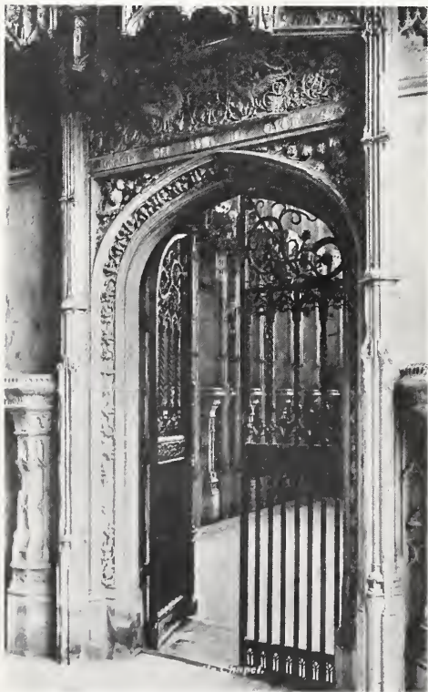
DETAIL OF DOOR, BISHOP WEST'S CHAPEL, ELY CATHEDRAL.
