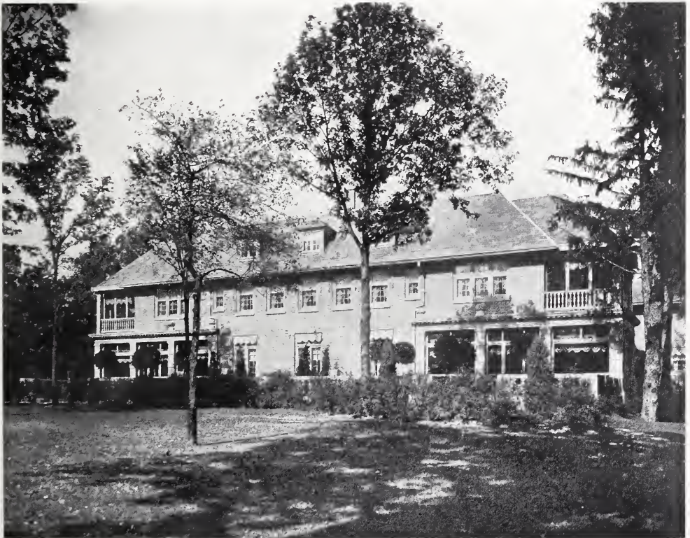
RESIDENCE OF FINLEY BARRELL, ESQ., LAKE FOREST, ILL. Howard Shaw, Architect.
