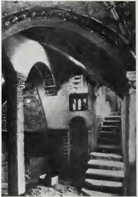
THE ALCOVE AND STAIRWAY LEADING TO THE BREAKFAST ROOM.
