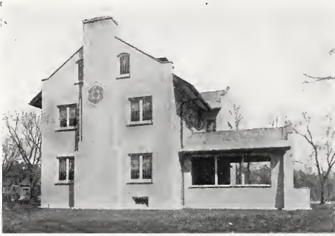
The masonry character of a stucco coated house of hollow tile is emphasized by the substitution of tile coped gable ends for overhanging verges.
