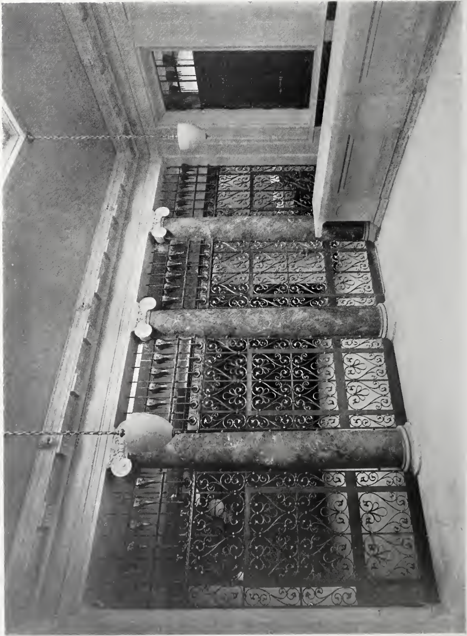
NEWSPAPER OFFICE, THE LEADER- NEWS BUILDING, CLEVELAND, O. CHARLES A. PLATT, ARCHITECT.
