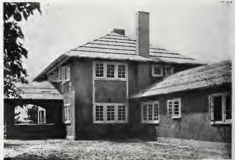
Doubling the shingles every seventh course gives a rather agreeable horizontal texture to a shingle roof.
