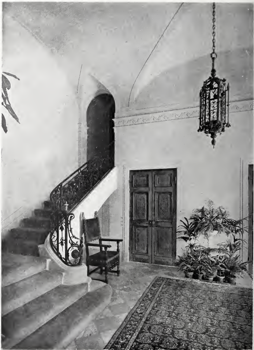
ENTRANCE HALL, RESIDENCE OF OAK- LEIGH THORNE, ESQ., NEW YORK CITY. ALBERT JOSEPH BODKER, ARCHITECT.
