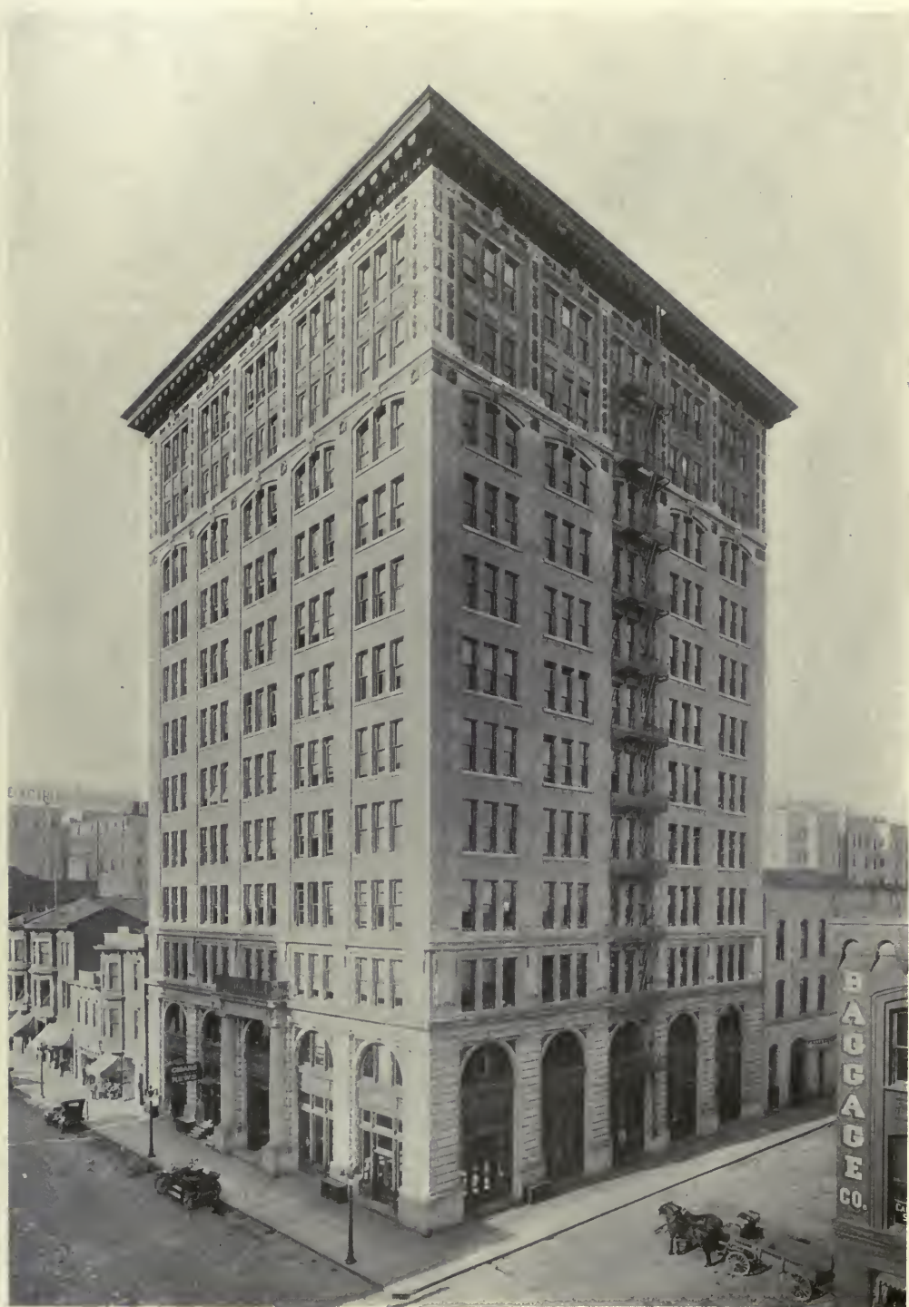
THE WELLS FARGO BUILDING, PORTLAND, OREGON. BENJ. WISTAR MORRIS, ARCHITECT.
