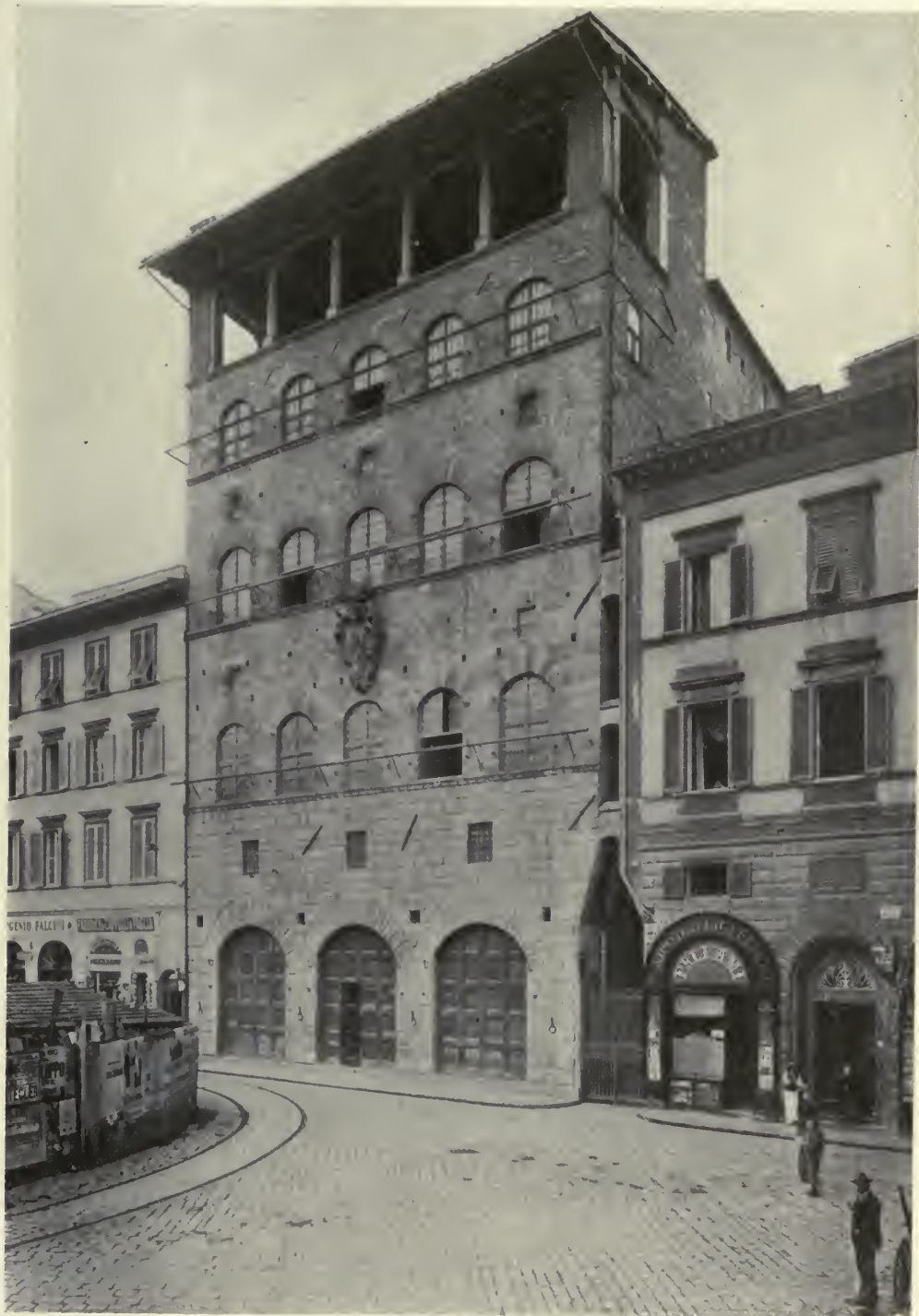
FAÇADE—THE PALAZZO DAVANZATI, FLORENCE, ITALY.
