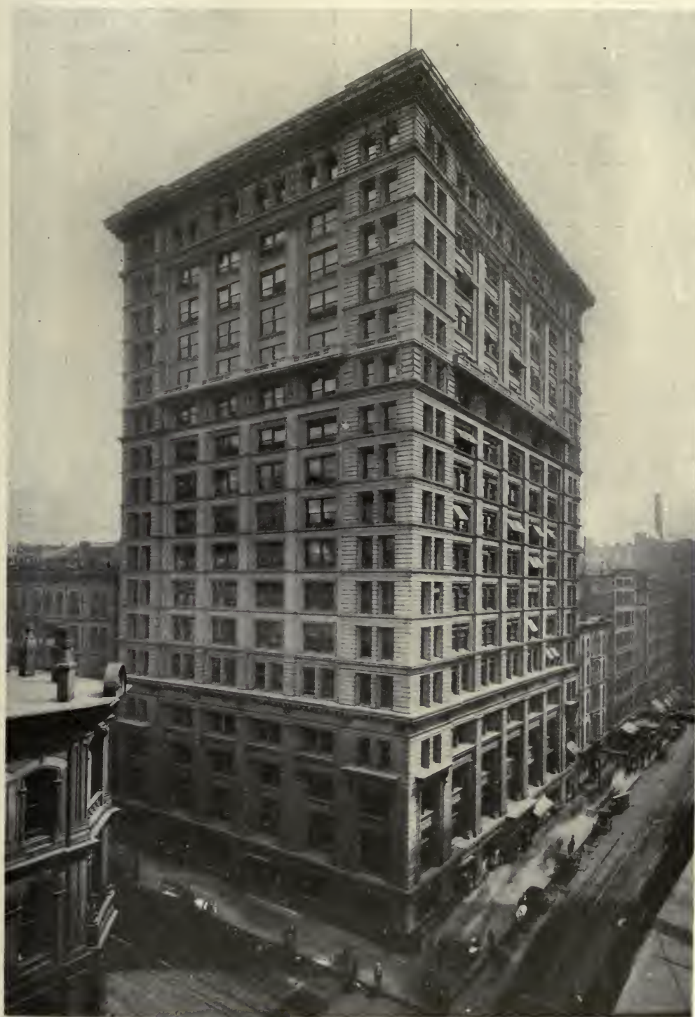
THE TRIBUNE BUILDING, CHICAGO. HOLABIRD & ROCHE, ARCHITECTS.
