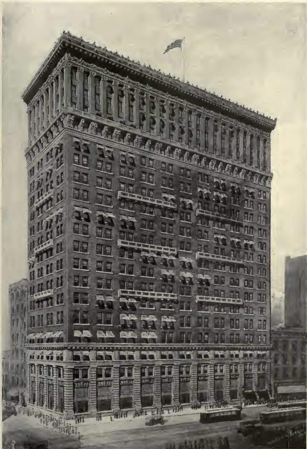
NEW BUILDING, CHICAGO TELEPHONE COMPANY, CHICAGO, ILLINOIS. HOLABIRD & ROCHE, ARCHITECTS.
