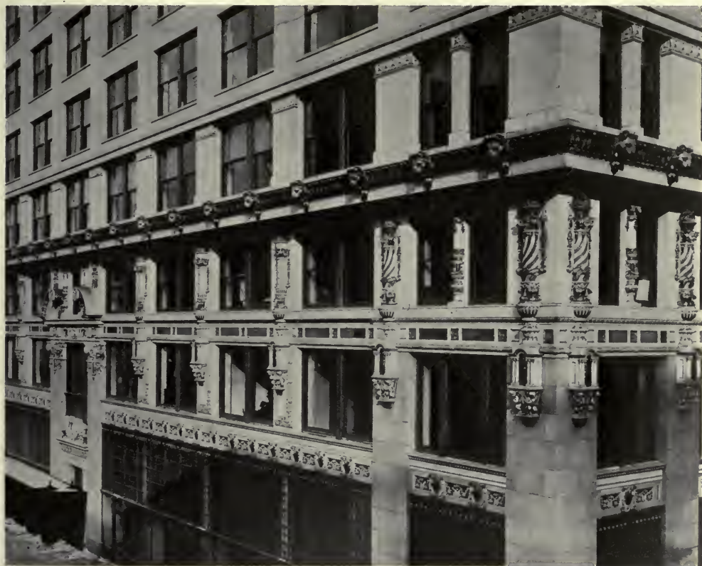
DETAIL OF THE HEARST BUILDING, CHICAGO, ILL.
