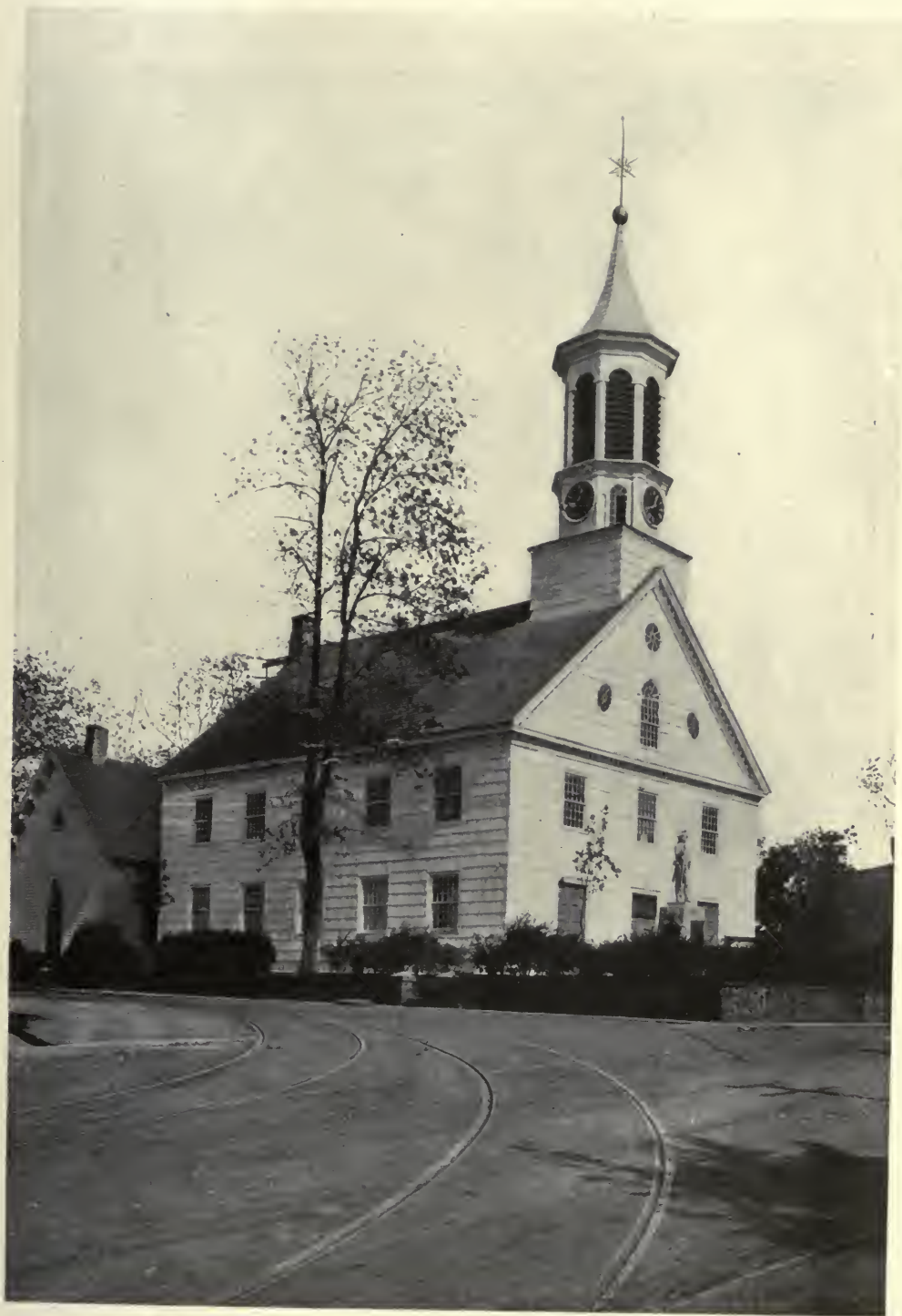
CHURCH AT SPRINGFIELD, NEW JERSEY.
