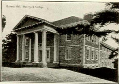
Roberts Hall, Haverford College. Haverford, Pa. Cope & Stewardson, Architects.
