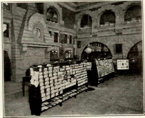
Interior of Library (1891). Philadelphia, Pa. Furness, Evans & Co., Architects.
