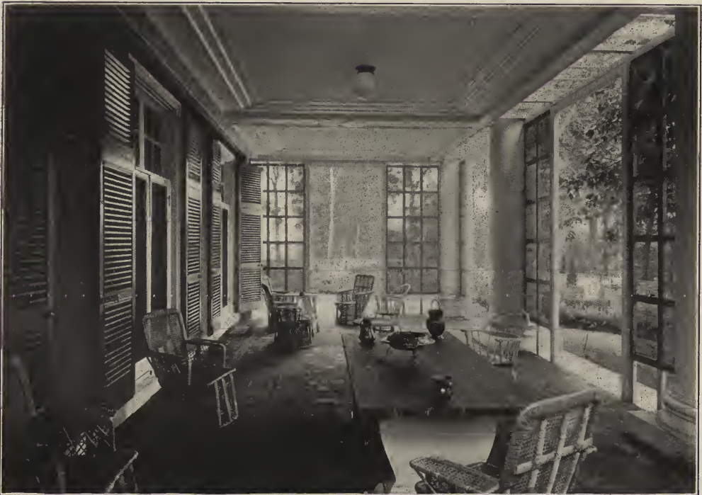
HOUSE OF MR. MARSHALL SLADE—ENCLOSED VERANDA.
