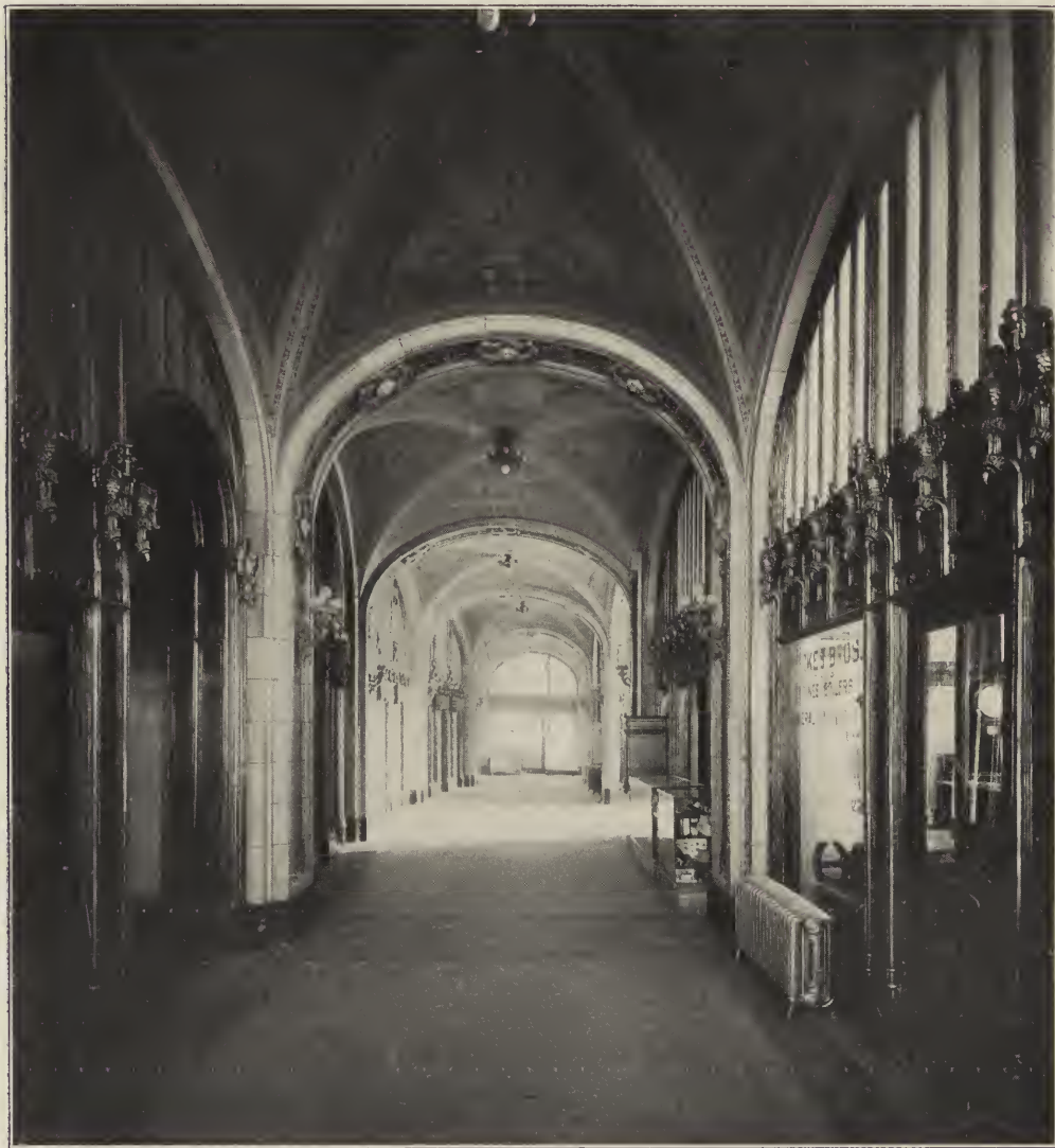
THE WEST STREET BUILDING—THE ENTRANCE CORRIDOR, LOOKING TOWARDS ALBANY ST.
