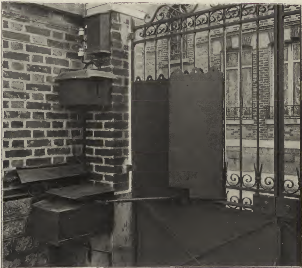
VILLA FERIA ELECTRA—INSIDE THE ALLEY, SHOWING MECHANISM FOR OPENING AND CLOSING GATES; IN THE UPPERMOST BOX IS THE TELEPHONE BY MEANS OF WHICH THE INVISIBLE HOST GREETED HIS APPROACHING GUEST.
