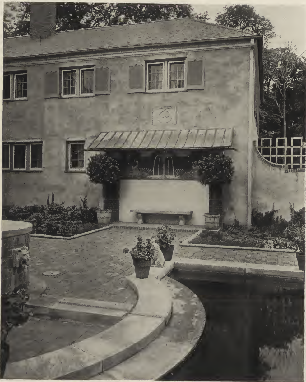
HOUSE OF MR. A. C. BARTLETT—DETAIL OF COURTYARD. Lake Geneva, Ill.
