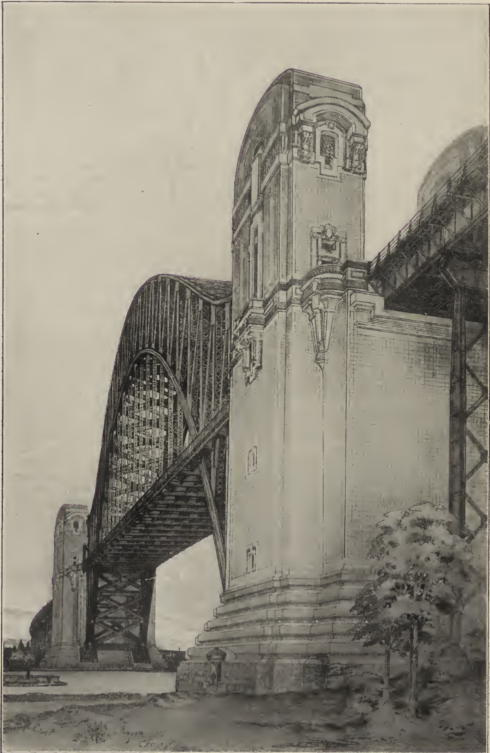
NEW YORK CONNECTING RAILROAD BRIDGE ACROSS THE EAST RIVER—VIEW WEST FROM THE LONG ISLAND PYLON.
