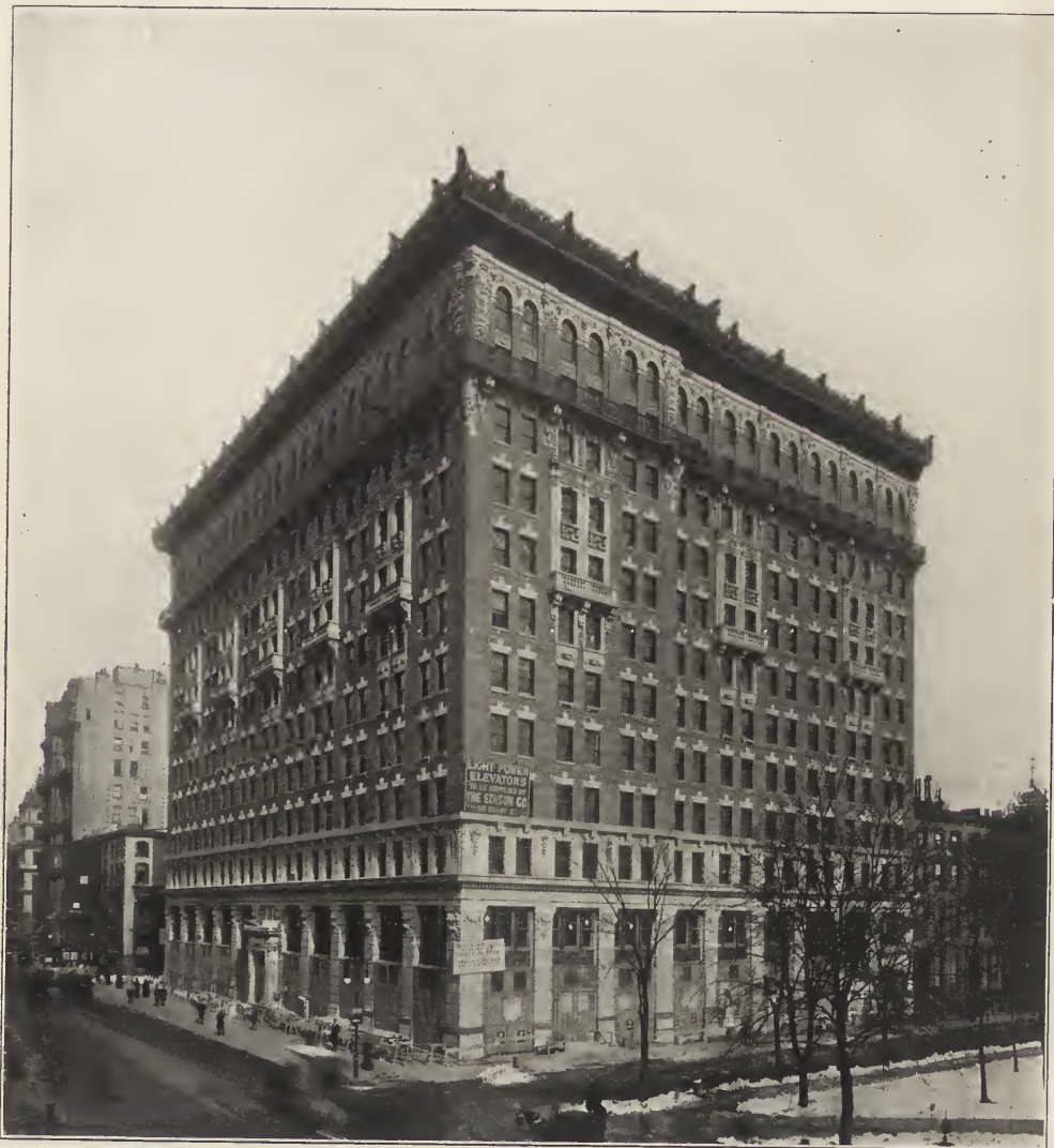
THE BRUNSWICK BUILDING.
