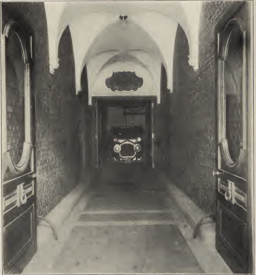
FIG. 3. RESIDENCE OF ERNEST FLAGG, ARCHITECT—PORTE-COCHERE, SHOWING AUTOMOBILE ON THE LIFT.
