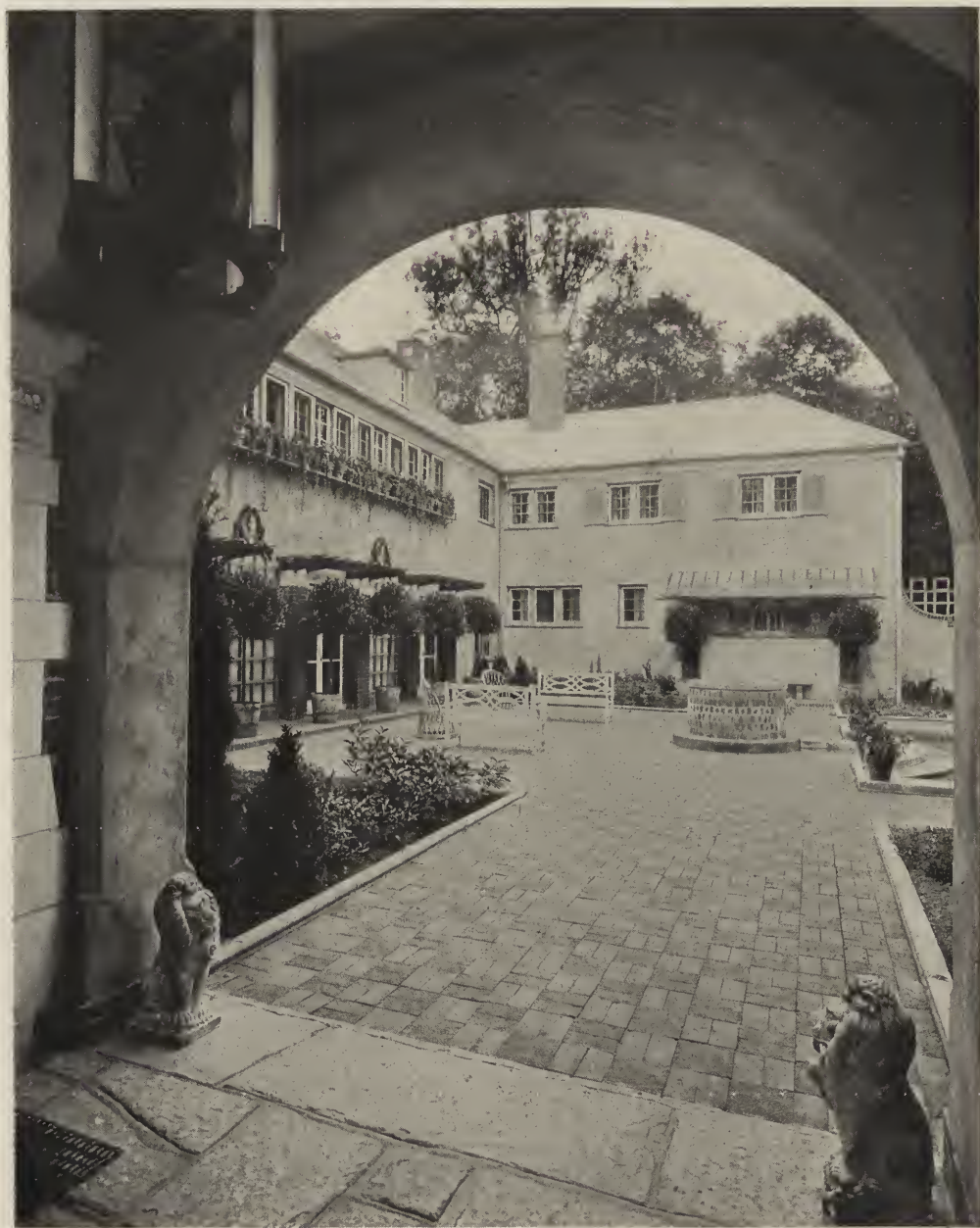
HOUSE OF MR. A. C. BARTLETT—VIEW INTO COURTYARD.
