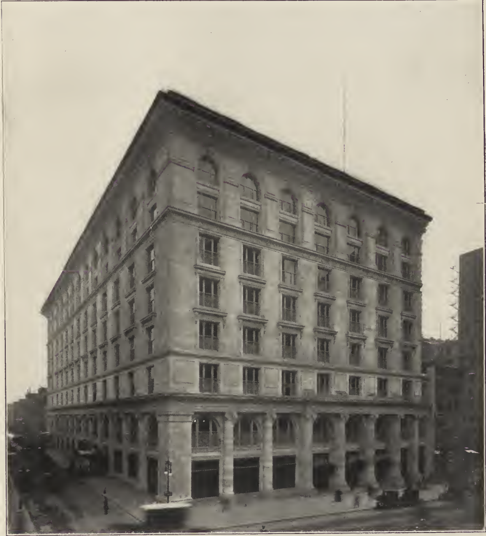
THE ALTMAN BUILDING.
