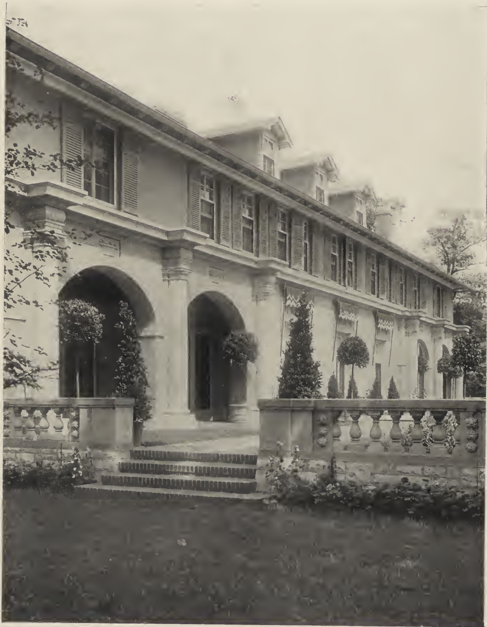
HOUSE OF MR. E. L. RYERSON—TERRACE.
