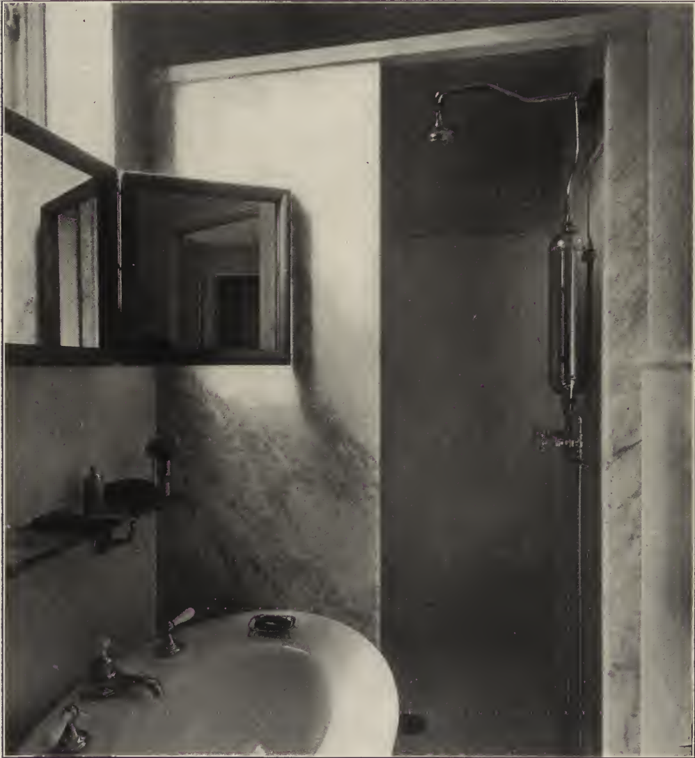
FIG. 27. RESIDENCE OF ERNEST FLAGG, ARCHITECT—BATHROOM, SHOWING RAIN BATH. 40th St., near Park Ave., New York.
