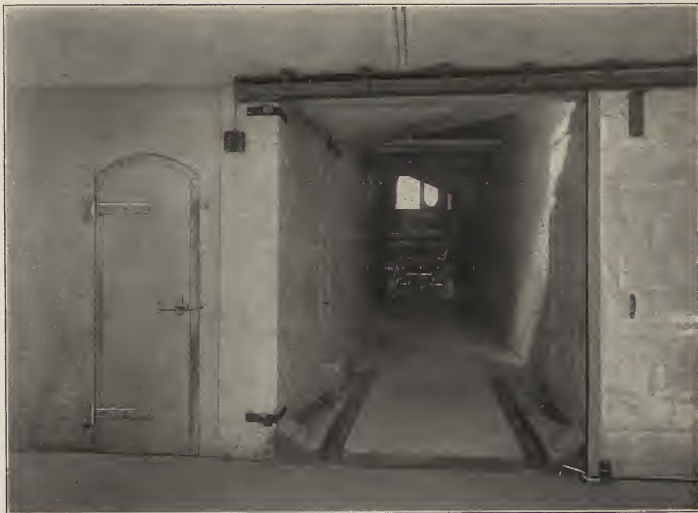
FIG. 8. RESIDENCE OF ERNEST FLAGG, ARCHITECT—VIEW IN GARAGE, LOOKING TOWARD AUTOMOBILE LIFT. 40th St., near Park Ave., New York.
