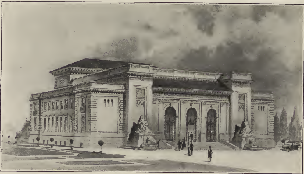
THE NEW BUILDING OF THE INTERNATIONAL BUREAU OF AMERICAN REPUBLICS. Washington, D. C.
