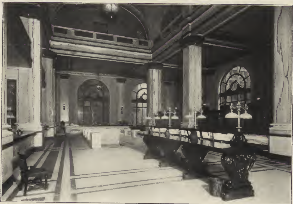
FIG. 1. BANKING ROOM, ON GROUND FLOOR.
