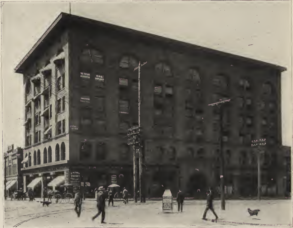
4.—THE DOOLEY BUILDING.
