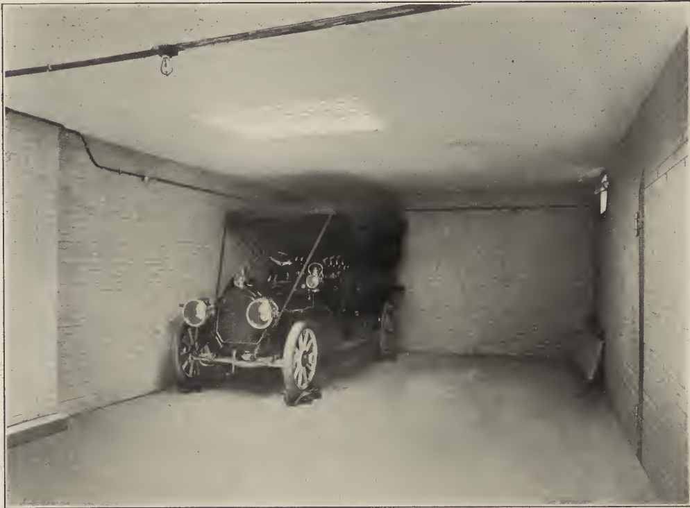
FIG. 7. VIEW IN THE GARAGE, LOOKING EAST.
