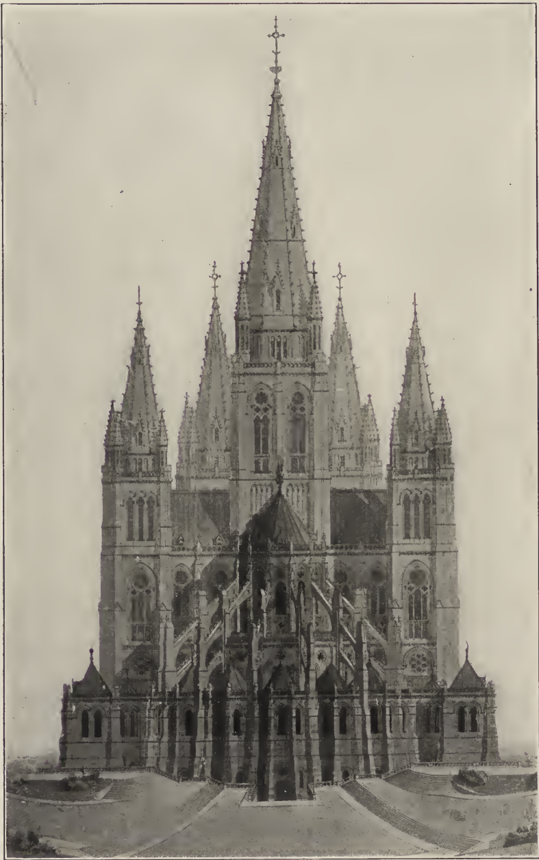
THE CATHEDRAL OF KOEKELBERG—REAR ELEVATION. Brussels, Belgium. M. Langerock, Architect.
