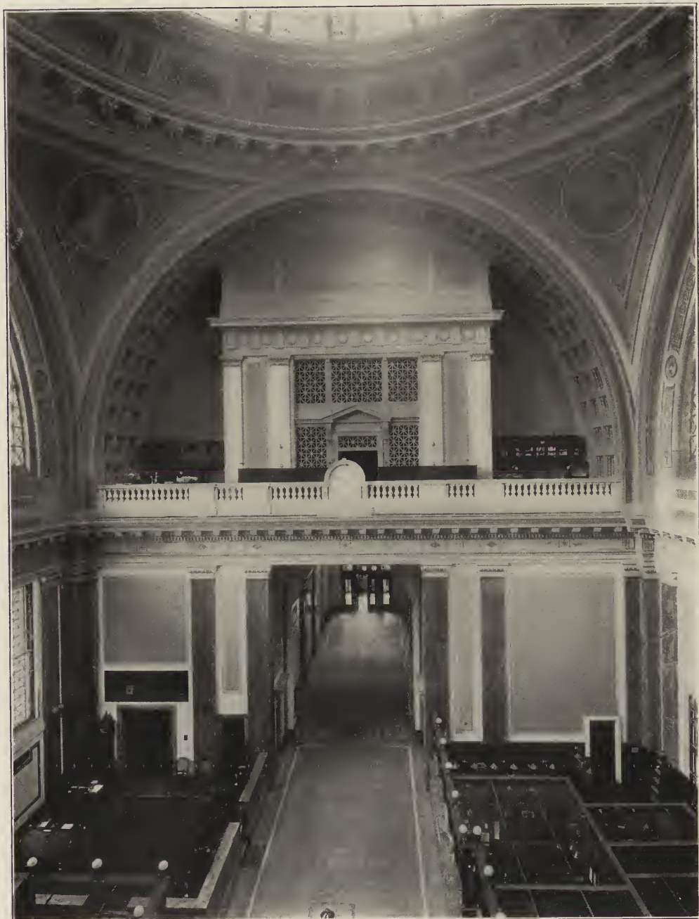
THE NEW CHEMICAL NATIONAL BANK—THE BANKING ROOM. LOOKING TOWARD THE ENTRANCE.
