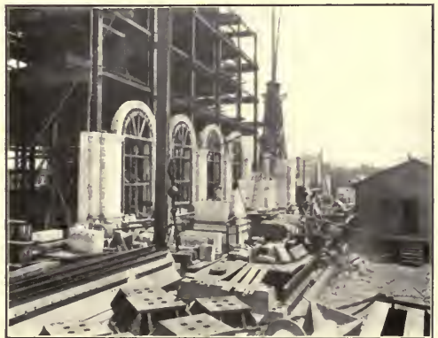
THE TERMINAL IN THE COURSE OF CONSTRUCTION.
