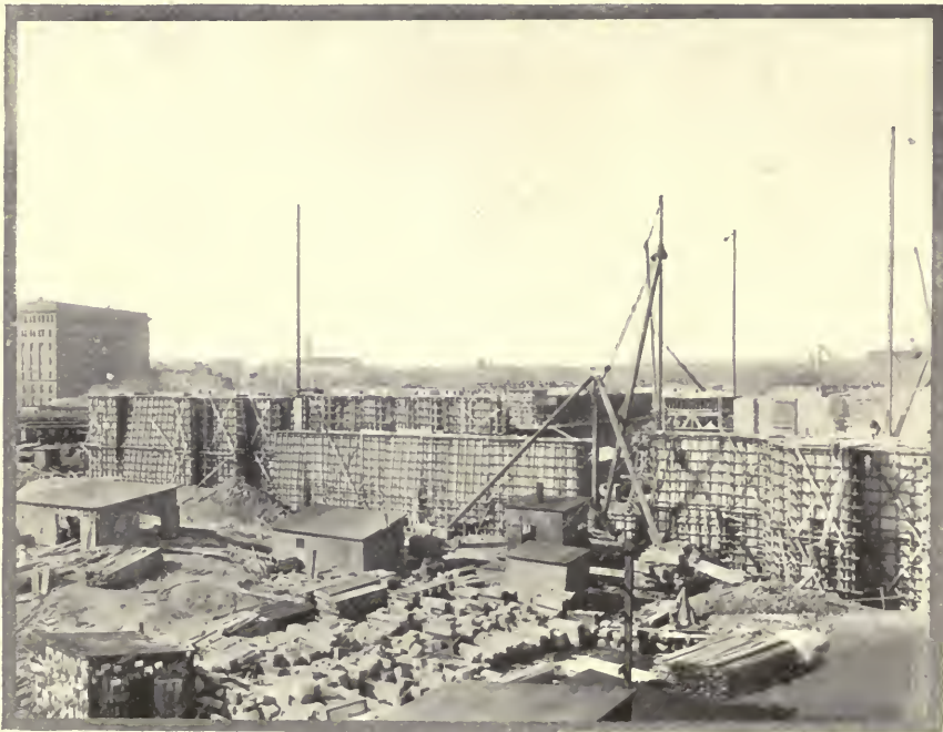
FIG. 5. THE WASHINGTON TERMINAL UNDER CONSTRUCTION.
