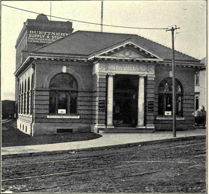
CHARTIERS TRUST CO. BUILDING.
