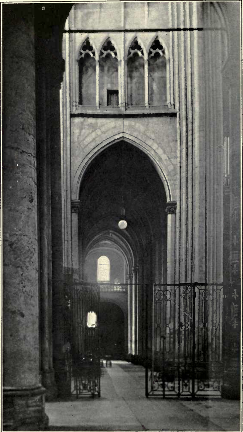
FIG. 12. THE CHURCH OF ST. QUENTIN, RIGHT AISLE. FROM THE CHOIR, LOOKING THROUGH THE TRANSEPT.
