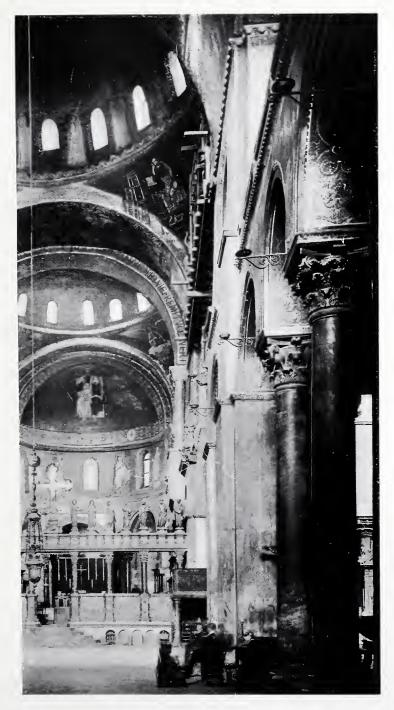
FIG. 3. SOUTH SIDE OF THE NAVE OF ST. MARK'S. From a Brooklyn Institute Survey photograph. Showing the changes of direction in the vertical lines.
