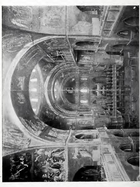
FIG. 1. ST. MARK'S, VENICE. THE NAVE IN PARALLEL PERSPECTIVE. FROM A BROOKLYN INSTITUTE SURVEY PHOTOGRAPH. THE AMOUNT OF WIDENING IS SHOWN BY FIG. 2.
