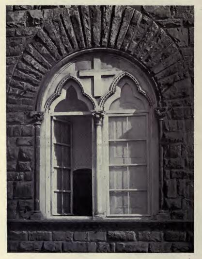
Fig. 5 bis. Detail of the Palazzo Vecchio, with tooled mouldings, which yet are effective by contrast of their sharp-edged and distinctly marked lights and darks with the irregular lighting on the rough surfaces.
