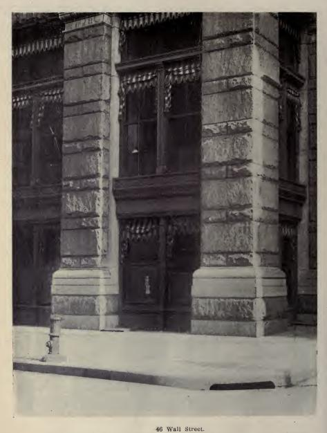
Rock-faced work in piers, contrasting with tooled work of inner jambs of windows and of moulded base-course a little above the side walk.
