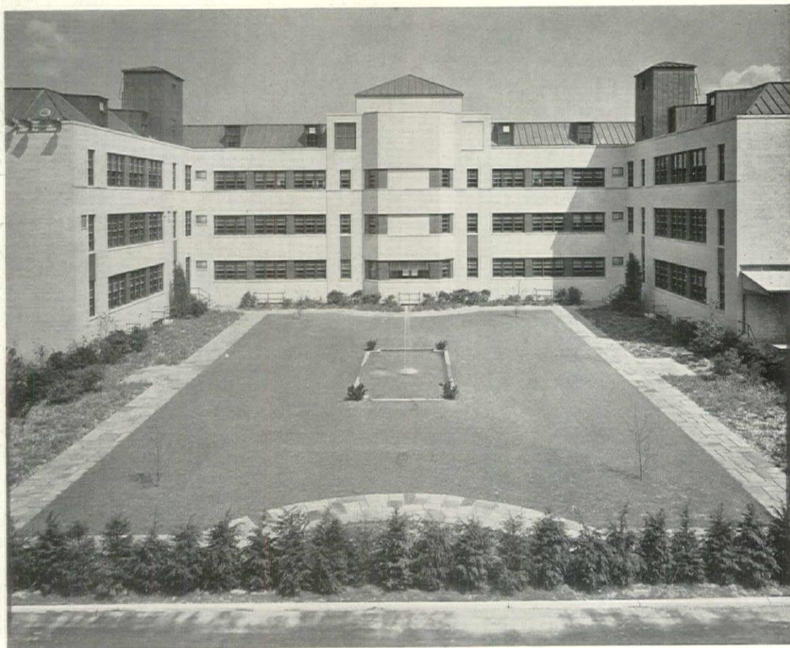
All the buildings are treated in the same manner with buff and purplish red brick, gable trim with occasional accents of buff. The clock is black. Facing on the administration building, seen from the rear, is copper. Here again fenestration has a horizontal character.
