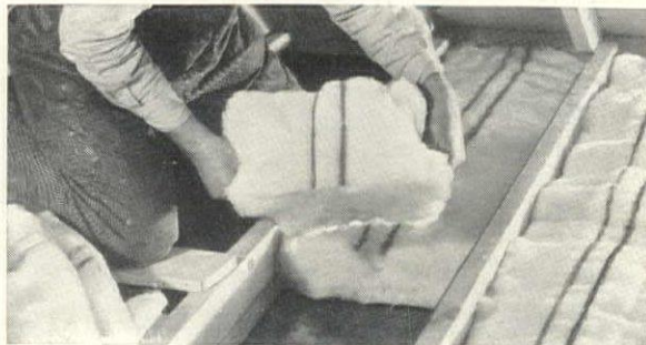
RED TOP JUNIOR BAT WOOL—in smaller sizes for use in complicated framing plans.
