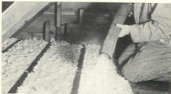
RED TOP NODULATED AND GRANULATED WOOL—in loose form for pouring or "blow-in."
