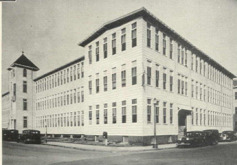
Section of Attleboro Associated Jewelers Building, Attleboro, Mass., re-sided with Timbertex Colonial Asbestos cement Shingles
