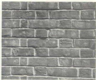
Textures in brickwork (left to right): Smooth brick of hand molded type with concave tooled joints; over-burned brick with rough, contrast-
