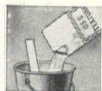
1. Painter mixes Textone with water as needed.
