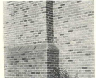
ing joints; light colored brick, occasional stretchers skintled; a combination of contrasting joints and occasional over-burned brick
