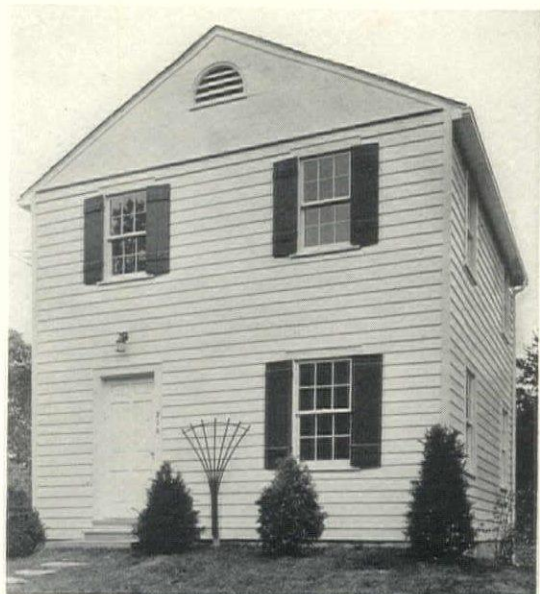
MODEL HOUSE CONSTRUCTED BY THE LUMBER INDUSTRY FROM PLANS DEVELOPED BY FHA FOR TECHNICAL BULLETIN NO. 4
