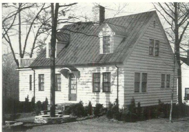
Here copper graces a really "small house," built as a Model F. H. A. home by Andrew H. Larsen at Waterbury, Conn.
