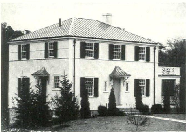
This home with Anaconda Copper roof is in Newton Highlands, Mass. Built by Davis & Vaughan, Boston, Mass.
