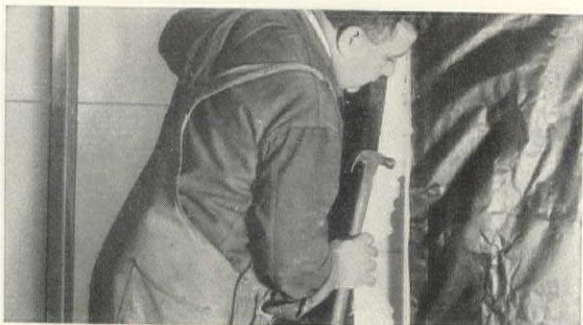
Showing stud application. Backed with heavy waterproof paper. RED TOP STRIP WOOL is easy to nail.
