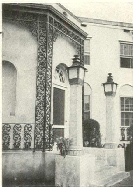
Smyser-Royer Company Cast Iron Veranda Design No. 69 White Estate, Miami, Fla. Architect: John Mead Howells, 156 E. 46th St., N. Y. C.
