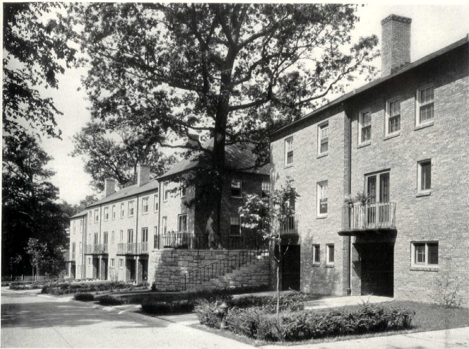
The rear of the group shown on the opposite page, with service entrances and garages on the road frontage
