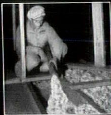
Gimco is easily and quickly blown over the top floor ceiling or into the side walls of homes already built. No muss—no dirt.
