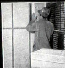
Gimco Sealal Bats are easily fitted between studs in buildings under construction. Can be easily cut to fit irregularly shaped spaces.
