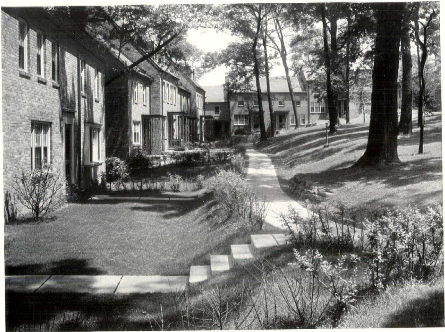
An interior court of the second unit. Considerable effort and expense were devoted to preserving the existing trees
