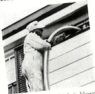
LOOSE-FILL which is blown between studdings and joists by special pneumatic process.
