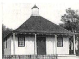
Kenmar Copper Roof. Tuck Shop, St. Georges School, Newport, R. I. Architect: W. T. Aldrich.
