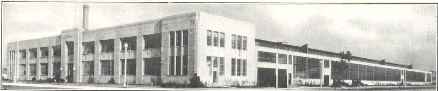
Genasco Trinidad Bonded 10-Year Built-up Roof, Pepsodent Company Plant, Chicago.
