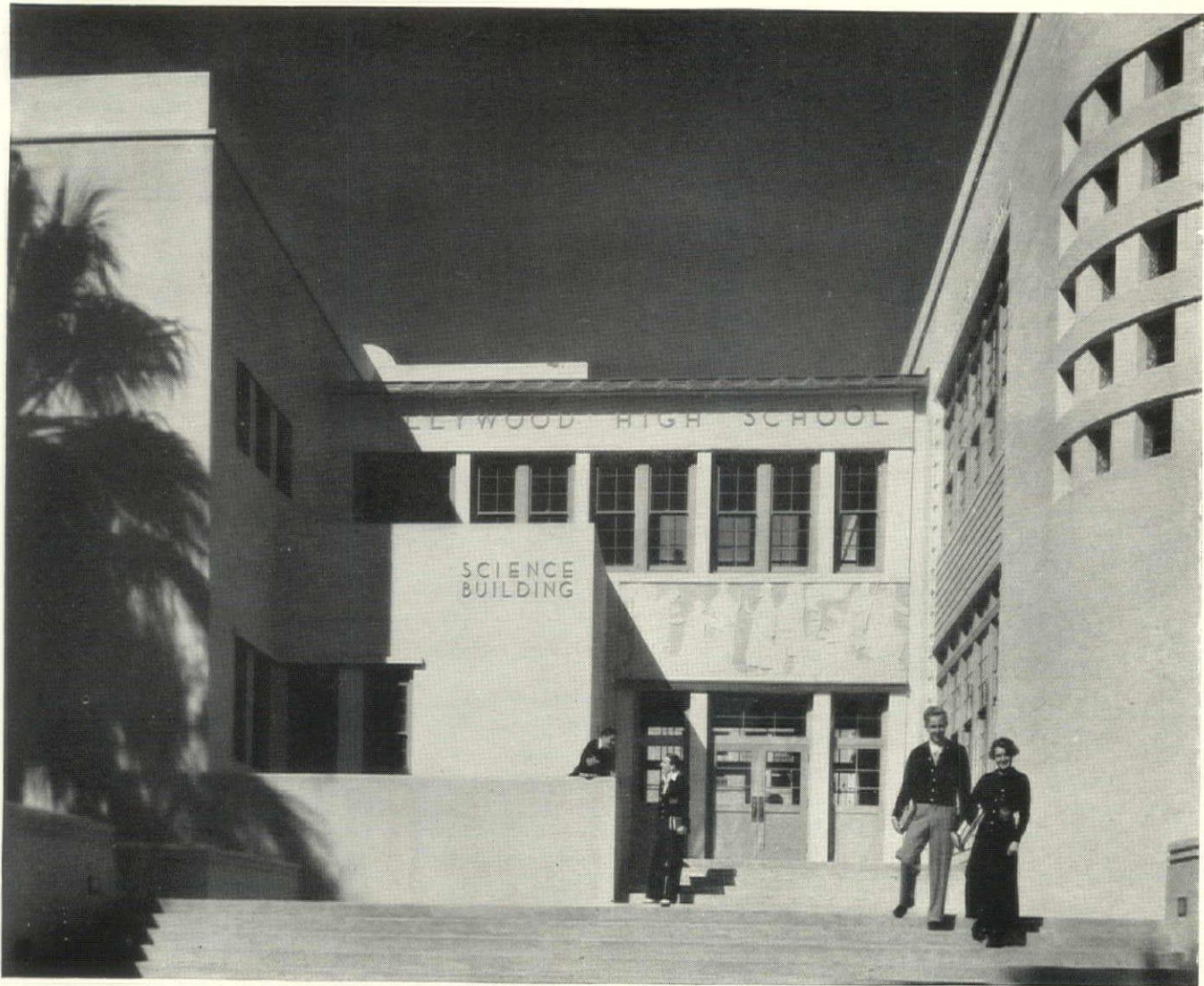
Science Building for Hollywood High School. Marsh, Smith & Powell, architects; R. H. Annin, supervising engineer; Sarver and Zoss, contractors—all of Los Angeles. Frame, walls and floors, as well as sculptured panel, grilles and other detail cast integrally in concrete of rigidly-controlled quality.
