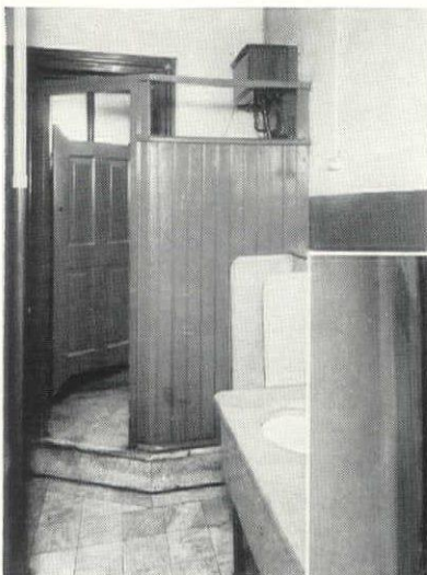
LEFT: Old-fashioned lavatory before remodeling.
