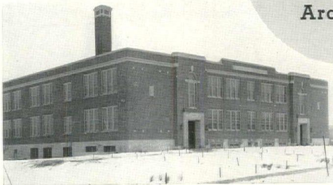
● Genuine wrought iron specified in John Van Duyn School for hot and cold and drinking water and inside supply lines; fire lines; and waste lines, vents, and drains 2" and under.
