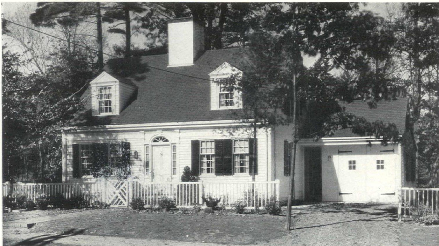
HOUSE OF MRS. HARRIET F. WOOD, STONEHAM, MASSACHUSETTS
