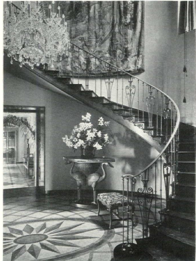
House, Middletown, R. I. Harrie T. Lindeberg
