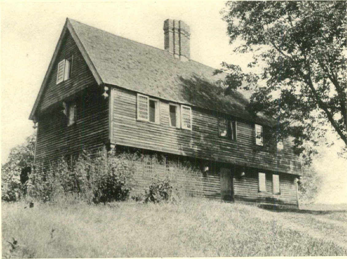
The Parson Capen House in Topsfield, Massachusetts, was built in 1683
