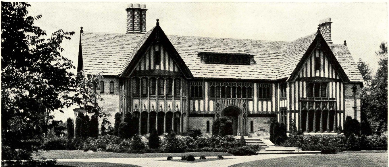
In the residence of Mr. Oscar Webber, 619 Lake Shore Drive, Detroit, Michigan, complete telephone convenience is provided by fourteen telephone outlets, including two in the garage and one on the third floor. Built-in conduit carries the wiring for the telephone system which includes intercommunicating setaures. LEONARD WILLEKE, Architect, Detroit.
