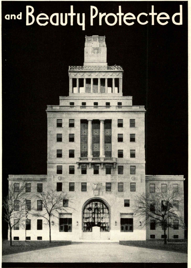
Memorial Building and City Hall, Cedar Rapids, Iowa. Henry Hornbostel, Pittsburgh, Pa., architect, and W. J. Brown and Harry Hunter, Cedar Rapids, associate architects; O. F. Paulson Construction Co., Cedar Rapids, general contractor. Atlas White used for pointing, setting and backing limestone.
