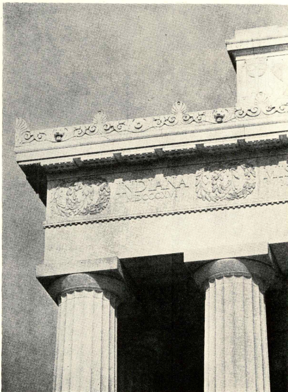
Detail of entablature, Lincoln Memorial, Henry Bacon, architect. From "Masterpieces of Architecture in the United States"
