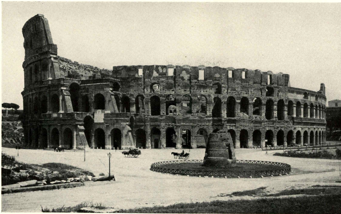
A new architecture that met the needs of its times is evident in the Colosseum. This magnificent amphitheatre utilized the idea, new in A. D. 80, of the round arch, a radical and progressive departure from the column and lintel of the earlier Greek construction
