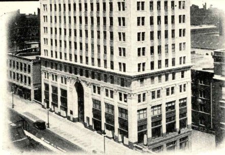
Bell Building Chicago, Illinois
