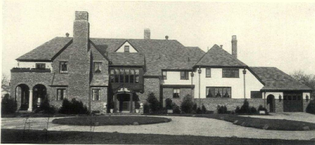
*On the estate of Mr. Monroe Eisner, Red Bank, N. J., are fourteen telephone outlets: eleven in the residence, and one each in the superintendent's cottage, the stables and a detached garage. Built-in conduit connects these outlets and carries the wiring for the telephone system which includes intercommunicating features. The dining-room and breakfast-room outlets are served with a portable telephone.*
