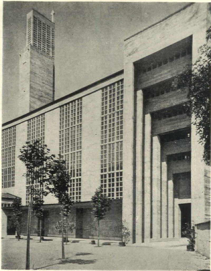
The utilization of modern construction results in a delicacy of form through the replacement of the massiveness of stone with glass and concrete
