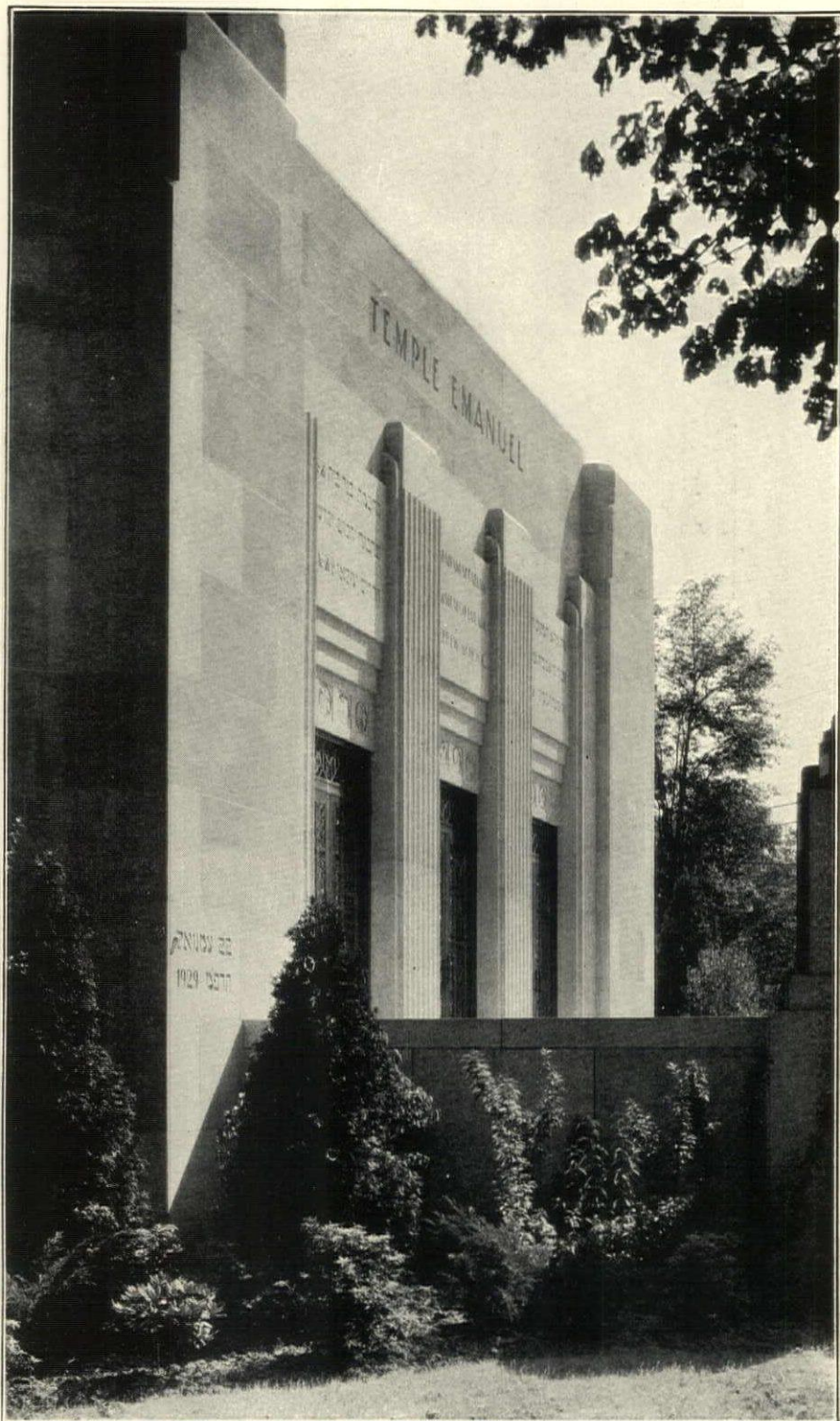
Temple Emanuel, Paterson, New Jersey. F. W. Wentworth, Architect. J. W. Ferguson Company, Builders.
