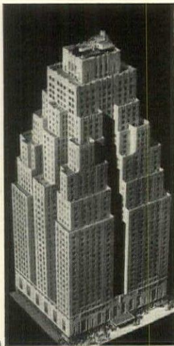
Sugarman and Berger Architects Wm. Bradley & Son Marble Contractor
