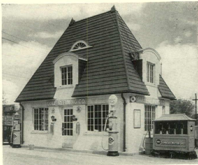
Dark green aluminum shingles used on the filling station of the Gulf Refining Co. at Lawndale, Pa. E. J. Krepley, architect
