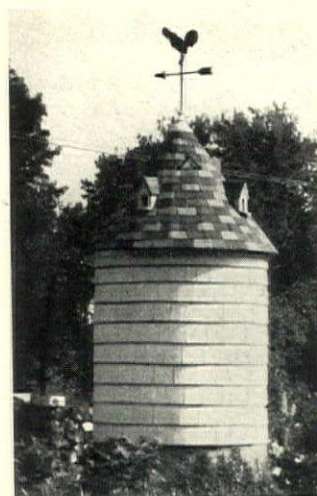
The oil supply tank was put on end above grade and enclosed with a structure covered with white shingles that matched the house itself
