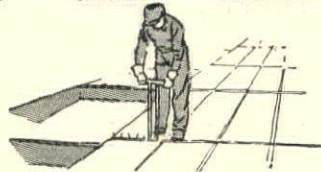
Tying the reinforcement
