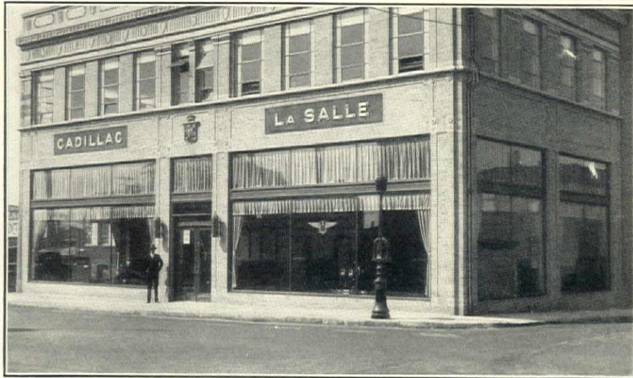
Desco Store Fronts installed in Cadillac-La Salle Showroom, Jersey City, N. J. Chas. G. Eicholz, Jr., Architect. James Billington & Sons, Inc., Builders
