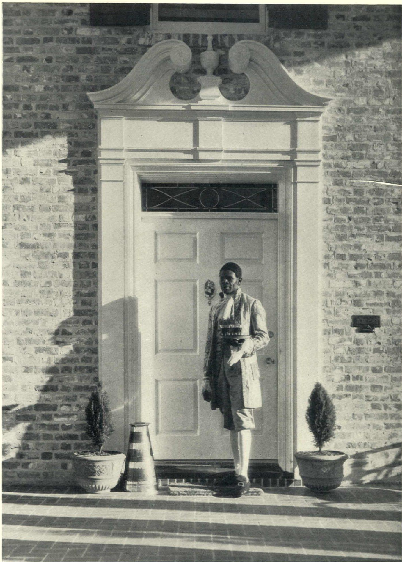
Refinement in mouldings, combined in a dignified composition, offers a pleasing contrast in color, texture, and scale to rough brick. The above doorway of Georgian inspiration in the entrance of the T. J. Bettes house, Houston, Texas; Charles W. Oliver, architect
