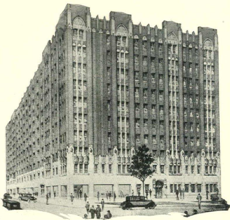
The 4425 Sheridan Apartments at Sheridan Rd. and Galt St., Chicago. Architect: Roy F. France & Co. Chicago, Ill. Consulting Engineer: Arthur S. Grossberg, Chicago, Ill. Heating Contractors: Schampel & Dougherty, Inc., Chicago, Ill.
