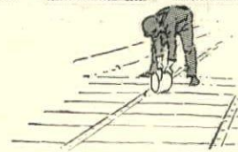
Grouting the joints between slabs
