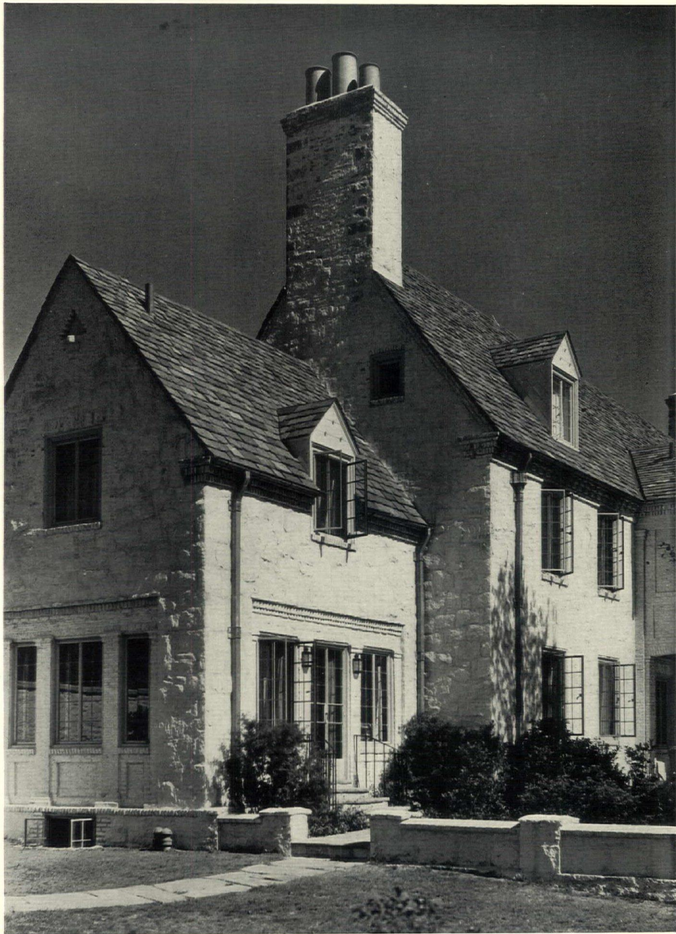
Local stone and brick have been combined in an interesting manner. No one can accuse the architect of having copied a house several centuries old. The colonial spirit that is evident satisfied the client's desire for a house that would provide a correct setting for his collection of some very fine specimens of seventeenth century English furniture
