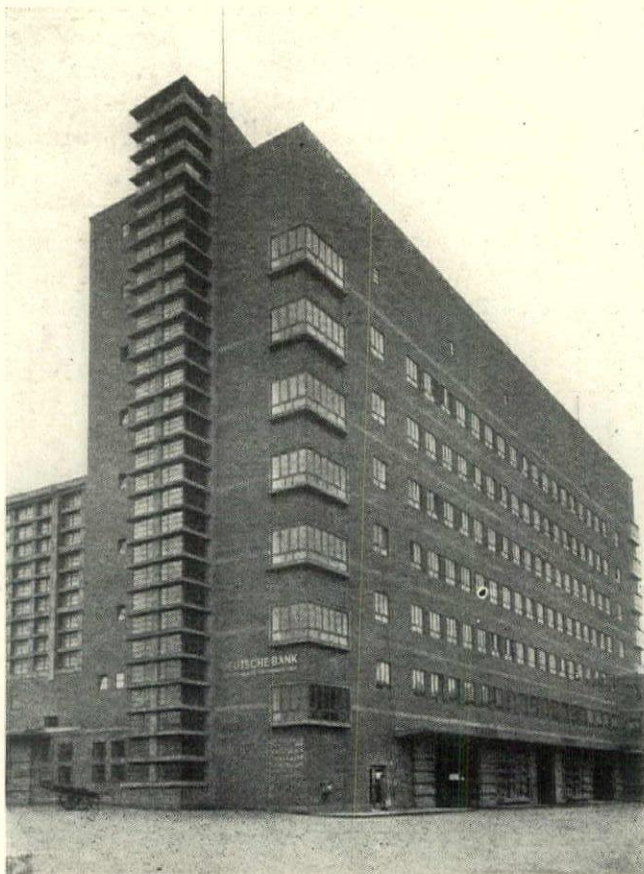
The administration block of the Frankfurt Market. On the left side is the elevator shaft of concrete and glass. Professor Elsaesser, architect. From the Architect and Building News, October 4, 1929
