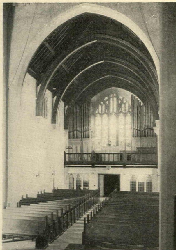
EARLY ENGLISH FORM OF HAMMER-BEAM TRUSSES USED IN THE FIRST BAPTIST CHURCH, CHICAGO, ILL.
