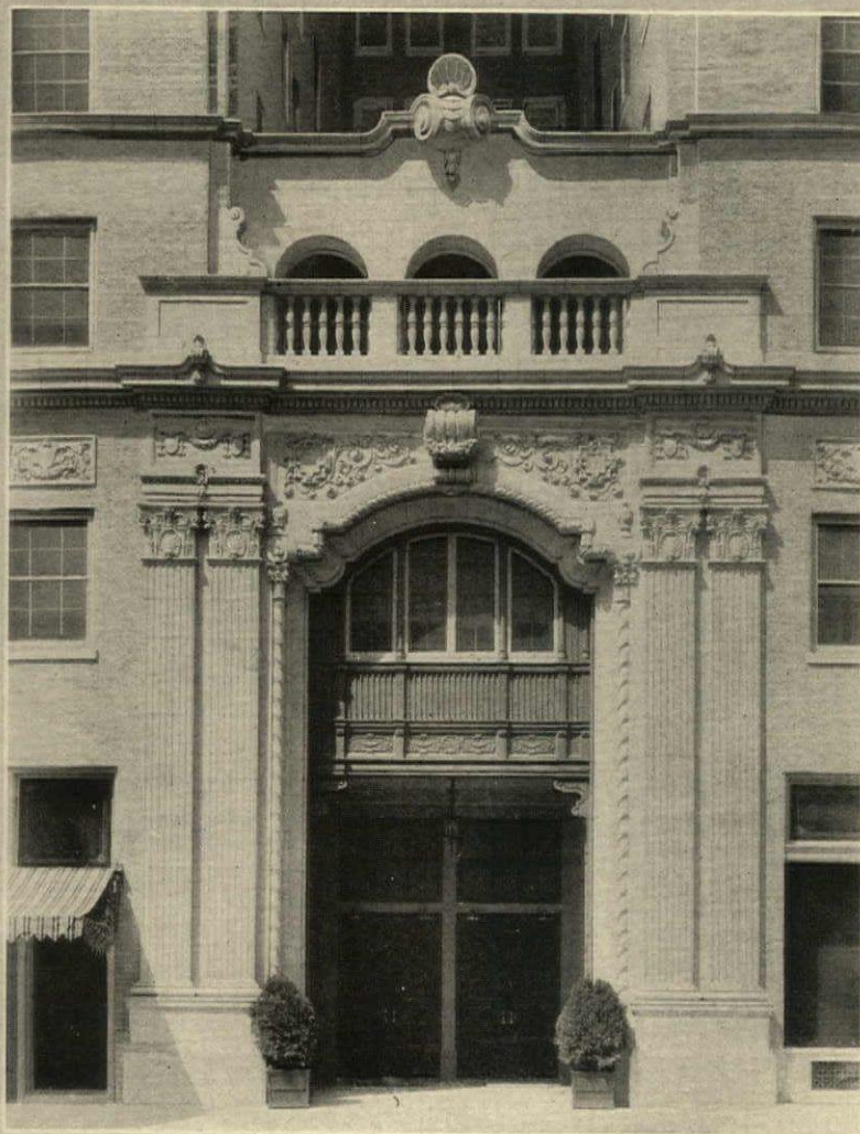
Harwood Street Entrance, Hilton Hotel, Dallas, Texas, Lang & Witchell, Architects, An effective and beautiful use of Terra Cotta with graceful clear cut detail.
