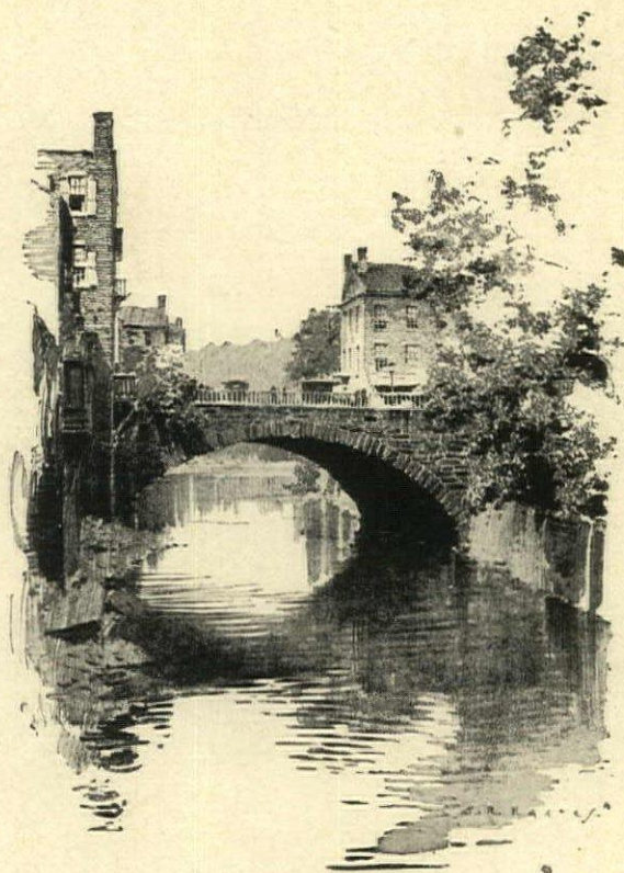
Street Bridge, Hartford, Conn.
