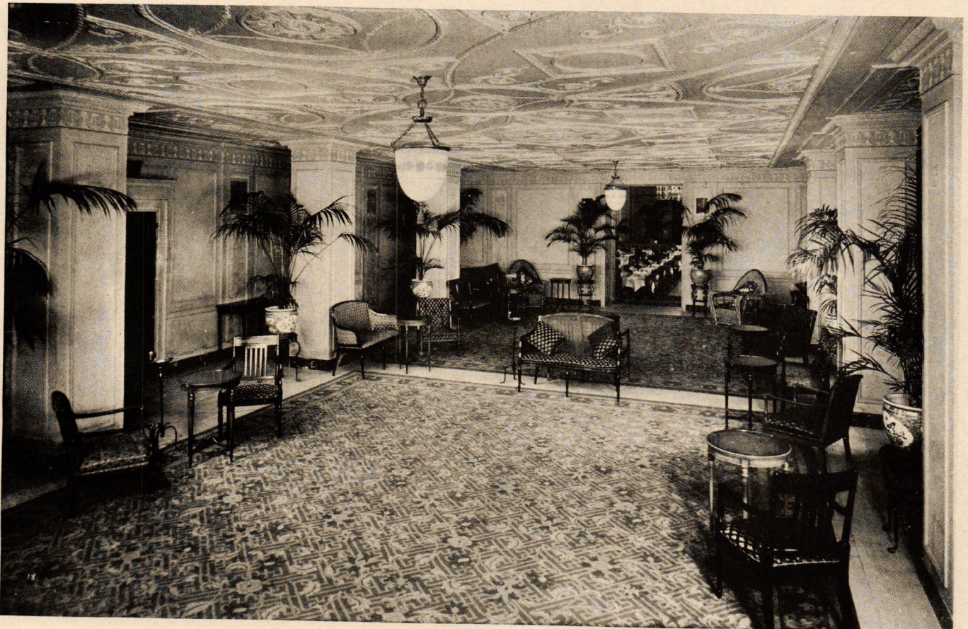
FOYER TO MAIN DINING ROOM ATLANTA-BILTMORE HOTEL, ATLANTA, GA. SCHULTZE & WEAVER, ARCHITECTS
