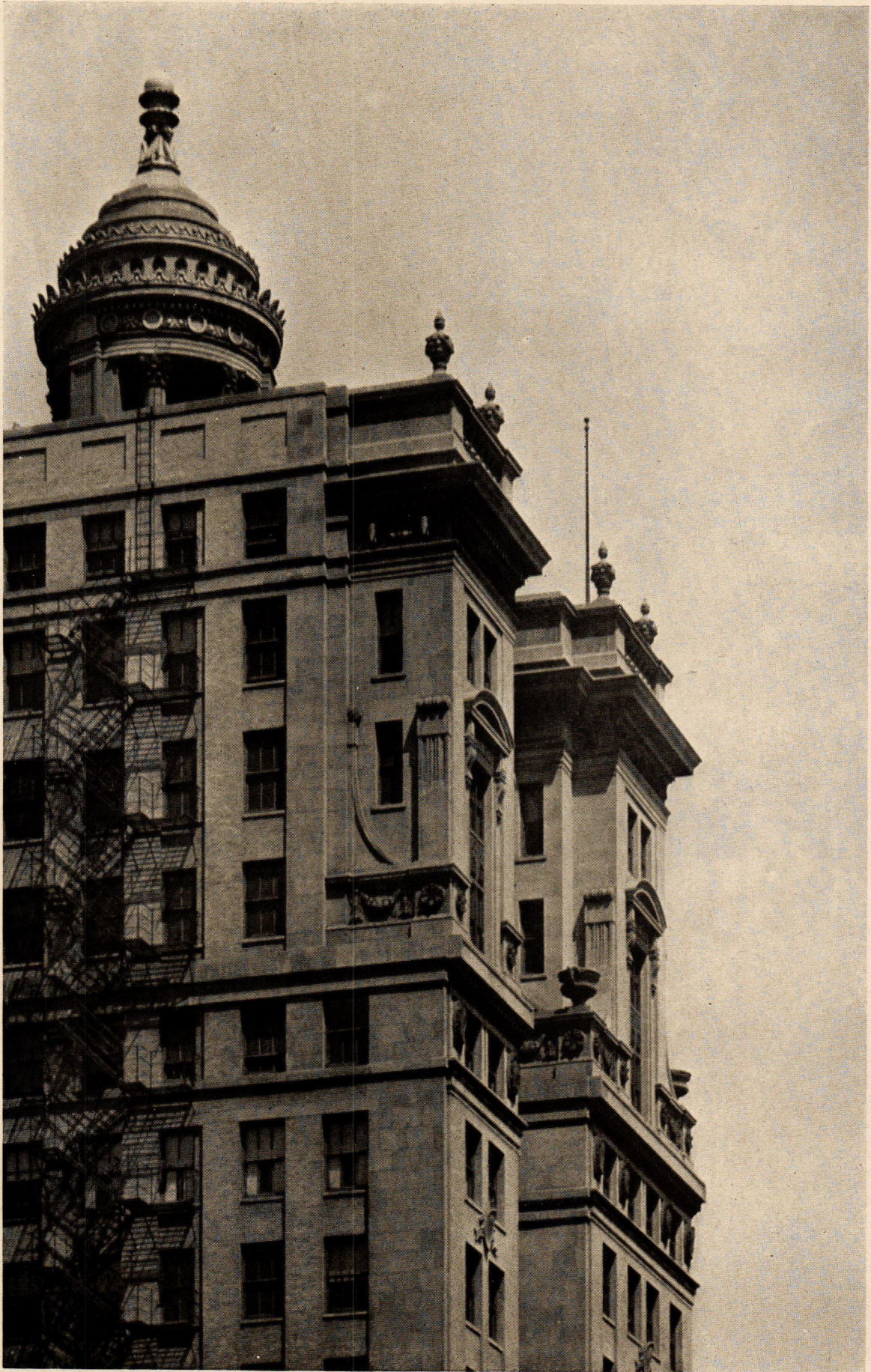
DETAIL OF UPPER STORIES ON MICHIGAN AVENUE LONDON GUARANTEE AND ACCIDENT BUILDING, CHICAGO, ILL.
