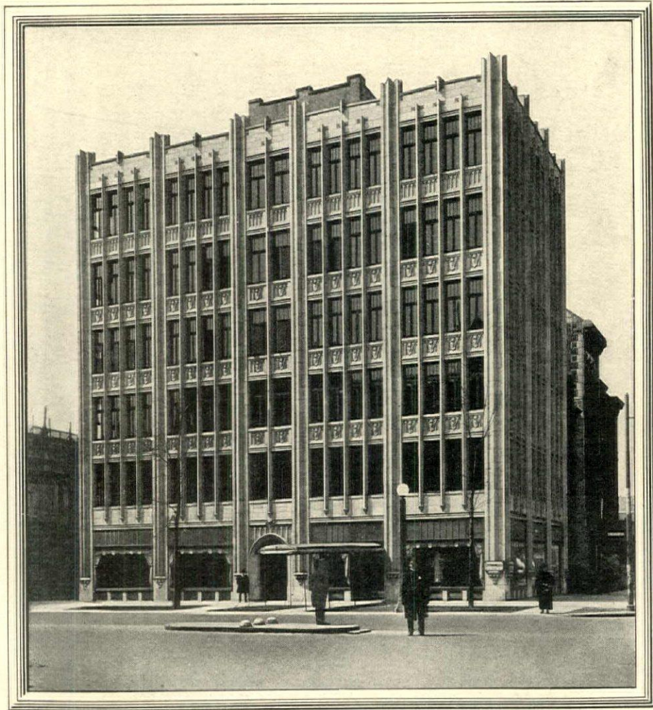
Building at Michigan and Chicago Avenues, Chicago — Entire Facing of Cast Stone Robert T. Newberry, Chicago, Ill., Architect. Ridenour & Erickson, Chicago, Contractor
