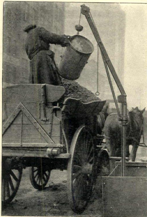
Model D Electric Hoist at Conley Tin Foil Co., New York. Francisco & Jacobus, Archts.
