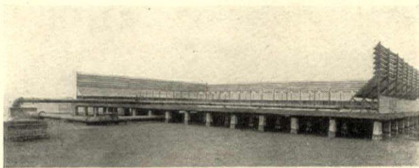
SPRAY POND ON ROOF WHERE WARM WATER FROM AMMONIA CONDENSERS IS COOLED BY BEING SPRAYED INTO THE AIR. LOUVRE FENCE AROUND POND PREVENTS WASTE OF WATER BY WIND
