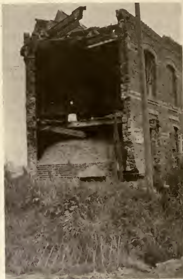
A “PILL BOX” BUILT THREE FEET THICK
