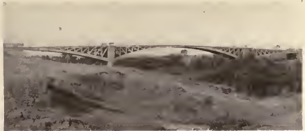
BRIDGE OF REINFORCED CONCRETE, CONSTRUCTED BY THE DIVISION OF HIGHWAYS
