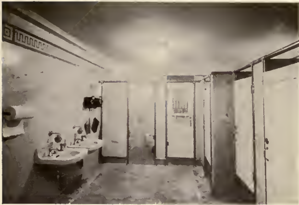
INTERIOR VIEW, PUBLIC CONVENIENCE STATION AT SCRANTON, PA.
