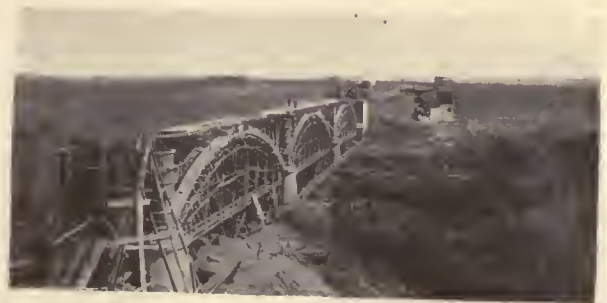
CONSTRUCTION OF CONCRETE BRIDGE
