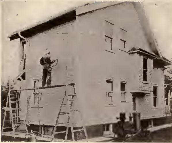
SPRAYING METHOD APPLIED TO SPRING HOUSE PAINTING
