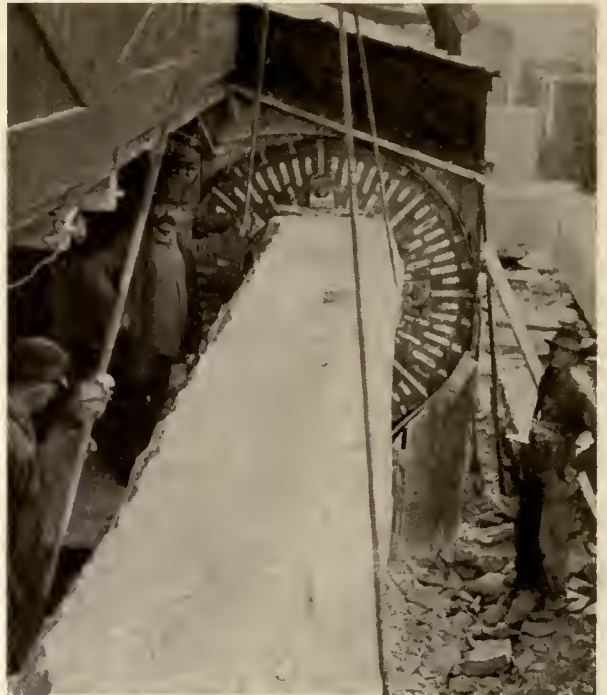
PLACING STONE IN LATHE FROM WHICH MONOLITHIC COLUMN IS TO BE TURNED
