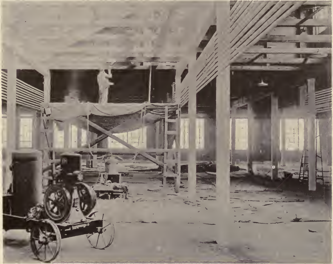
SPRAY PAINTING A FACTORY CEILING
