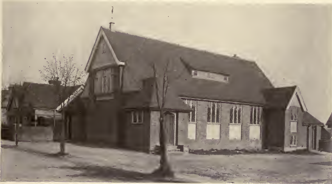
BRANTHAM VILLAGE HALL, NEAR MANNINGTREE, ESSEX, ENGLAND MESSRS. SEARLE & SEARLE, ARCHITECTS
