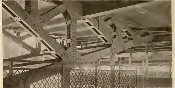
CANTILEVER TRUSSES SUPPORTING CONNECTING ROADWAY, HANGING BRIDGE BELOW TRACKS ALSO VISIBLE
