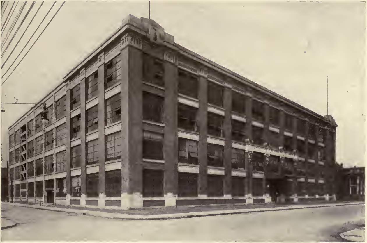
KAHN TAILORING COMPANY BUILDING, INDIANAPOLIS. VONNEGUT, BOHN & MUELLER, ARCHITECTS DOUBLE STAIR EXIT SHOWN ON SIDE ELEVATION
