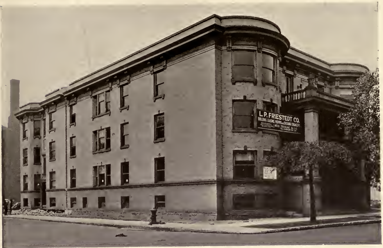
BUILDING IN ORIGINAL POSITION, SECTION 2 FACING JACKSON BOULEVARD, SECTION 1 IN REAR FACING IRVING AVENUE. NOTE THE CUT IN SIDE WALL DIVIDING THE TWO SECTIONS. CRANE TECHNICAL HIGH SCHOOL IN REAR.
