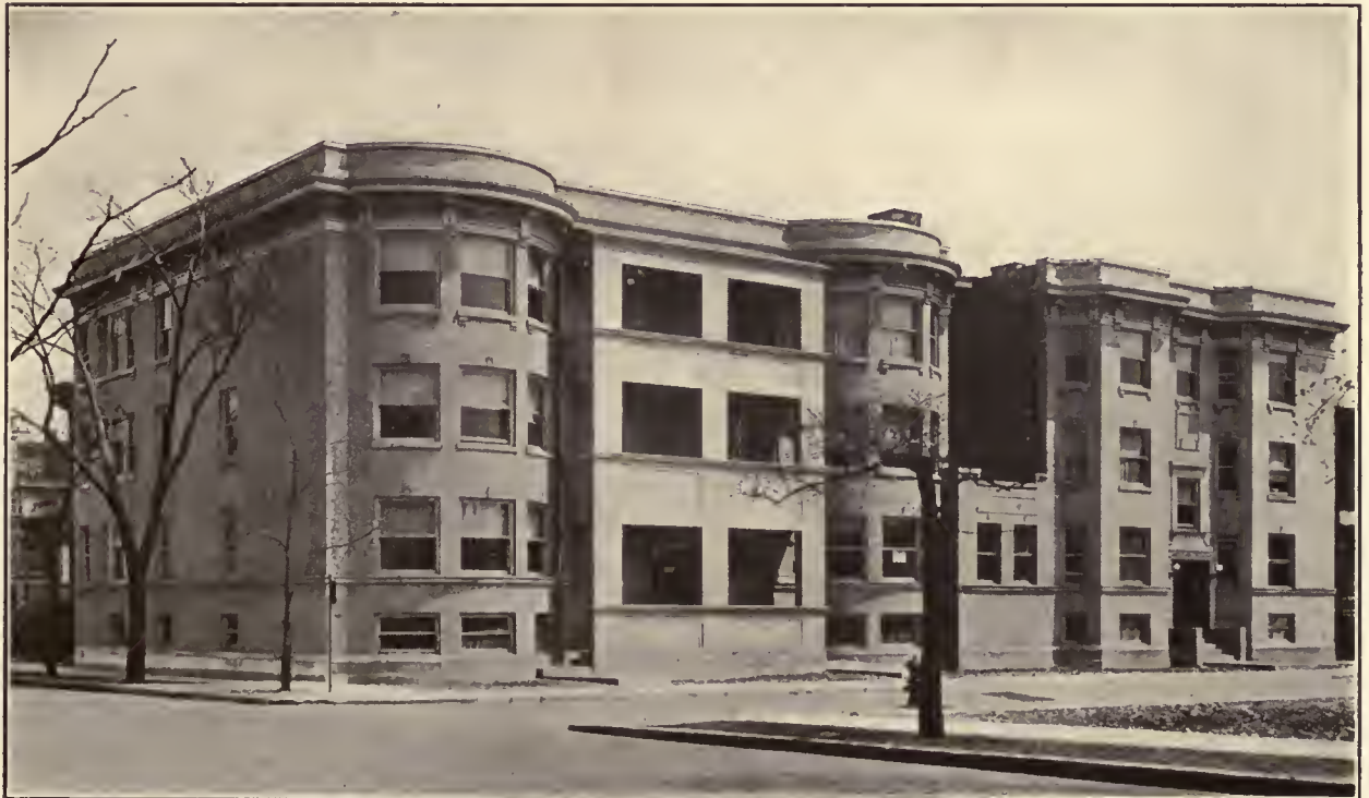
SECTION 1 AT RIGHT, SECTION 2 AT LEFT. BOTH IN FINAL POSITION ON EAST SIDE OF IRVING AVENUE, FACING WEST. THE SECTIONS ARE NOT JOINED EXCEPT BY A ONE STORY STRUCTURE AS SHOWN.
