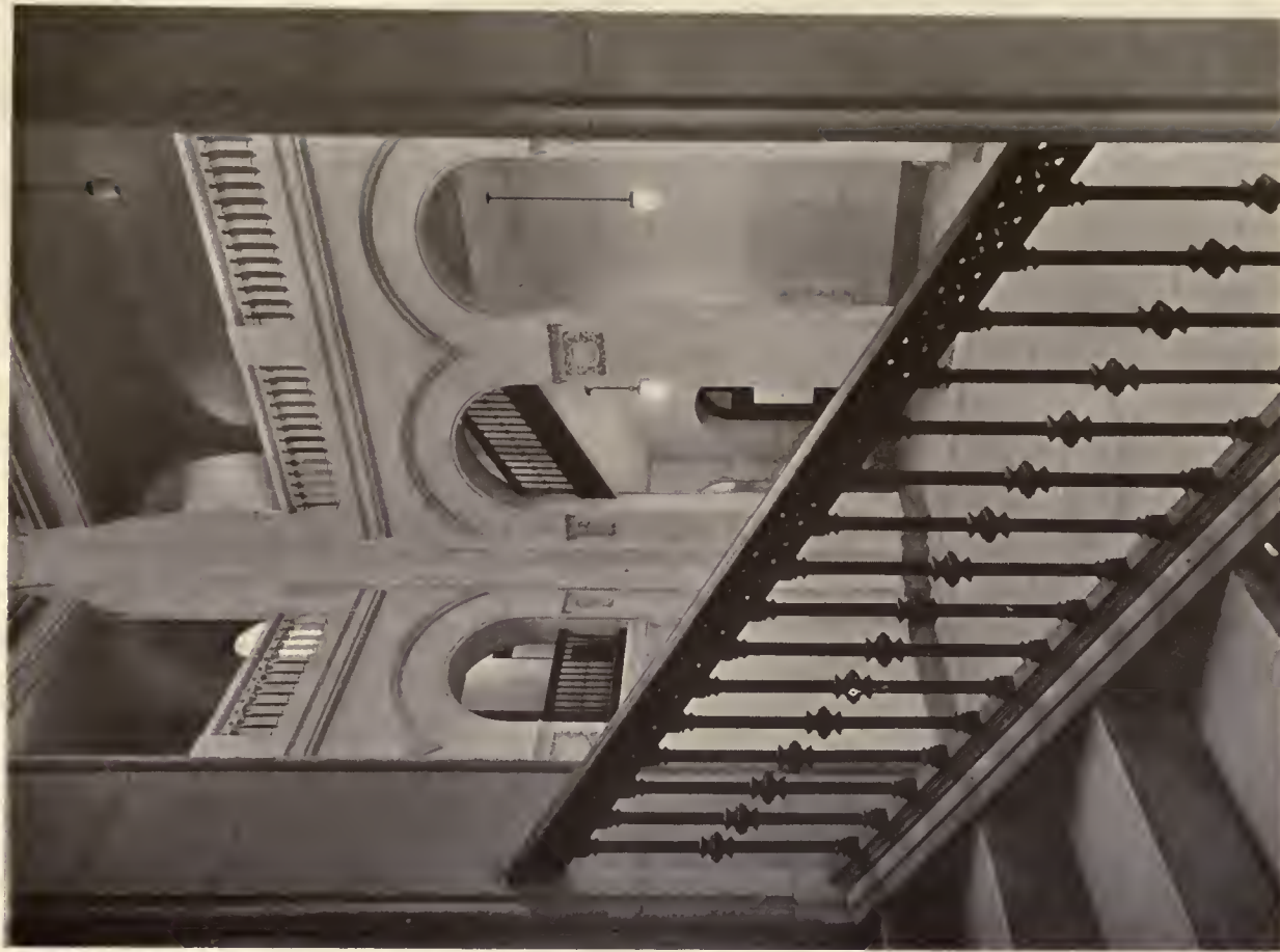
NEW VIEW FROM MAIN STAIRWAY LOOKING INTO LIGHT WELL
