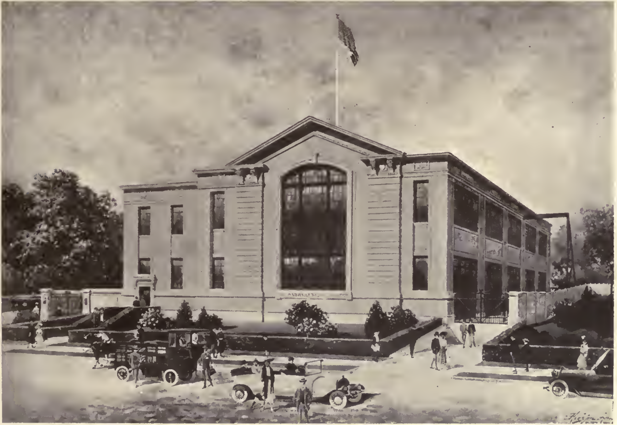
SUB-STATION AT FLUSHING, L. I., BUILT FOR NEW YORK & QUEENS ELECTRIC LIGHT & POWER CO. WILLIAM W. KNOWLES, ARCHITECT
