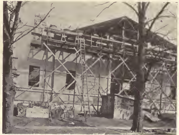
NO. 4. THREE MONTHS LATER. FLOOR AND ROOF ARCHES COMPLETED. WALLS NEARLY TOPPED OUT
