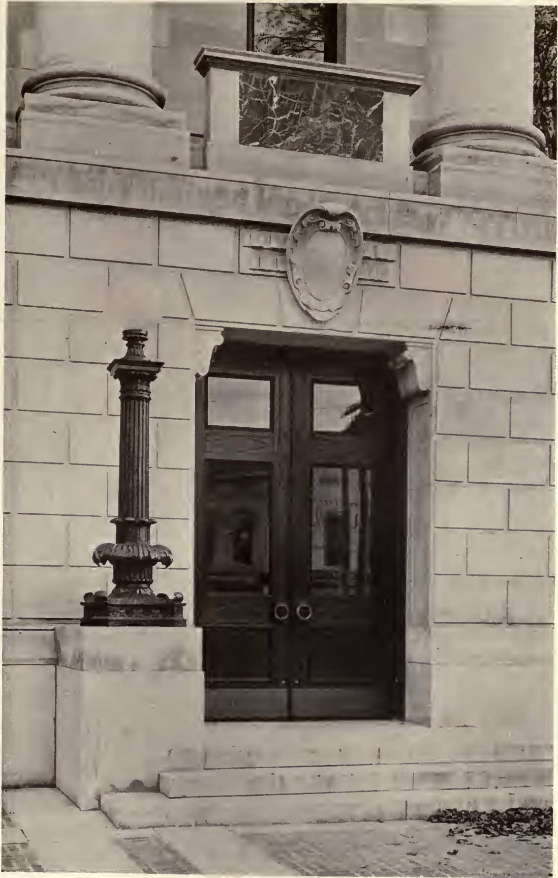
A MAIN ENTRANCE, NORTH ELEVATION PREBLE COUNTY COURT HOUSE, EATON, OHIO H. H. HIESTAND AND RICHARDS, McCARTY & BULFORD, ASSOCIATED ARCHITECTS
