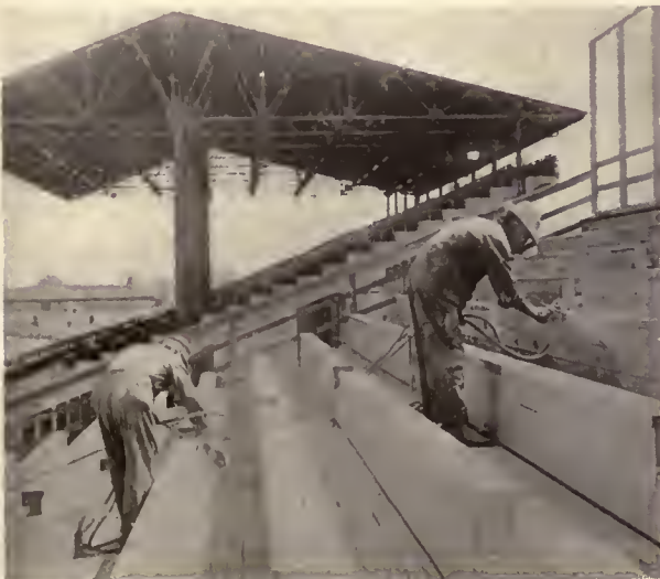
PROLONGING THE LIFE OF THE "BLEACHERS" BY SPRAY PAINTING
