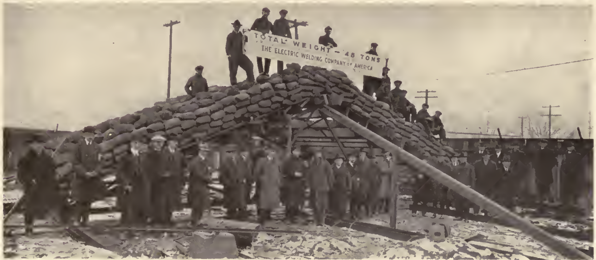
TWO ELECTRICALLY ARC WELDED TRUSSES SUPPORTING A 50 PER CENT OVERLOAD
