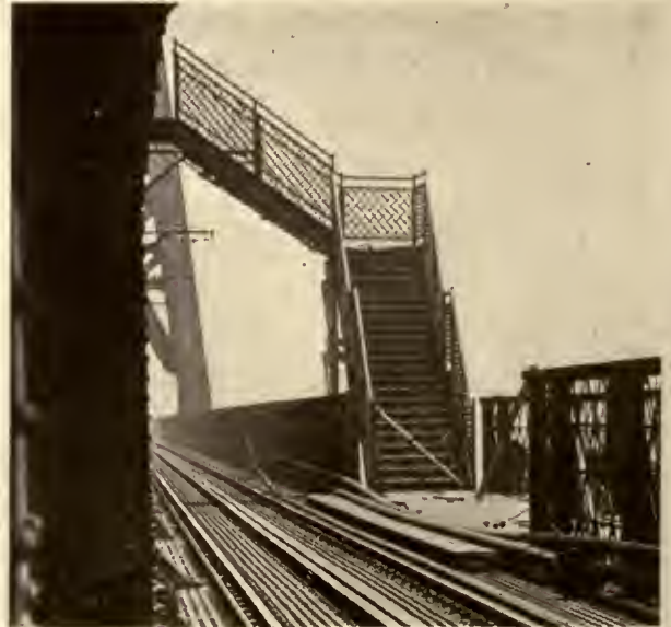
STAIRWAY ON SOUTHERLY SIDE FROM PROMENADE LEVEL, AND CONNECTING WITH HANGING BRIDGE BELOW TRACK LEVEL, BY WHICH ACCESS TO BUILDING IS HAD
