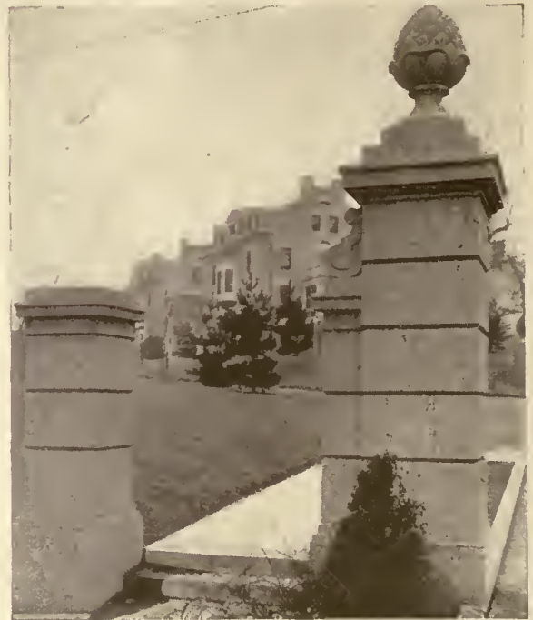
FIG. 7. GATE POSTS AT ENTRANCE TO UNITED STATES NAVAL HOSPITAL, WASHINGTON—AGGREGATE POTOMAC RIVER GRAVEL
