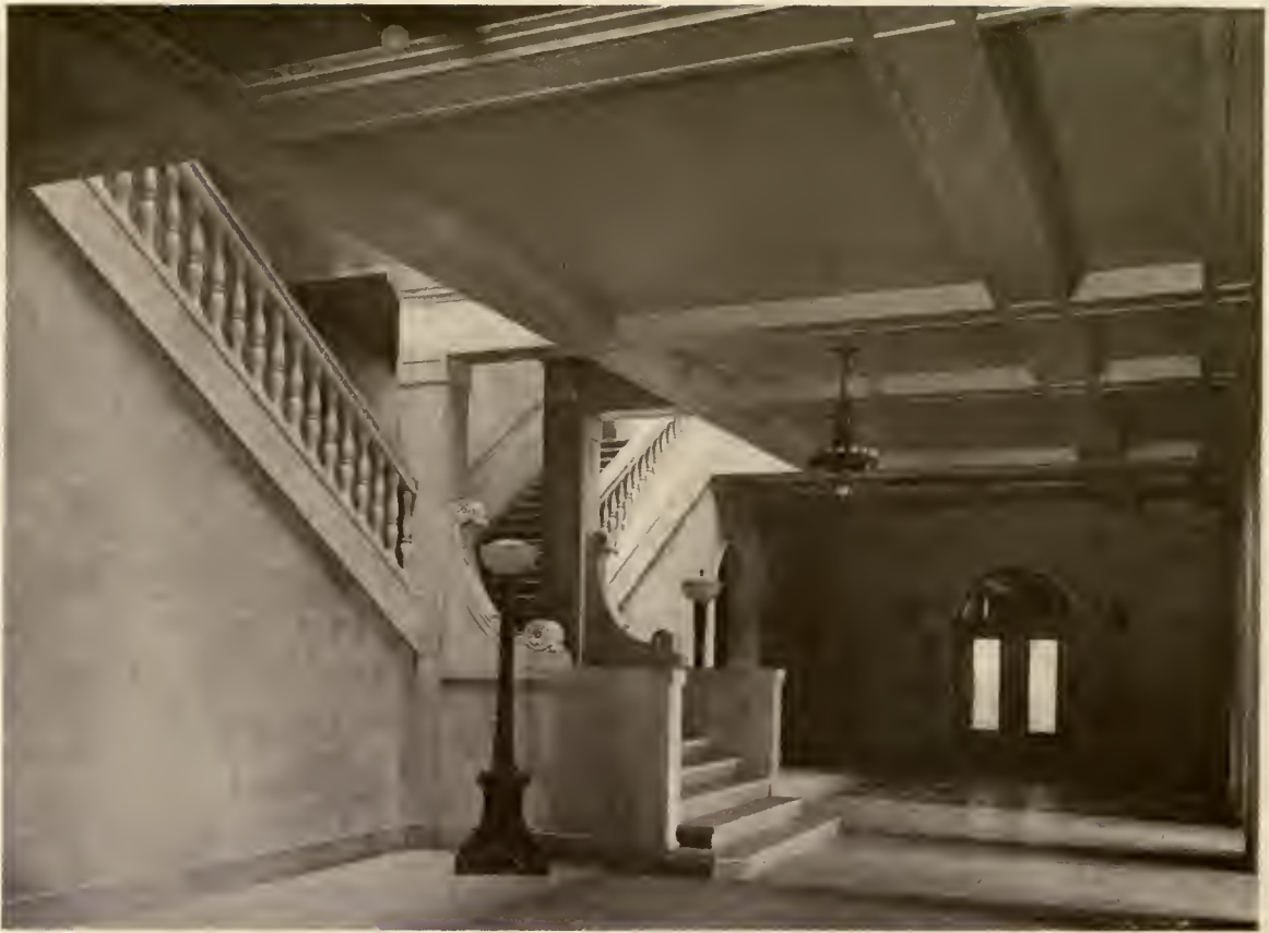
GROUND FLOOR LOBBY, LOOKING SOUTHWEST
