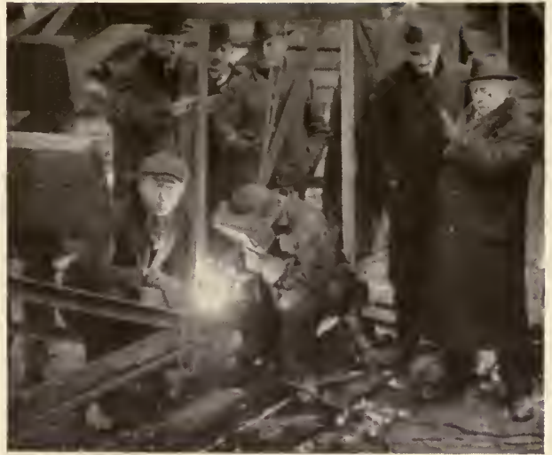
MAKING AN ELECTRIC ARC WELD
