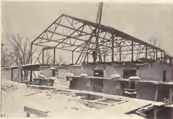
NO. 3. THREE WEEKS LATER. STEEL ERECTION COMPLETED. MASONRY WORK IN PROGRESS
