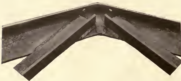
WELDED CONNECTION AT PEAK OF TRUSS
