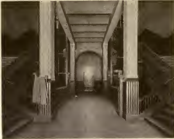
OLD FIRST FLOOR LOBBY
