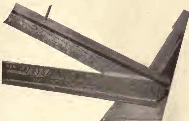
WELDED INTERSECTION OF UPPER AND LOWER TRUSS CHORDS
