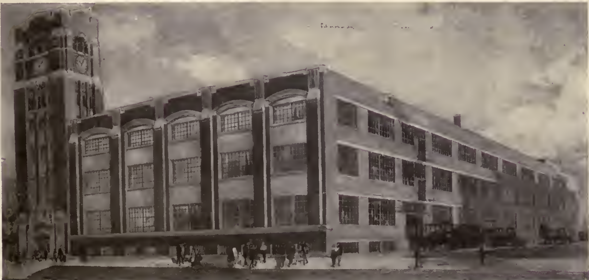
BUILDING FOR THE CONTINENTAL CAN CO., CENTRAL MANUFACTURING DISTRICT, CHICAGO. S. SCOTT JOY, ARCHITECT
