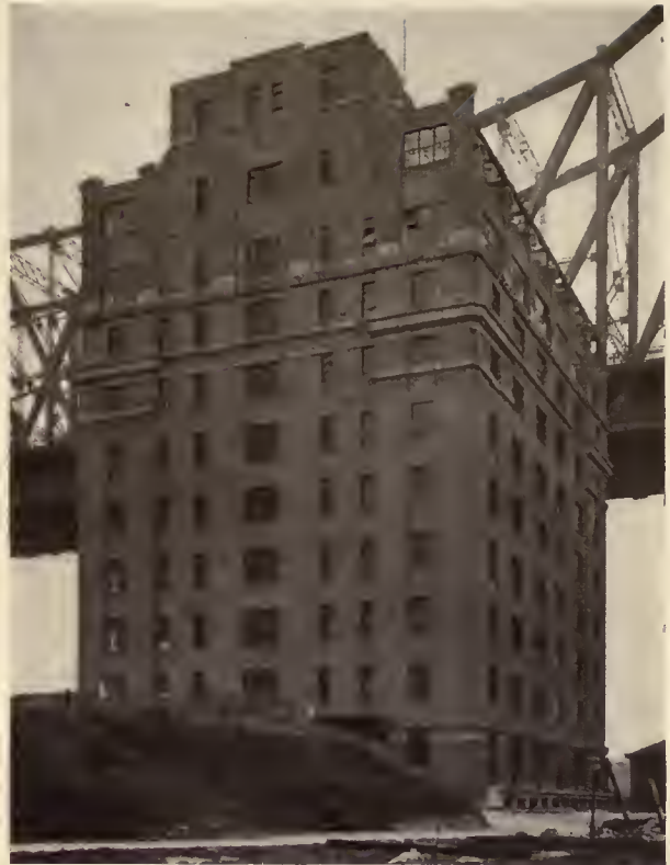
NORTH ELEVATION OF COMPLETED ELEVATOR STOREHOUSE BUILDING, BLACKWELLS ISLAND, N. Y.
