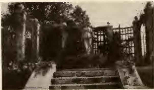
ROSE TRELLIS SUPPORTS—CAST STONE TREATED WITH SULPHATE OF COPPER TO PRODUCE COLOR EFFECT. STATUE BRONZE, TRELLIS WOOD STAINED BROWN, STEPS LOCAL QUARRY STONE. ROSEMONT, PENNA.
