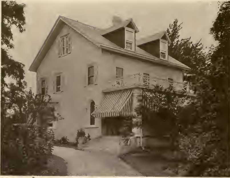
HOUSE OF E. L. COHEN, LARCHMONT, N. Y. MAGNESITE STUCCO ON WOOD LATH; DASH FINISH. A. L. BENNIX, ARCHITECT
