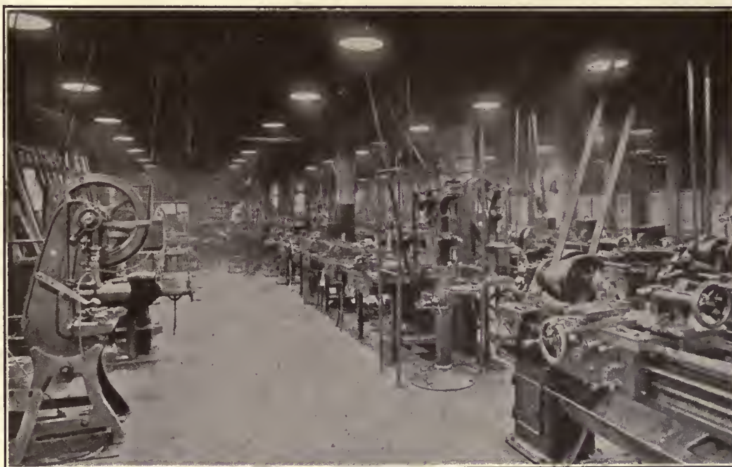
DIRECT LIGHTING IN MACHINE SHOP Note evenness of illumination and absence of sharp shadows
