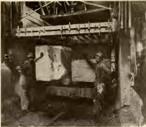
VIEW OF STONE GANG-SAW. ON THE GRATING ABOVE IS PLACED OTTAWA SAND, USED AS AN ABRASIVE, THE SAWS NOT BEING PROVIDED WITH TEETH
