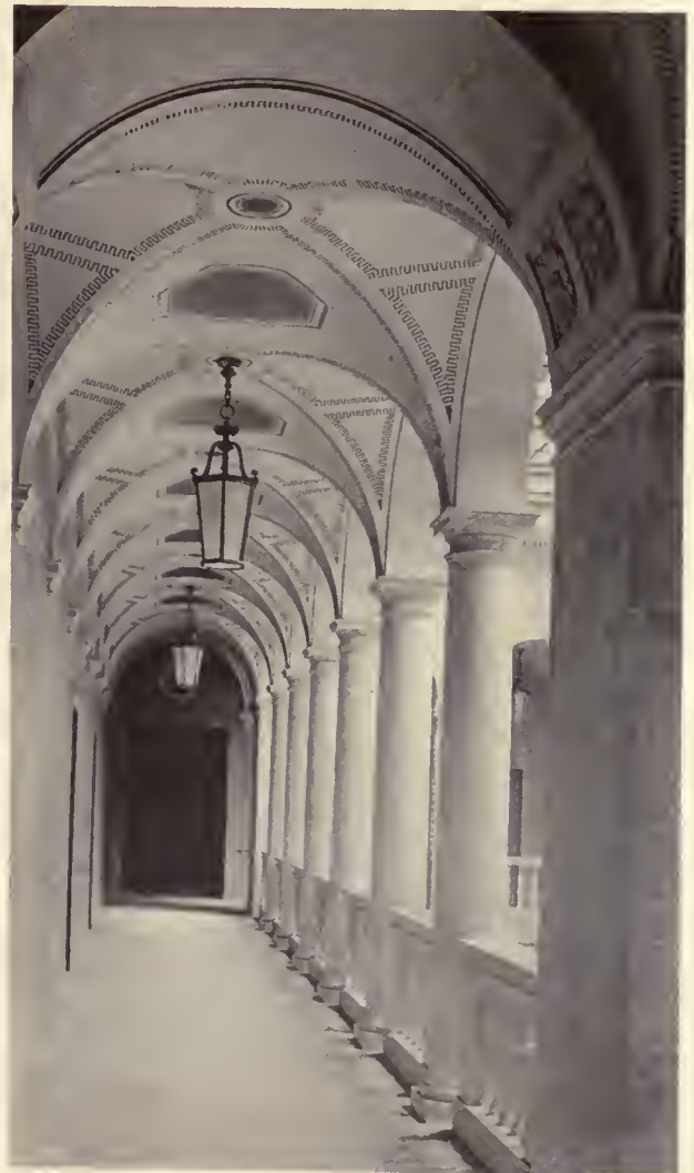
NORTH CORRIDOR, SECOND FLOOR
