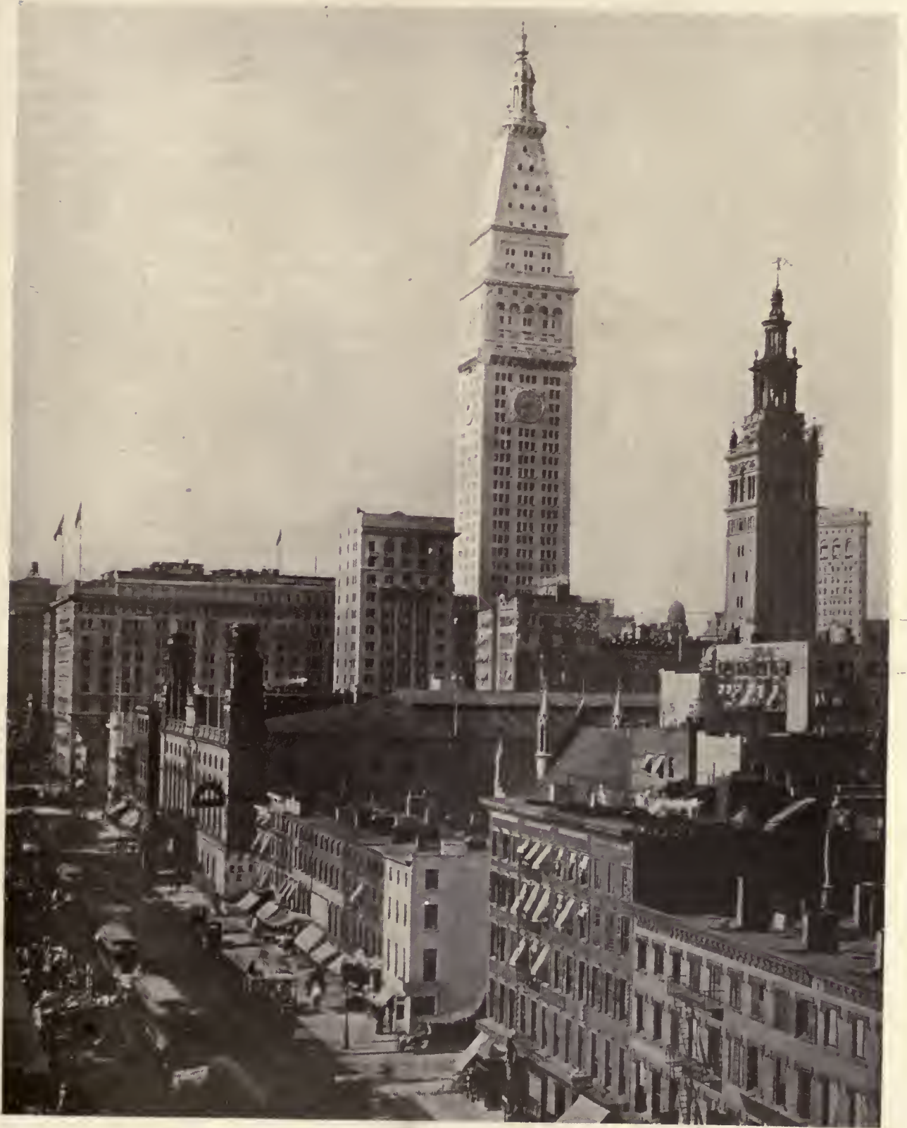
VIEW SHOWING THE METROPOLITAN TOWER, MADISON SQUARE, NEW YORK CITY
