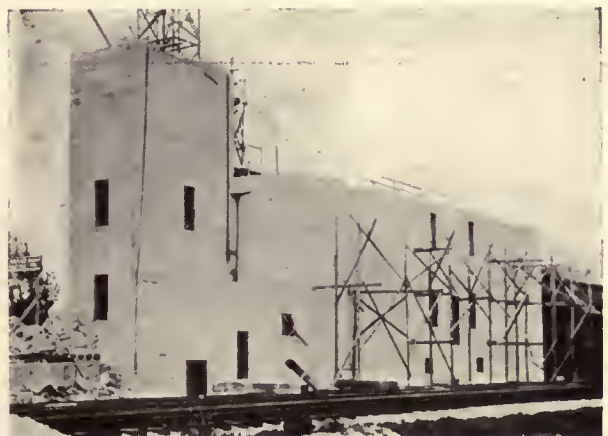
STUCCO WORK PRACTICALLY COMPLETED. LIGHT SCAFFOLD USED BEING TAKEN DOWN
