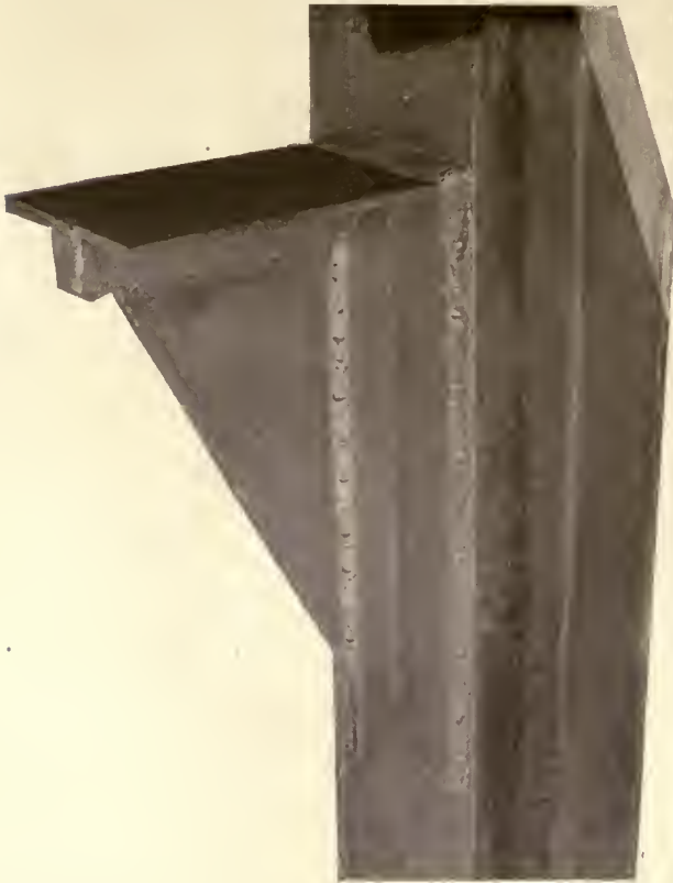
BRACKET SUPPORT FOR 5-TON CRANE RAIL, JOINED TO COLUMN BY ELECTRIC ARC WELDING
