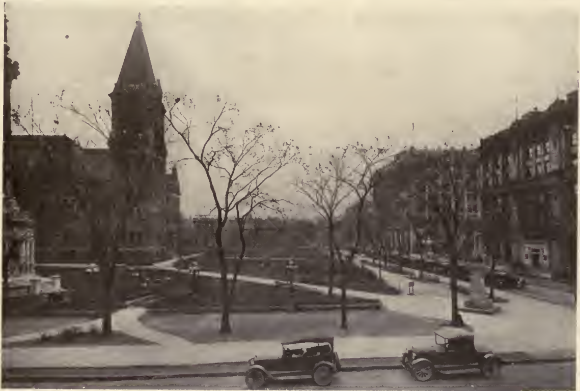
VIEW SHOWING ENTRANCES TO UNDERGROUND CONVENIENCE STATION, SCRANTON, PA. DUCKWORTH BROTHERS, ARCHITECTS Note excellent arrangement of entrance. Stairs to men's and women's section are from different streets. Exhaust for vitiated air disguised as a large flower urn
