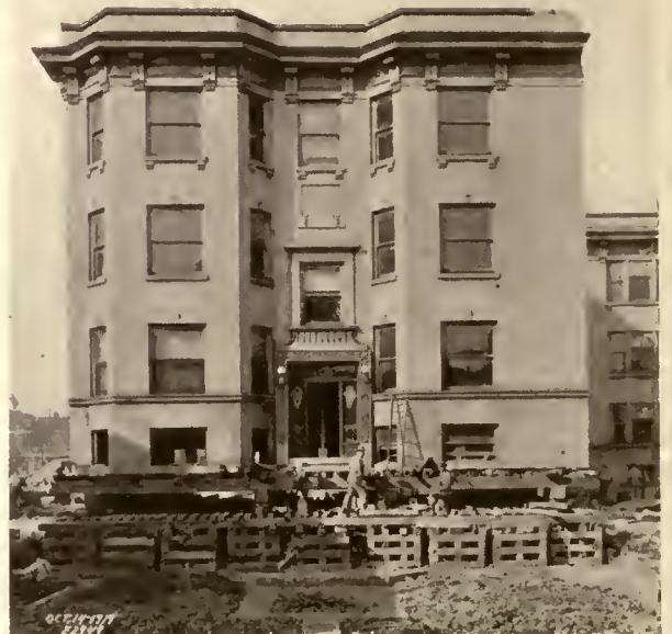
SECTION 1 IN MIDDLE OF IRVING AVENUE AND FACING EAST JUST BEFORE TURNING; SECTION 2 AT RIGHT IN ORIGINAL POSITION
