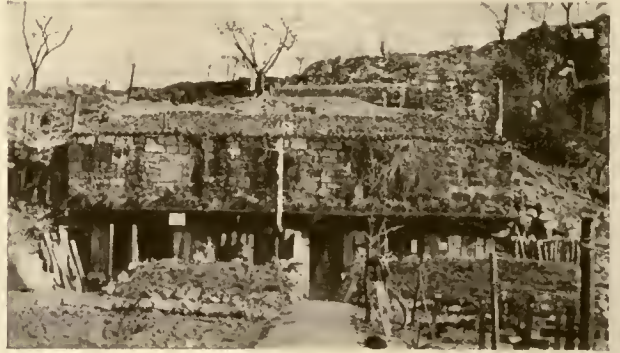
THE FIRST CIVILIAN HOME, AFTER THE ARMISTICE, IN VARENNES-EN-ARGONNE, ONCE A GERMAN DUG-OUT
