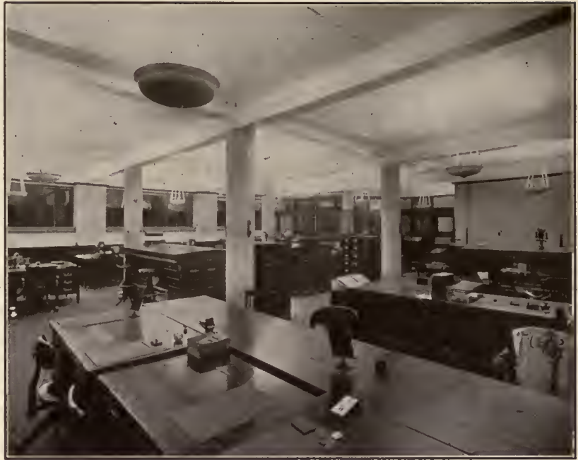
INDIRECT LIGHTING OF OFFICE OF VAN DUSEN HARRINGTON COMPANY, MINNEAPOLIS, MINN
