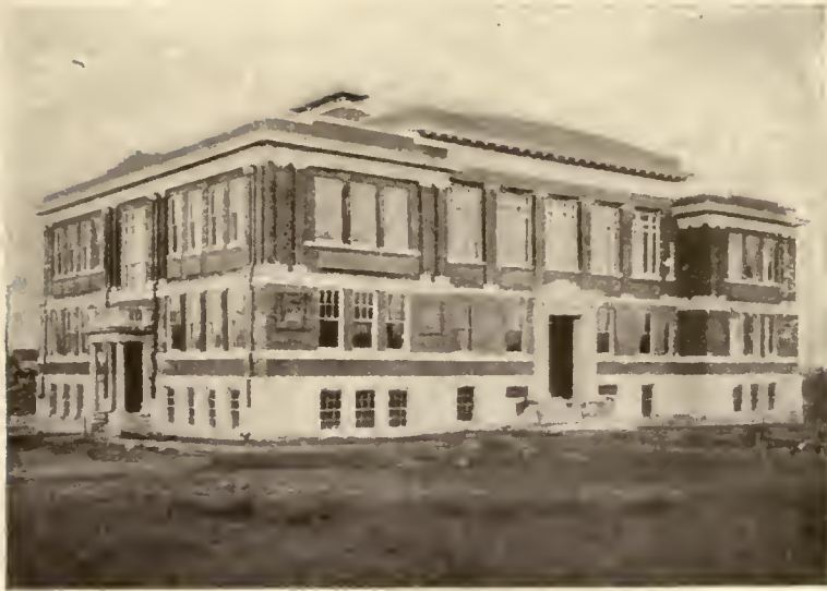
FIG. 8. BRICK AND WOOD-JOISTED SCHOOL BUILDING. SAME PLAN AND COST AS BUILDING SHOWN IN FIG. 9. INTERIOR CONSTRUCTION OF WOOD, WOODEN CORNICES AND CEILINGS OF STAMPED METAL.
