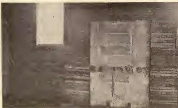
UNLESS THE AIR SPACE IN THE WALL CONSTRUCTION IS CONTINUOUS, INTERIOR PLASTERING SHOULD BE ON LATH FURRED OUT FROM THE FACE OF THE WALL AS SHOWN ABOVE
