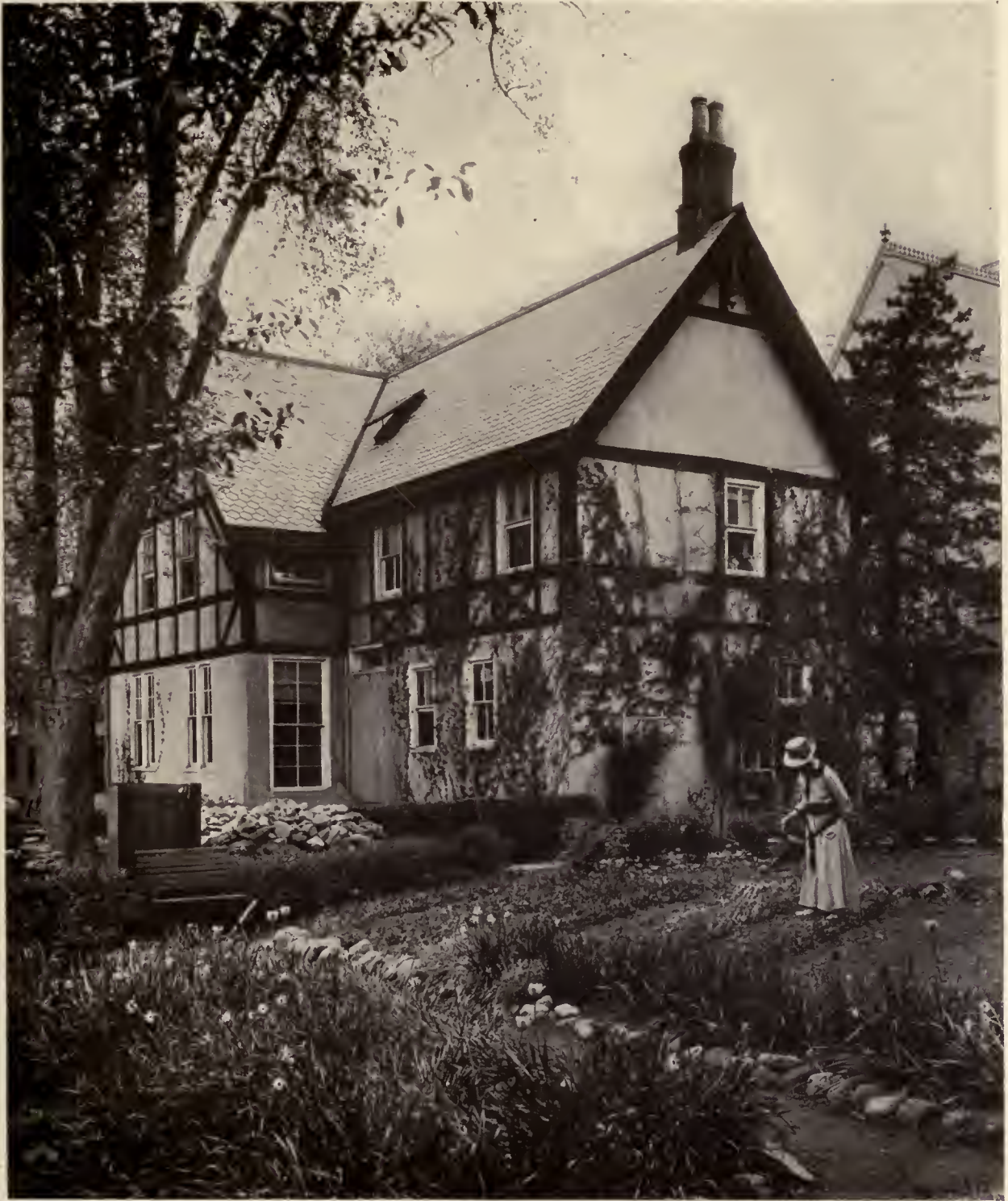
ALTERATIONS TO HOUSE OF EDWARD M. HALE, PASSAIC, N. J. JOHN F. JACKSON, ARCHITECT
