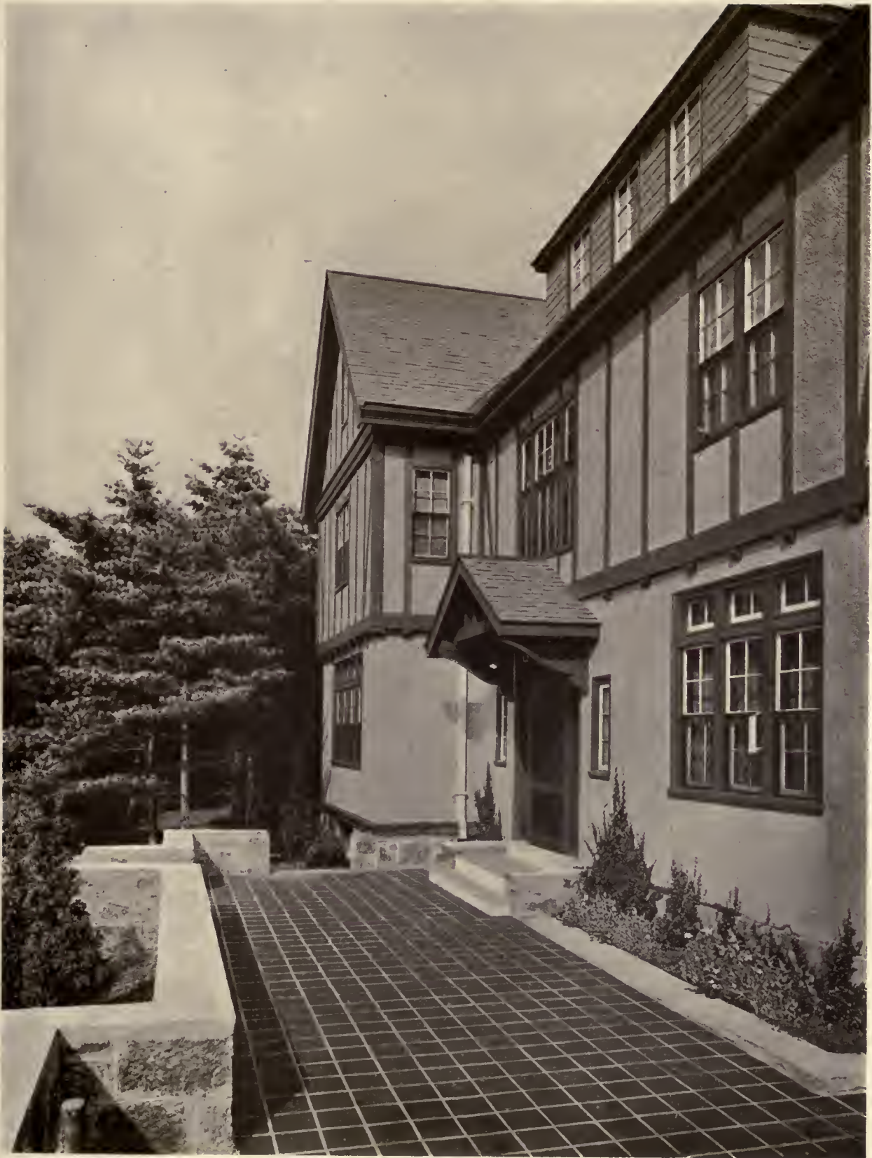
HOUSE OF GEORGE L. OSBORN, BROOKLINE, MASS. JAMES PURDON, ARCHITECT
