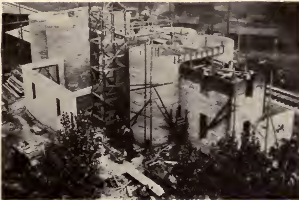
DOUBLE WALLS BUILT IN SUCCESSIVE TIERS
