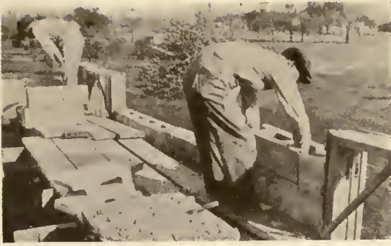
A WALL BEING CONSTRUCTED OF THE USUAL TYPE OF CONCRETE BLOCK
