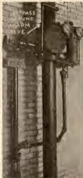
FIG 3. THE ARRANGEMENT OF VALVE HERE SHOWN IS IDENTICAL WITH REGULAR SYSTEM EXCEPT FOR THE BY-PASS.
