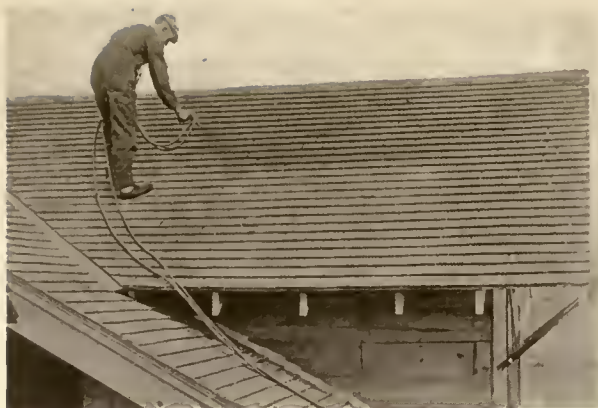
SPRAY PAINTING A SHINGLE ROOF Such surfaces often prove difficult for brush work
