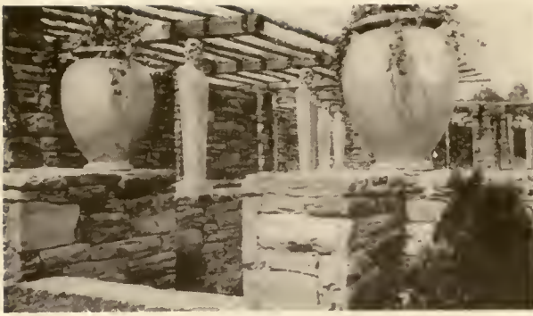
PERGOLA—CAST STONE WITH ROUGH AXED AND BARK COVERED WOOD AND LOCAL QUARRY STONE WALLS. ROSEMONT, PENNA.
