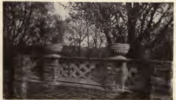
CAST STONE SCREEN AND ORNAMENTS WITH LOCAL QUARRY STONE WALLS. TEXTURE AND COLOR OF SCREEN MADE TO HARMONIZE WITH QUARRY STONE
