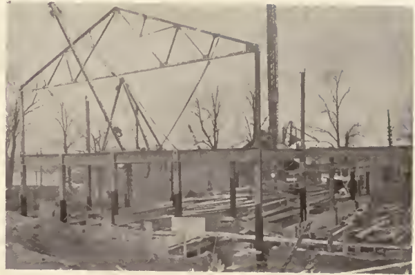
NO. 2. ONE WEEK LATER. STEEL IN COURSE OF ERECTION
