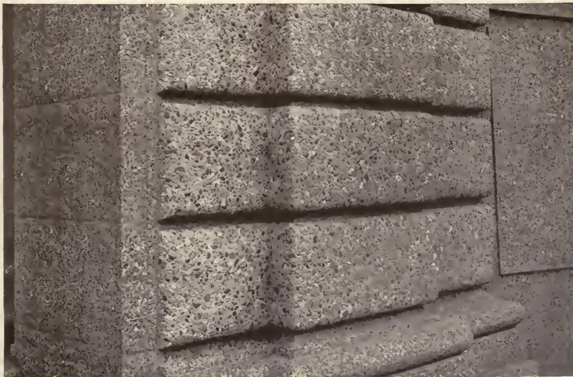
FIG. 5. DETAIL VIEW OF ENTRANCE TO MERIDIAN HILL PARK, WASHINGTON, D. C., SHOWING EXPOSED AGGREGATE SURFACES
