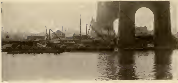
SITE OF STOREHOUSE BUILDING SHOWING COMMENCEMENT OF WORK
