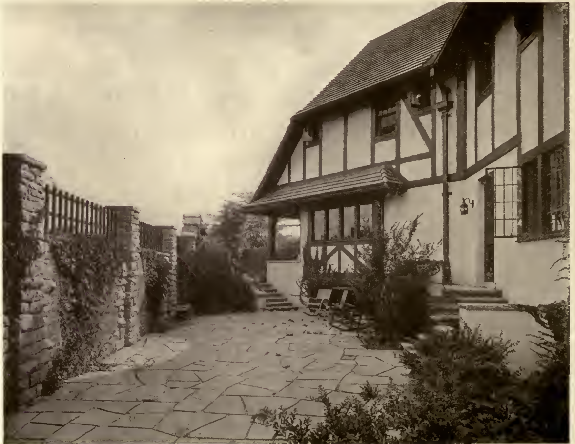
SERVICE COURT ON ESTATE OF WILLIAM S. WALBRIDGE, TOLEDO, O.
