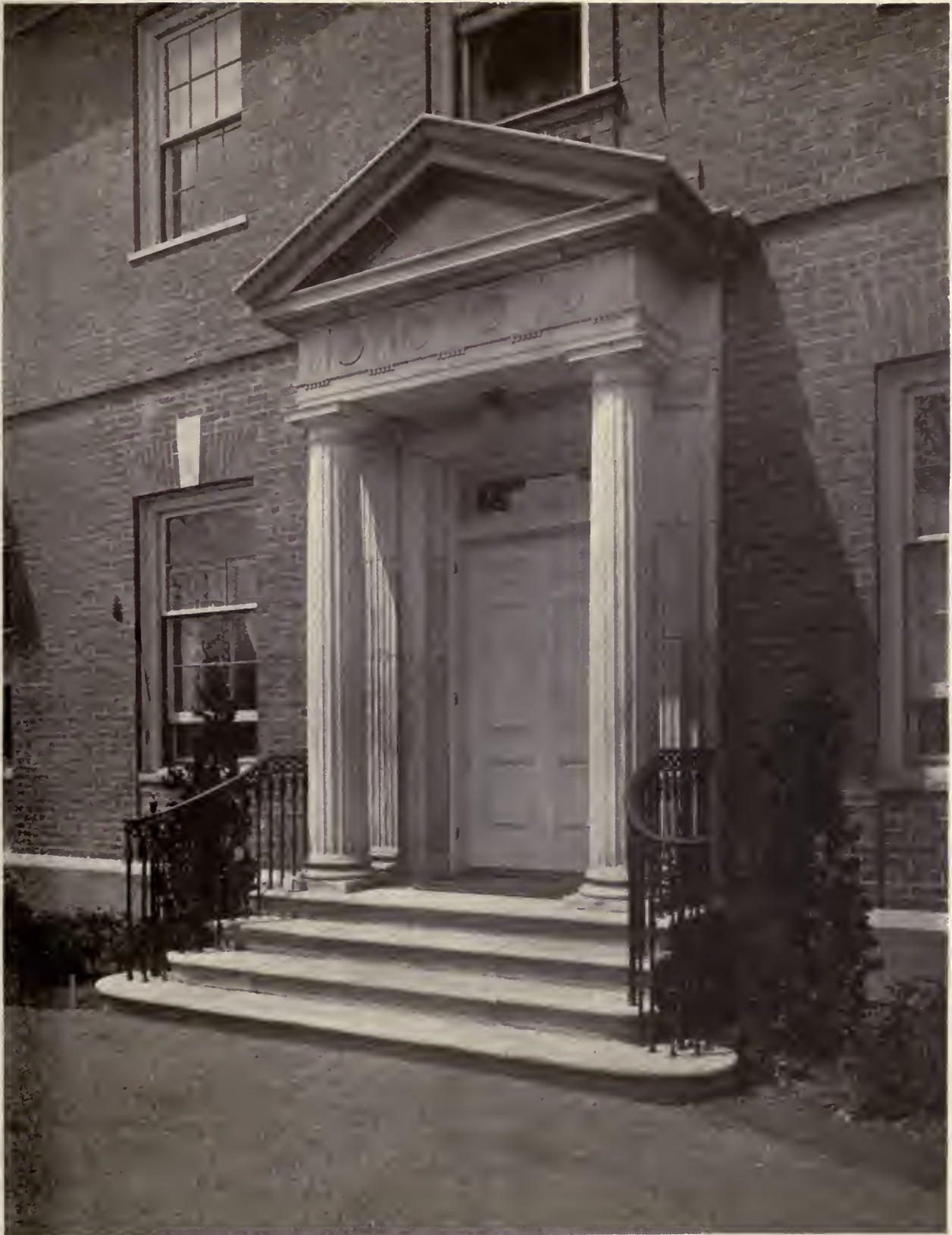
ENTRANCE DETAIL OF A HOUSE AT HARTFORD, CONN. GOODWIN, BULLARD & WOOLSEY, ARCHITECTS 1920 EXHIBITION OF THE ARCHITECTURAL LEAGUE OF NEW YORK
