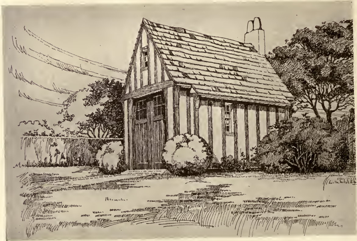
A ONE-CAR GARAGE AYMAR EMBURY II, ARCHITECT
