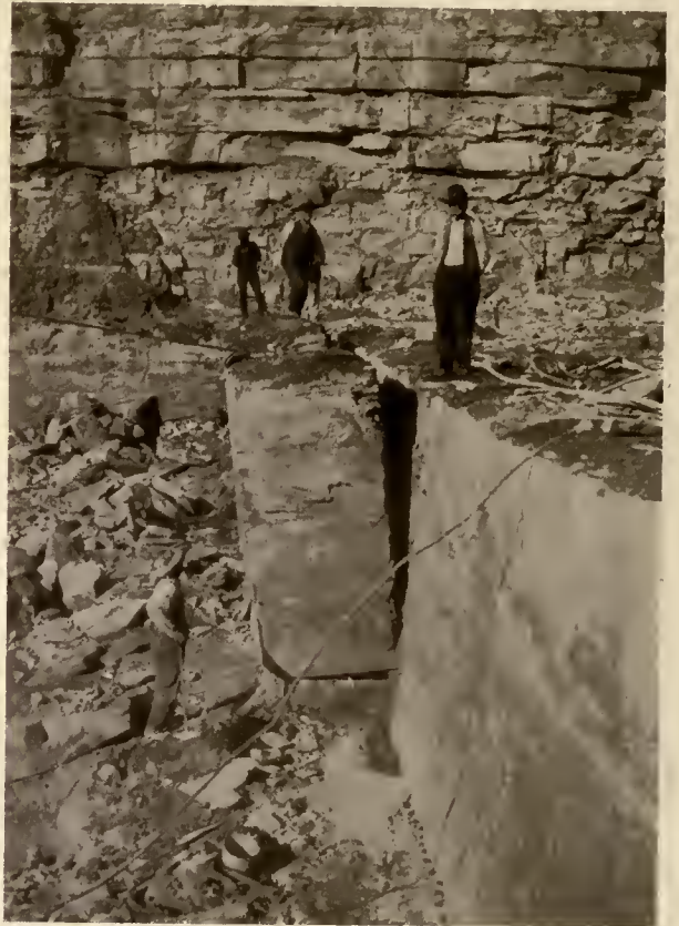
TURNING OVER "CUT" IN QUARRY AFTER BEING CUT OR CHANNELLED BY CHOPPING OR CHANNELING MACHINE
