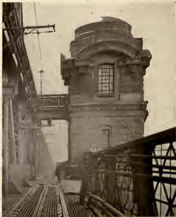
TOWER CONTAINING PASSENGER ELEVATOR AT BRIDGE PIER OF QUEENS APPROACH. ONE PLAN CONTEMPLATED THE ERECTION OF SIMILAR TOWERS AT THE BLACKWELLS ISLAND PIERS
