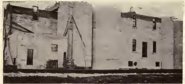
WALLS NEARING COMPLETION. NOTE HORIZONTAL LINES SHOWING PROGRESSIVE TIERS
