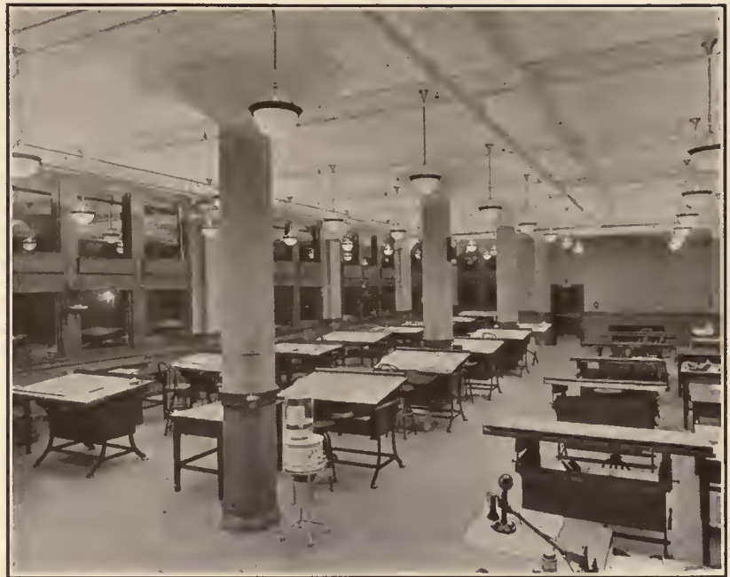
SEMI-INDIRECT ILLUMINATION IN DRAFTING ROOM OF AMERICAN CAN COMPANY, NEWARK, N. J.
