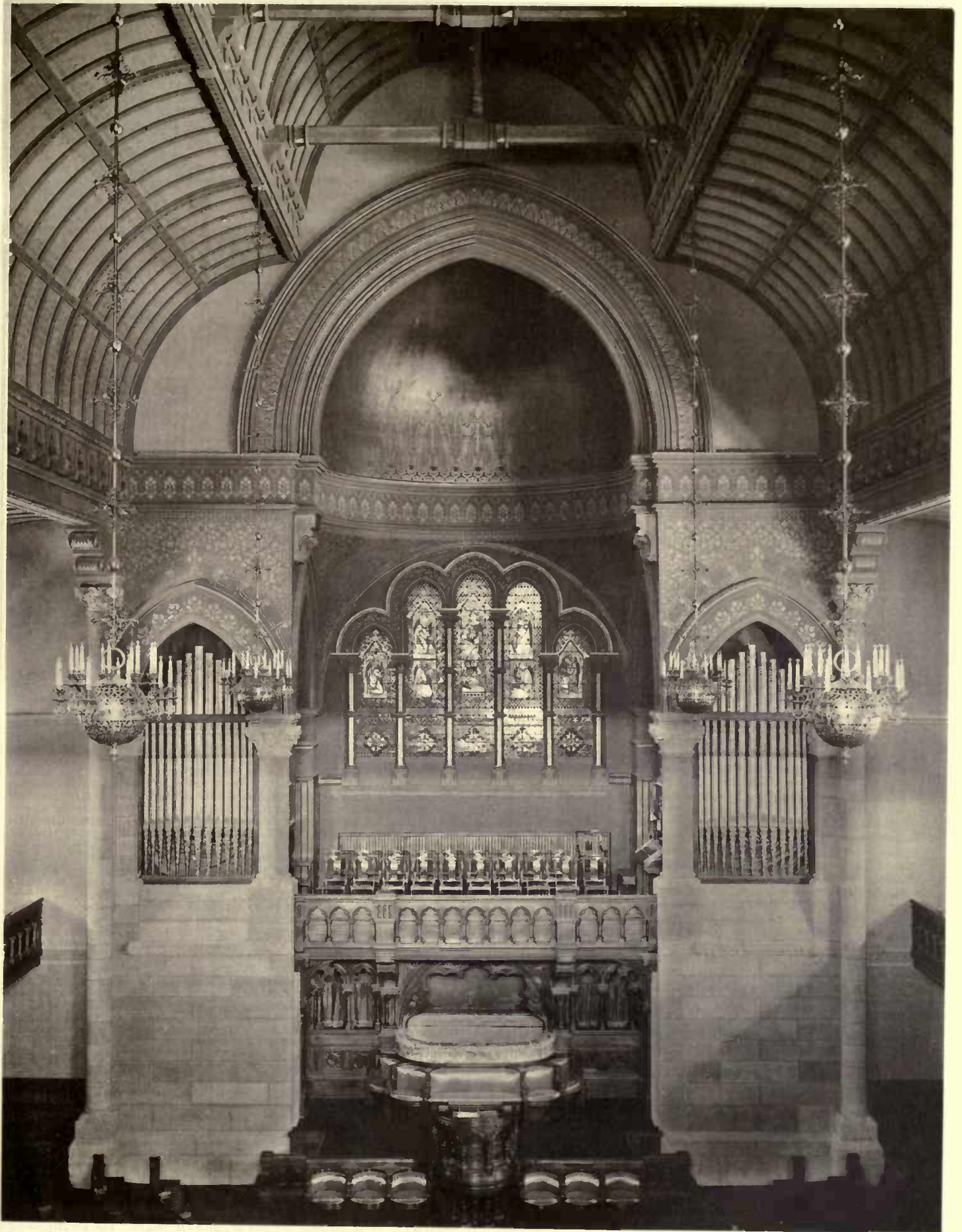
EMANUEL BAPTIST CHURCH, BROOKLYN, N. Y. FRANCIS H. KIMBALL, Architect.
