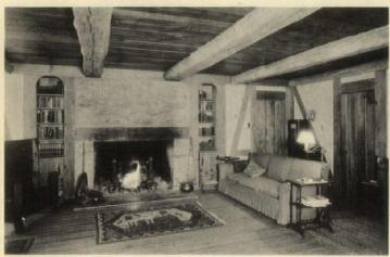
The walls of the livingroom show the timber construction, with a textured plaster between. Some old beams from a barn were
