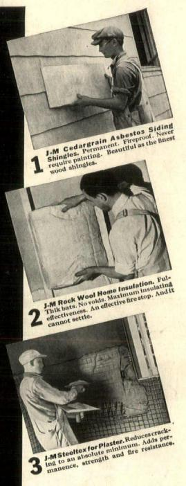
And what do we mean by a "triple-insulated" wall?
