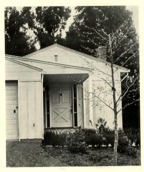
Exterior walls are of frame construction covered with 24-inch shingles painted, and brick veneer across the chimney end. Cubage, 28,000 feet; cost, including architect's fee, \$7400
