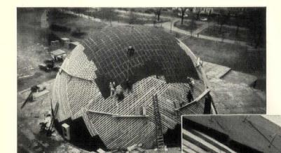
★ Covering the wooden framework of the Hayden Planetarium with J-M Rock Wool...unique in its ability to absorb sound and to insulate, as well. After the concrete shell was formed over the Rock Wool, this wooden lattice was removed and an interior dome of J-M Sanacoustic Panels of perforated stainless steel was suspended below the Rock Wool. These materials were also used on the side walls under the dome. Trowbridge and Livingston, architects.
