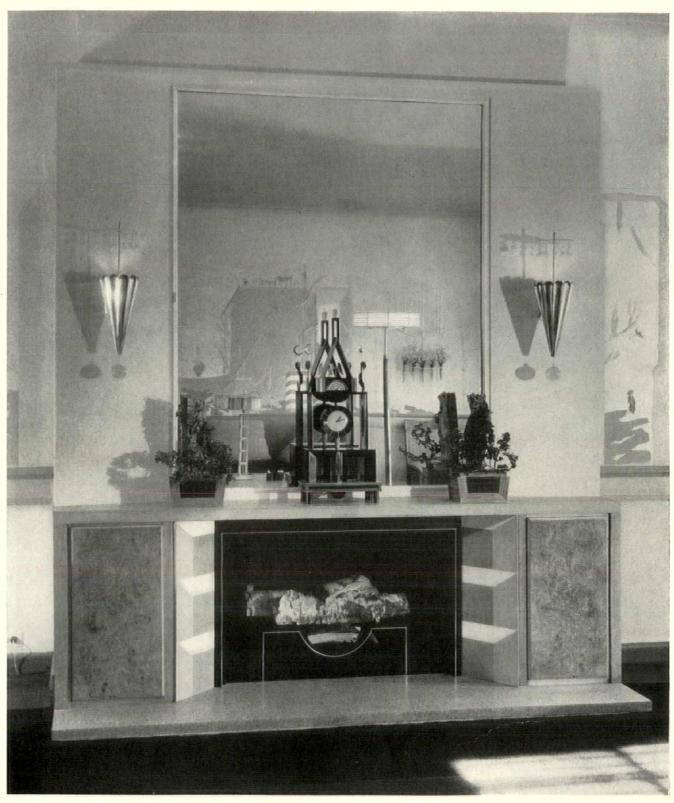
Chimney breast in the south living-room. The frame and jambs enclosing the hearth opening are of a marble composition, somewhat resembling terrazzo, in two shades of cerulean blue. To the right and left of the jambs are panels of olive wood behind which firewood is stored. The
