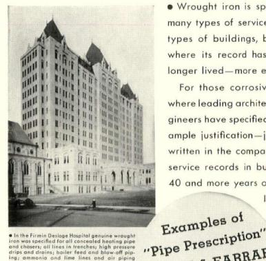
In the Firmin Desloge Hospital genuine wrought iron was specified for all concealed heating pipe and chasers; all lines in trenches; high pressure drips and drains; boiler feed and blow-off piping: ammonia and lime lines and air pip
