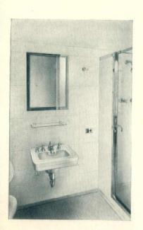
(Left) A Private Toilet and Bath—Crane Norwich vitreous china lavatories with liquid soap famets, ice water faucets, Securo leveraction wastes and Metro slow-closing supply valves. Crane shower fixtures. Crane Purus Jr. closets with Alpha flush valves.
