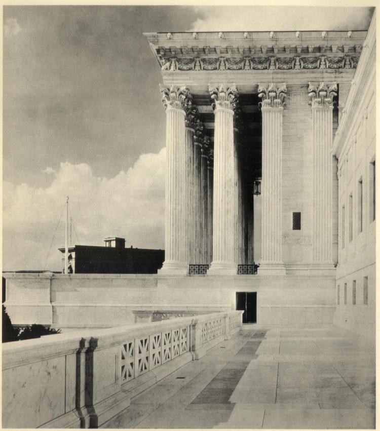
A detail of the south side of the west portico from the terrace. Incidentally, the marble paving of this terrace and the others is laid with an open joint of one-quarter inch between the slabs, to provide for expansion and contraction
