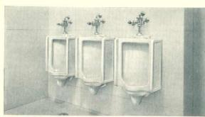
Men's Public Toilet No. 1—Crane Rio vitreous china wall urinals with foot-operated Alpha flush valves, Expedio wall closets with Alpha flush valves.
