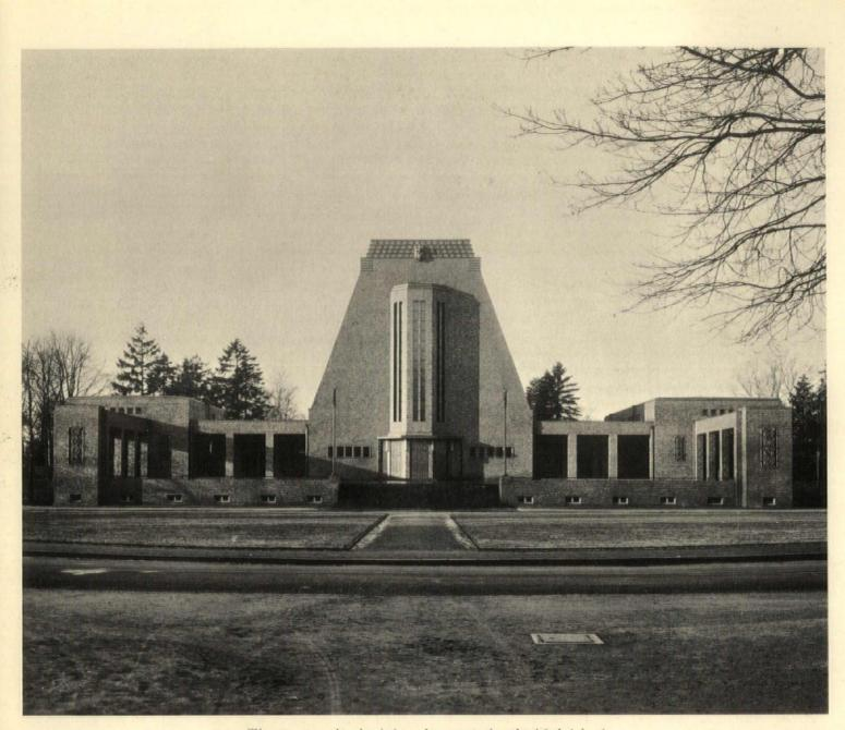
The structure is of reinforced concrete faced with brick of a blue-red color. All of the ornamentation—which is very much restricted—is in brick. There is a broad terrace across the front with the entrances through the loggia
