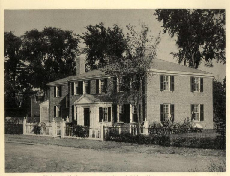
The house is of brick veneer on a wooden frame, the brick used being a common waterstruck New England brick laid with a wiped joint of light gray mortar. The trim is wood painted white, with the exception of the blinds and front door, which are dark green. A sea green Vermont slate is used for the roof
