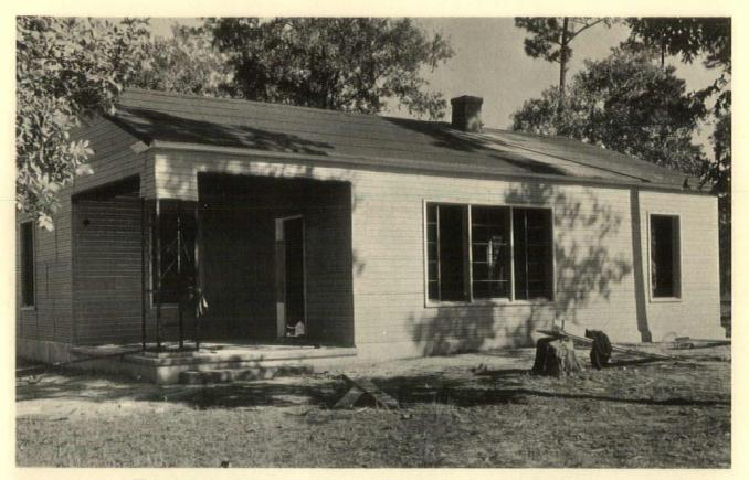
The exterior is plaster over a large-mesh fabric backed by insulation, which lat-ter is also carried under the roof of cement tiles. The cost of the house was \$2,750
