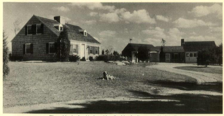
The roof is of cedar shingles, with walls of hand-split cypress shingles, all left to weather. Trim is white, with dark green shutters
