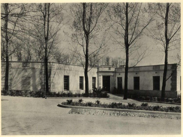
The walls are of stucco in a light buff with darker buff trim. This trim, also of stucco, is in a smooth finish, while the general field of the wall surfaces has a slight sand-floated texture. Window frames and staff beads are gray-blue, sash buff. The front door is dark green, with dark gray-blue frame and door trim
