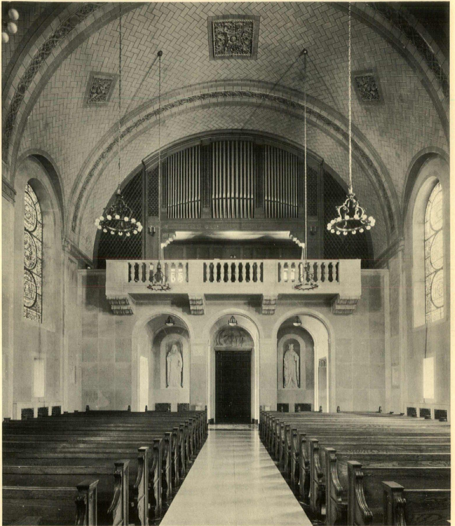
Walls are faced inside with Briar Hill stone, the arrises in Botticino marble, and the vault of acoustic tile. Gold is used sparingly on the ribs
