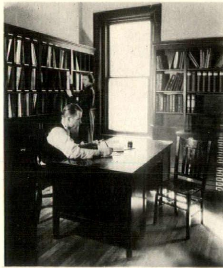
A corner of the library The drafting-room is shown below
