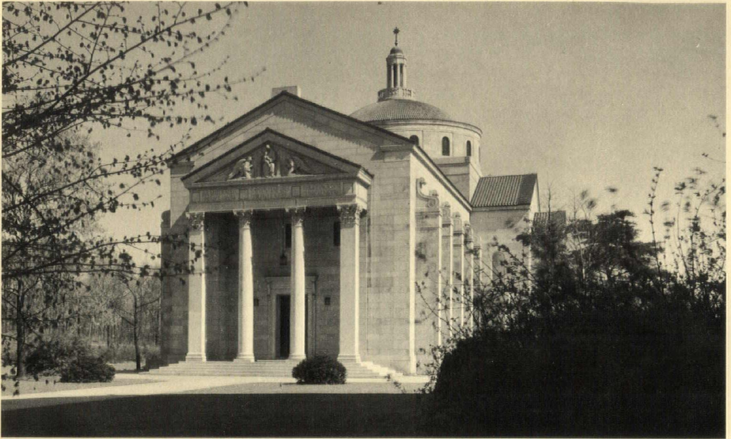
Kentucky limestone is used for the exterior walls, the roofs being of a Mission type of tile
