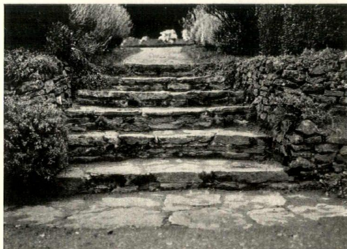
Below at right: In England—the stonework laid up with soil pockets
