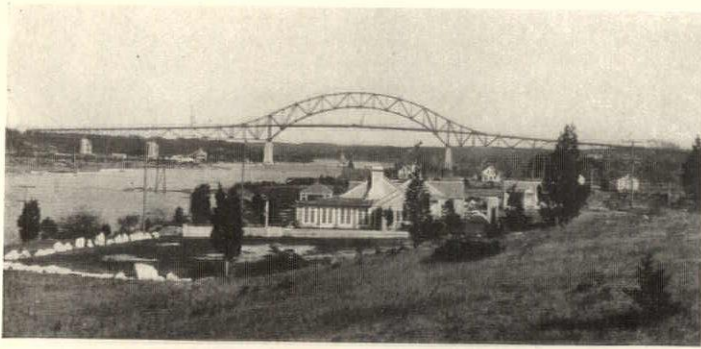
Bourne Bridge across Cape Cod Canal, at Bourne, Mass. Winner of Class A prize, 1934, A. I. S. C. Fay, Spofford & Thorndike, engineers
