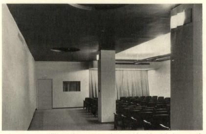
The conference room has a wide side aisle between the piers and the wall. On the latter objects are hung for demonstration and these are evenly lighted by the luminaires at the tops of the piers. Control lenses, set in a saw-tooth plan, direct the light from ordinary incandescent lamps upon the wall, without back glare—a form of lighting well adapted to corridor use or for lighting exhibition walls or mural paintings
