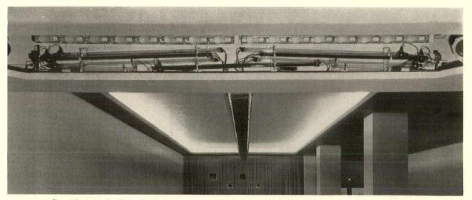
Detail of the built-in light source above and in front of the platform, in the same conference room, showing the mercury vapor and neon tubes for the production of a light closely approximating daylight. There are also three mercury vapor ultra-violet lamps and the upper series of incandescent lamps, making possible many special effects for demonstration purposes
