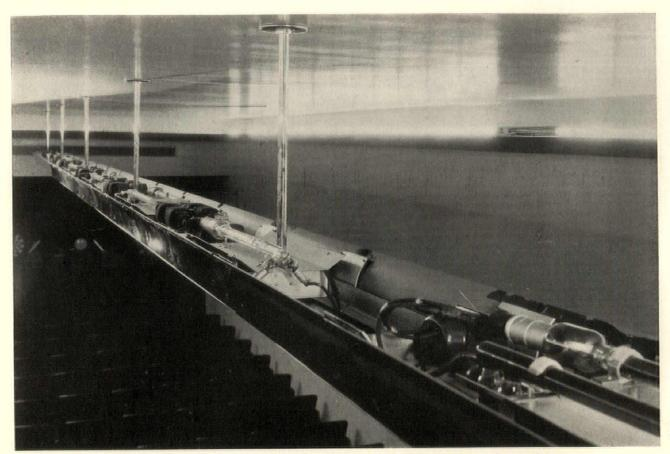
Looking down into the trough fixture, showing the mercury vapor and neon lamps with their auxiliary apparatus
