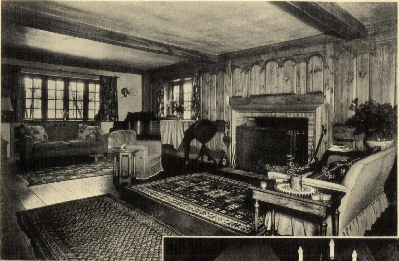
In the living-room one whole long side is panelled in pine. The floor is of oak in random-width boards, screwed down and plugged. Ceiling beams are of oak with a molded edge
