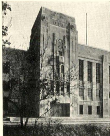
● 124th Field Artillery Armory, Chicago. Perkins, Chatten & Hammond, Architects—C. Herrick Hammond, State Architect. Byers Genuine Wrought Iron Pipe specified for hot and cold water lines, branch wastes and vents and heating return lines.
