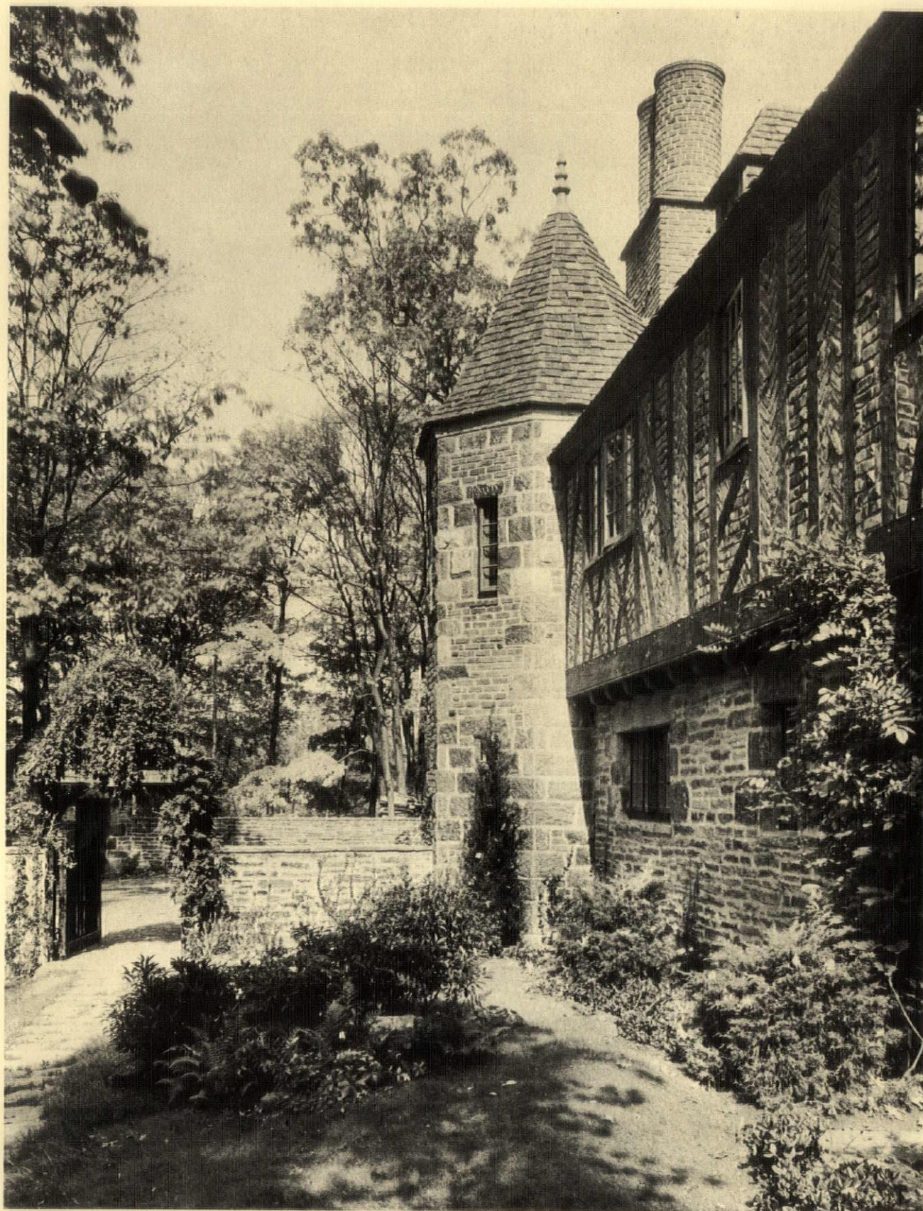
Another view of the west front, looking toward the enclosed court. The half-timber work, with its brick nogging, is of structural timbers doweled and pinned together
