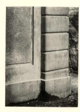
On the left, a structural concrete wall in which there is no provision for color other than that of the natural cement
