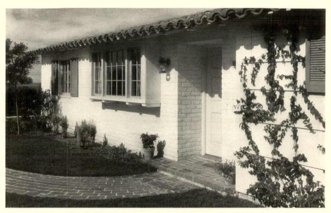
Detail of the front entrance, showing the junction of the brick wall and the sheathed wall. Below, one side of the living-room, the seventeen-foot width of which is not encroached upon by a chimney breast
