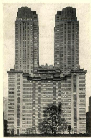
A substantial tonnage of Bethlehem Light Sections was used in the framework of the Century Apartments, N.Y. C.—Chanin Construction Co., Inc., General Contractors; I.S. Chanin, Architect; Alexander D. Crosett, Engineer. loads, such as apartment houses, school buildings, hospitals, hotels, and similar structures.
