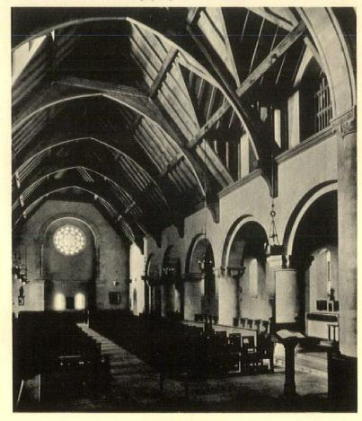
In the north aisle, looking toward the baptistry. Walls are sand-finished plaster adjoining the limestone structure of piers and arches. The floor is of flagstone
