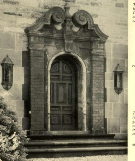
The architect has used a local stone secured in part from old fences in the vicinity. Limestone is used for the trim, and there is a tile roof of reds and browns. This is the east front with its loggia and broad steps leading down to a terrace
