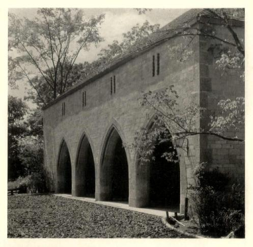
The open shed, with the stable for the farm horses in the foreground. It will be noticed that in the wall structure a variety of texture and jointing has been obtained by the use of block courses of four heights—4, 5, 6, and 8 in. The quoins and trim are of cast stone
